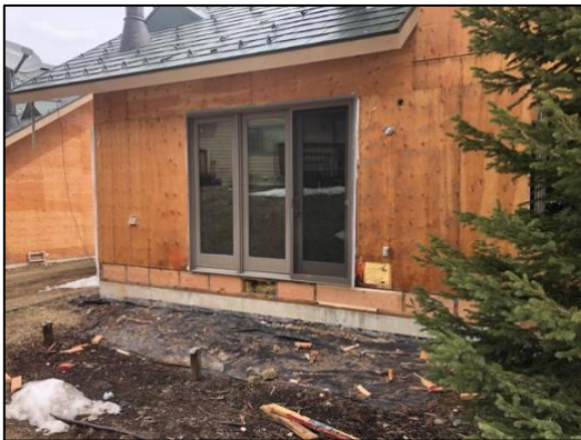
Bldg E4 Unit #28 New Ledger Blocking
