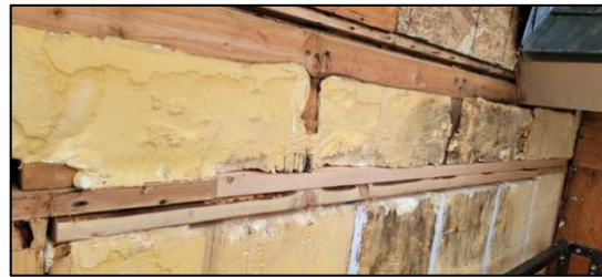
Bldg E4 Unit #28 Entry Exterior Repaired
