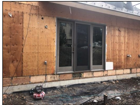
Bldg E4 Unit #29 New Ledger Blocking
