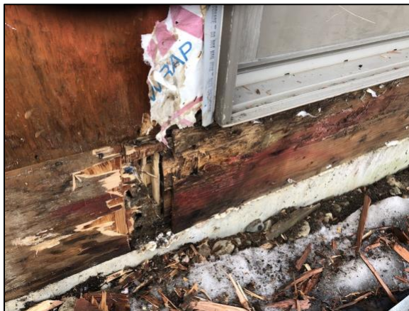
Bldg E3 Unit #24 Deck Location
