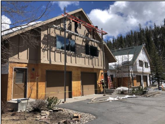
Bldg E3 South Side – Looking East
