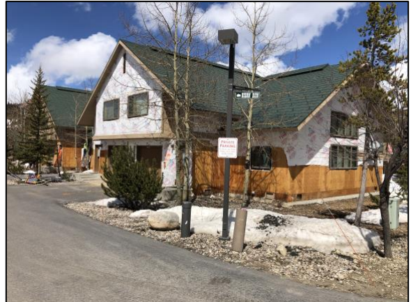
Bldg E3 South Side – Looking West
