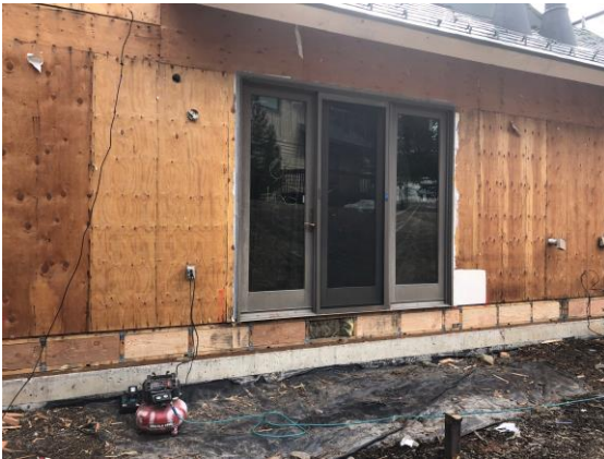
Building E4 Unit #29 Deck Blocking in Place
