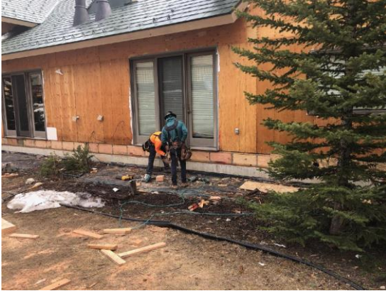
Building E4 Unit #30 Deck Blocking in Place
