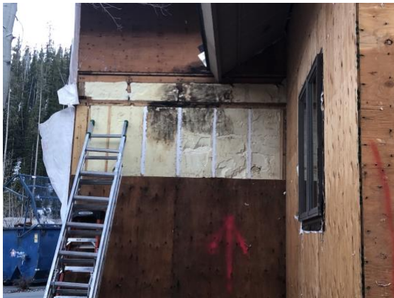
Bldg E4 Unit #28 with Vert Studs Treated
