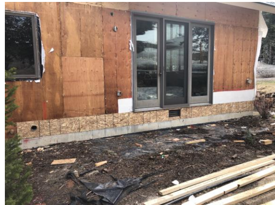
Building E4 - Unit #31 Sheathing over blocking
