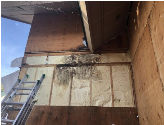
Bldg E4 Unit #28 Exterior Wall at Entry-3
