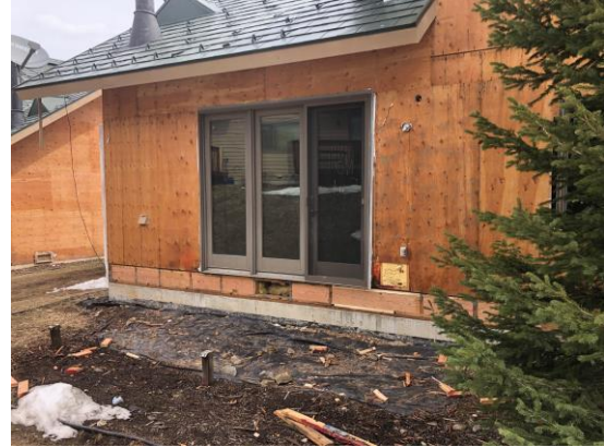
Building E4 Unit #28 Deck Blocking in Place
