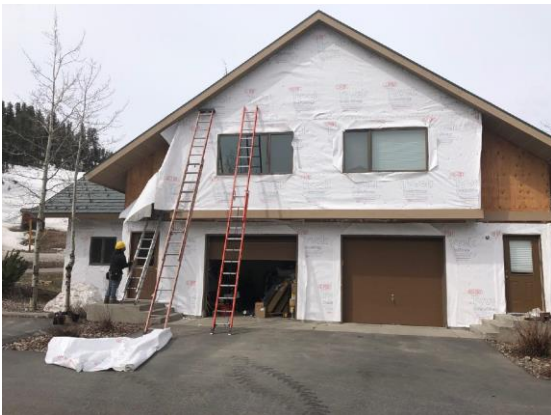
Building E4 - Units 31,30 Building Wrap
