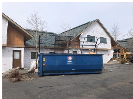
Building E4 - Units 29, 28 Building Wrap North Side
