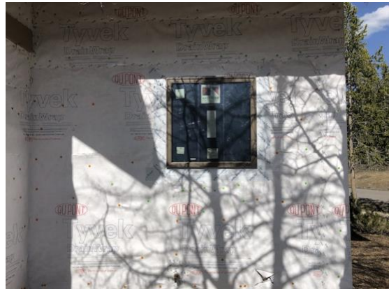
Bldg E3 Unit #27 Kitchen Wdw in Place
