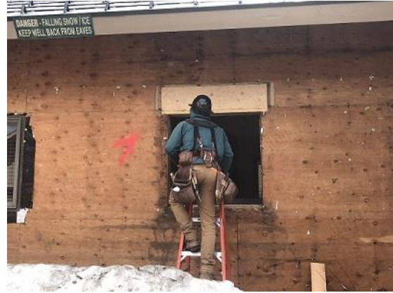
Bldg E1 Unit #10 New Kitchen Window Header
