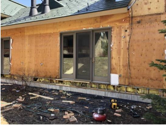
Bldg E2 Unit #22 Blocking in Progress
