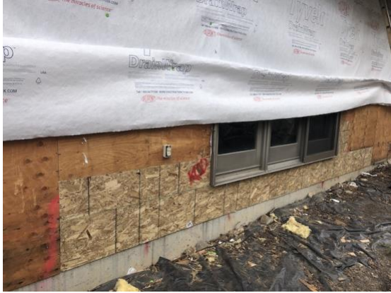
Bldg EW1 Unit #10 Repairs Complete
