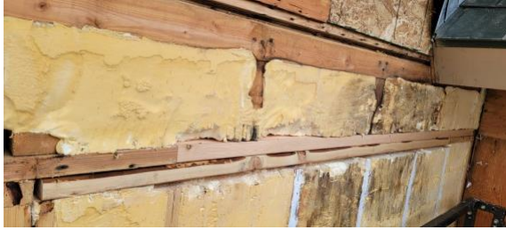
Unit #28 Top Plate at Entry Repair
