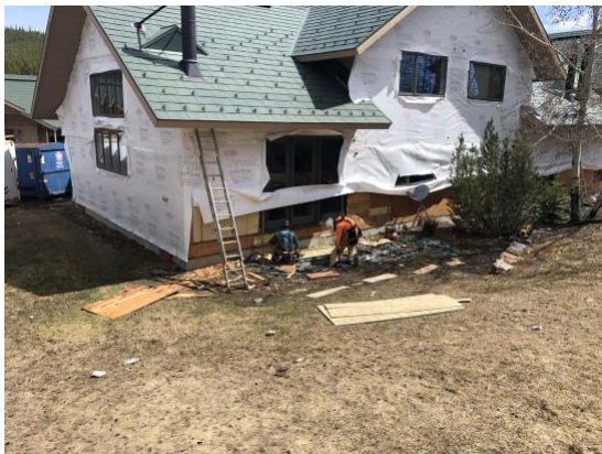
Bldg E1 Unit #11 Blocking Progress
