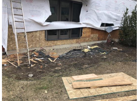
Bldg EW1 Unit #11 Repairs Complete
