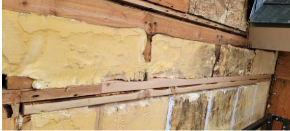
Unit #28 Top Plate at Entry Repair
