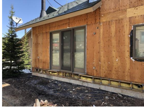
Bldg E2 Unit #20 Blocking in Progress
