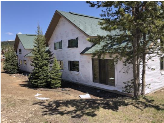
Bldg E4 South & East Sides Wrap in Progress
