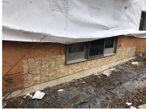
Bldg EW1 Unit #09 Repairs Complete
