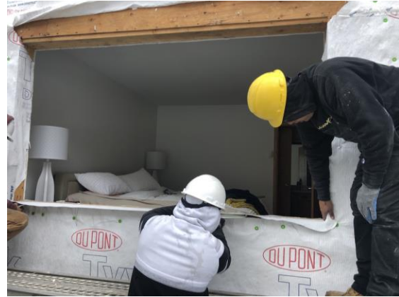
Bldg E1 Unit #10 Window Installation Progress
