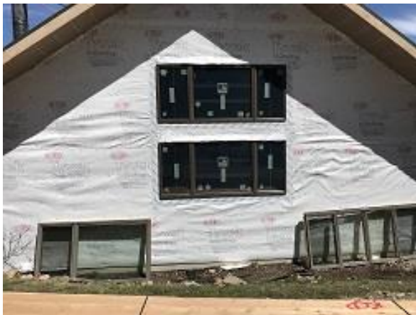
Bldg E4 Unit #31 Upper & Lower Side Windows
