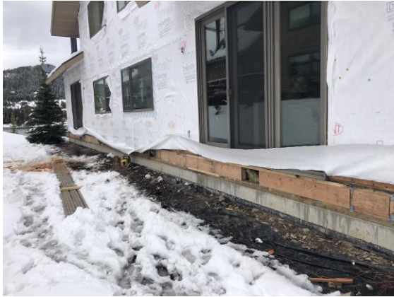
Bldg E2 Units #20 & #21 Future Deck Area Blocking
