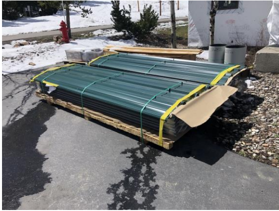
Delivery of Soffit Material
