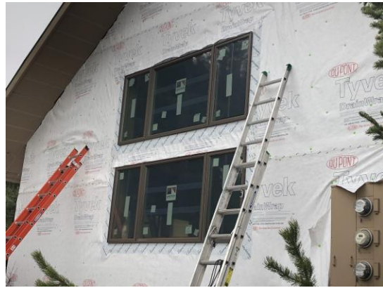
Bldg E1 Unit #8 Lower & Upper Window
