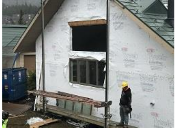
Bldg E1 Unit #11 Upper Window in Progress
