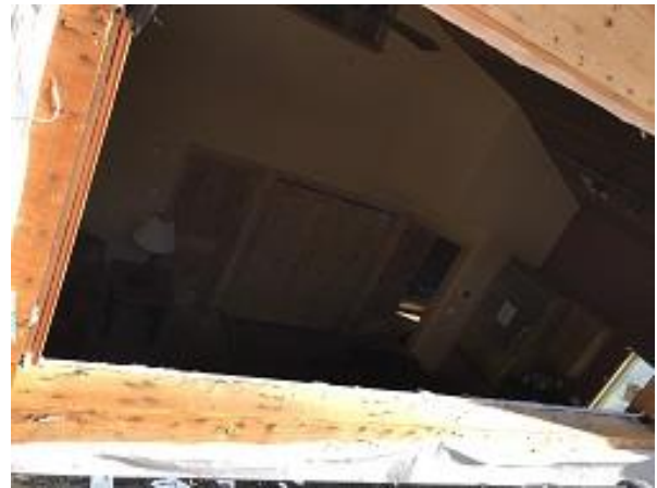
Bldg E4 Unit #31 Upper Window Sill
