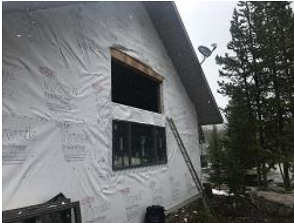
Bldg E3 Unit #27 South Upper Window In Progress
