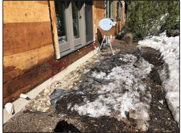
Bldg E1 Unit #11 Previous Patio Location
