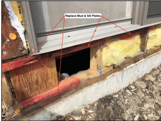
Bldg E3 Unit #24 Replace Wood Rot @ Mud & Sill Plates
