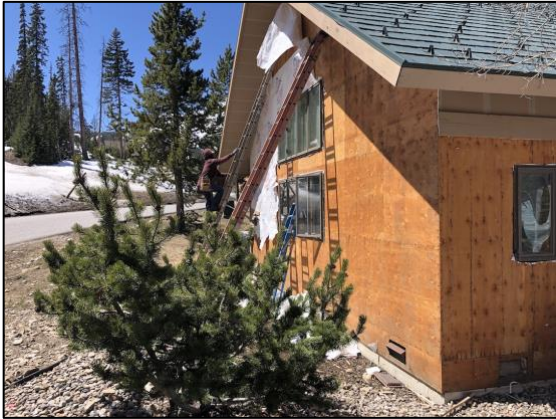
Bldg E4 Unit #31 East Side Siding Removal
