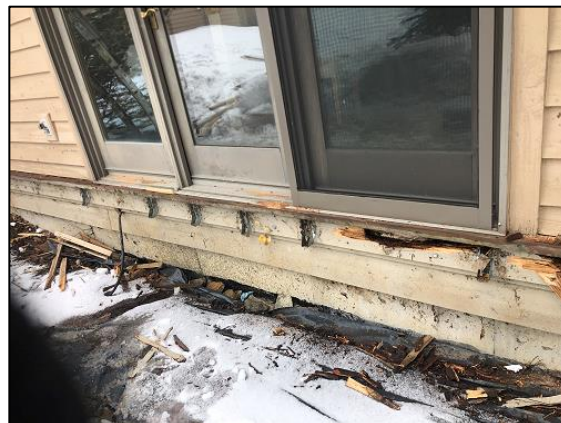
Bldg E3 Unit #8 Existing Deck Location
