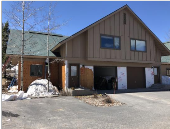
Bldg E4 Unit #31 North Side Siding Removal
