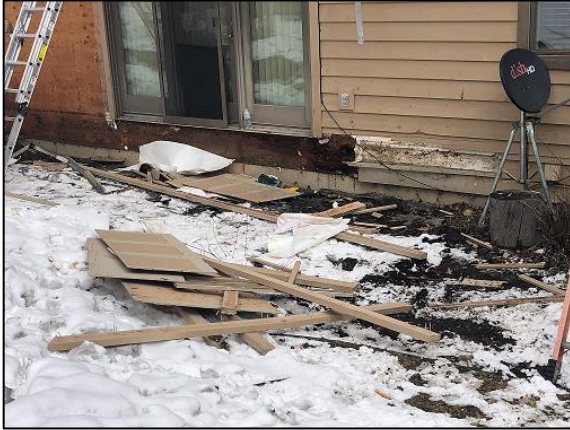
Bldg E3 Unit #9 Existing Deck Location
