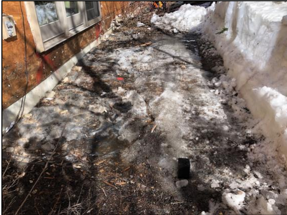
Bldg E1 Unit #10 Previous Patio Location
