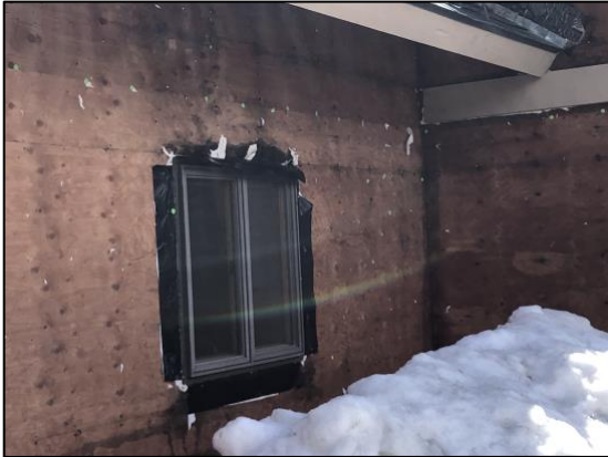
Bldg E1 Unit #10 Kitchen Window
