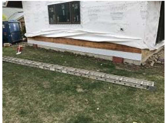
Building E1 Unit 11 Flashing Tape Installation
