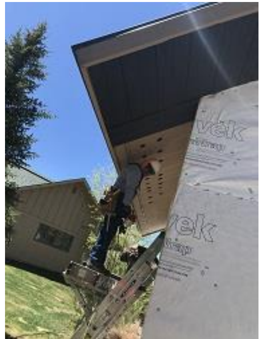
Building E1 Unit 8 Venting Drilled
