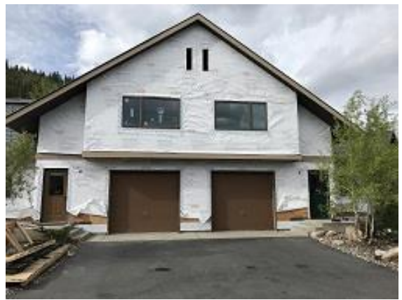
Building E1 Unit 10 & 11 Gable Vents
