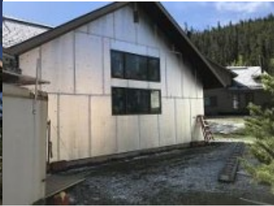
E1 Unit 8 Foam Board Installation Building E1 Unit 11 Foam Board Installation
