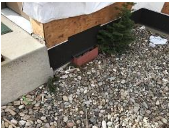
Building E1 Unit 9 Metal Flashing Installation
