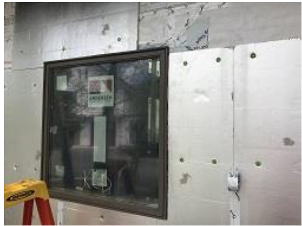
Building E3 Unit 24 Kitchen Window Flashing and Insulation Foam Board Installation
