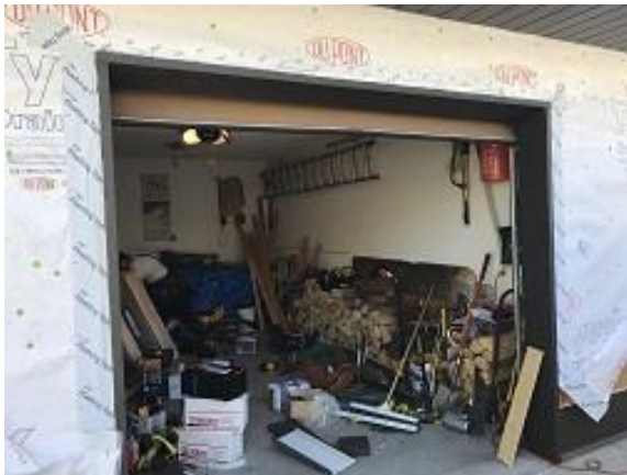
Building E3 Unit 24 Garage Door Trim Metal Installation
