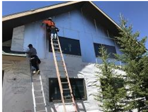
Building E3 Unit 27 & 26 Foam Board Installation
