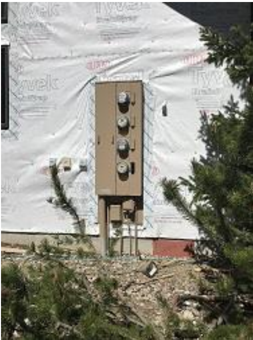
Building E1 Unit 8 Flashing Tape Applied
