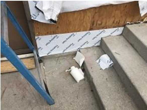
Building E3 Unit 27 Setup Flashing Tape
