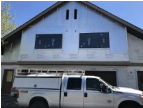
E3 Unit 24 Foam Board Installation Building E3 Unit 27 & 26 Foam Board Installation
