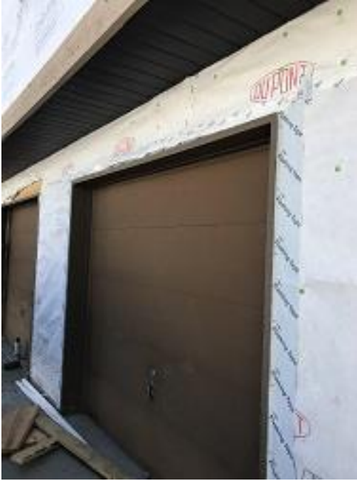
Building E3 Unit 25 Flashing Tape Applied
