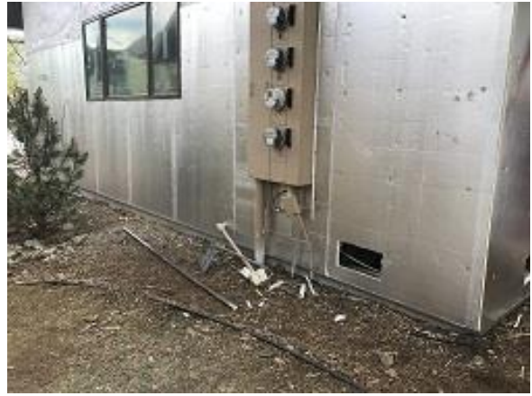
Building E3 Unit 24 Insulation Board Installation
