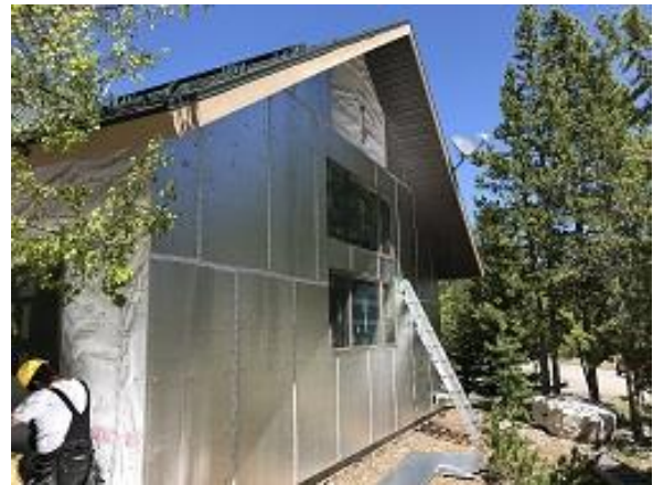
Building E3 Unit 27 Foam Board Installation
