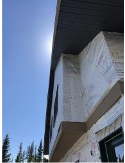
Building E1 Unit 11 & 12 Soffit Installed
