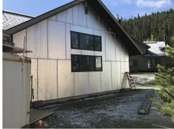
Building E1 Unit 11 Foam Board Installation
