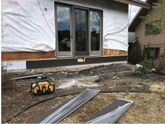
Building E3 Unit 24 Metal Flashing Installation
