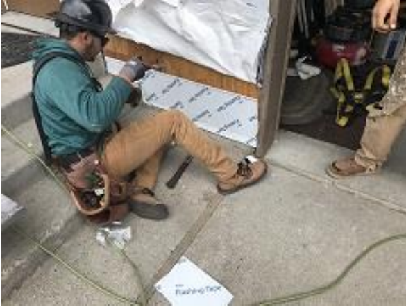
Building E3 Unit 24 Setup Flashing Tape
