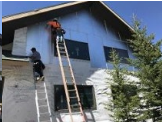
E3 Unit 24 Foam Board Installation Building E3 Unit 27 & 26 Foam Board Installation
