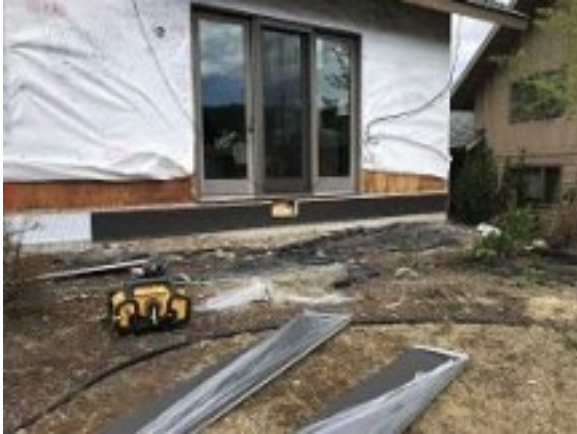
Building E3 Unit 24 Metal Flashing Installation Building E1 Unit 11 Diverter Flashing
