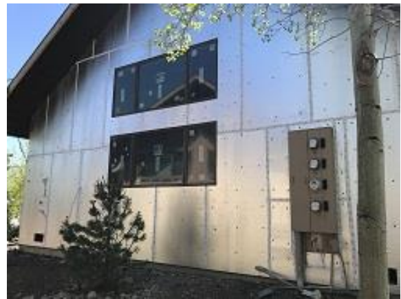
Building E3 Unit 24 Foam Board Installation
