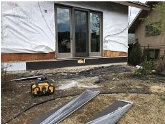
Building E3 Unit 24 Metal Flashing Installation
