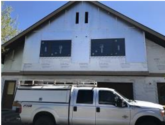
Building E3 Unit 24 Foam Board Installation
