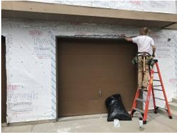
Building E2 Unit 20 Garage Flashing Tape Application
