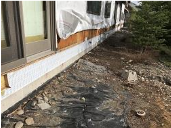
Building E3 Unit 27 Flashing Tape Installation
