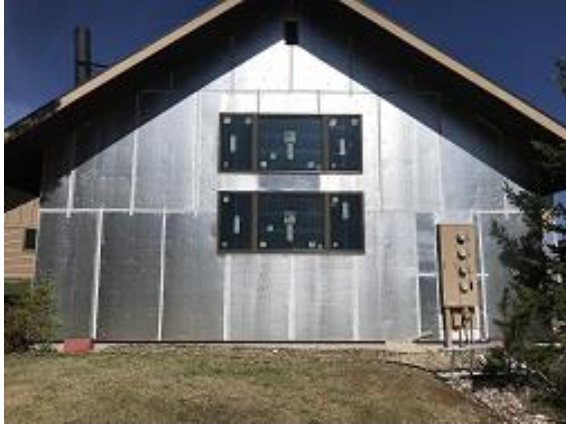
Building E1 Unit 8 Foam Board Installation
