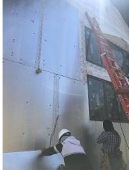
Building E3 Unit 24 Window Drip Flashing & Insulation Board Installation
