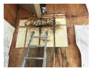
Building F1 Unit 17 Damaged Sheathing Removed For Engineer Inspection
