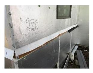
Building E3 Unit 24 Front Wainscote Top Metal Flashing Installation
