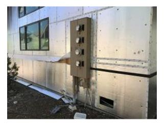
Building E3 Unit 24 Side Wainscote Top Metal Flashing Installation
