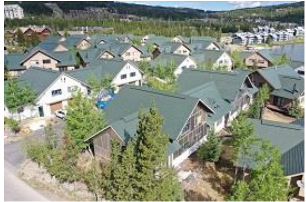
Bldg E3 North and East Sides
