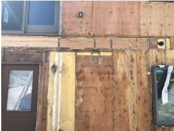
Building F1 Unit 16 Ledger Blocking
