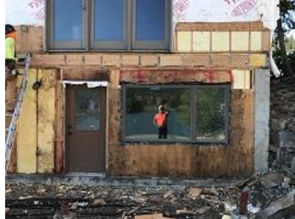
Building F1 Unit 17 Ledger Blocking
