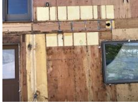
Building F1 Unit 16 Ledger Blocking
