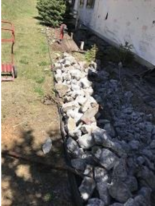
Building E4 Units 29 & 28 Deck Footing Demo
