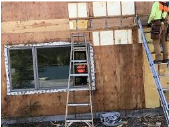
Building F1 Unit 17 Ledger Blocking
