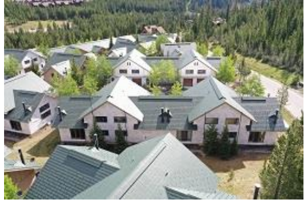
Bldg E4 South Side
