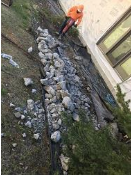
Building E4 Unit 30 Deck Footing Demo
