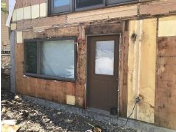
Building F1 Unit 16 Ledger Blocking
