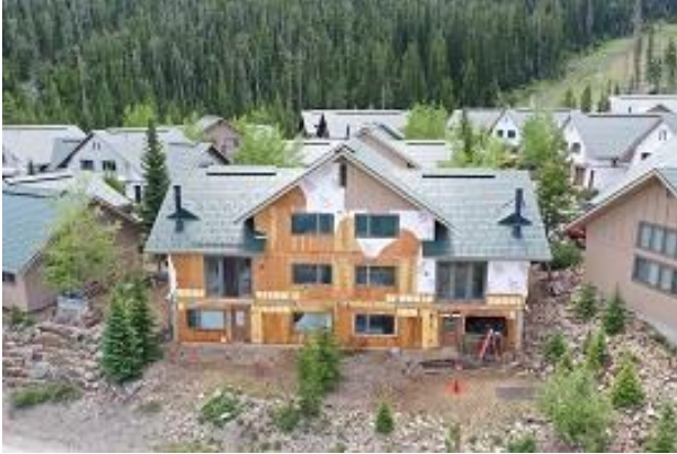
Bldg F1 West Side Sheathing Repair in Process
