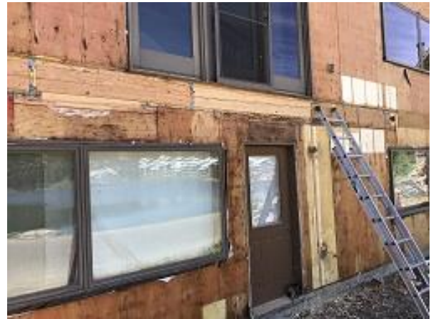
Building F1 Unit 16 Sheating Removal for Sheating Replacement
