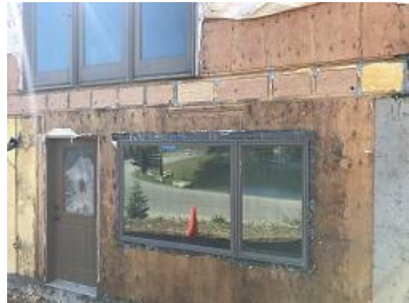
Building F1 Unit 17 Ledger Blocking
