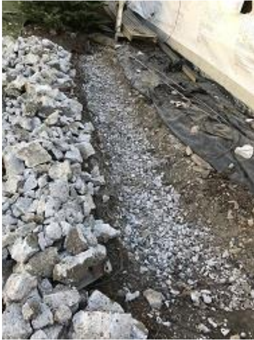
Building E4 Unit 28 Deck Foundation Removal
