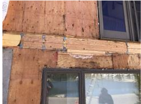
Building F1 Unit 16 Ledger Blocking
