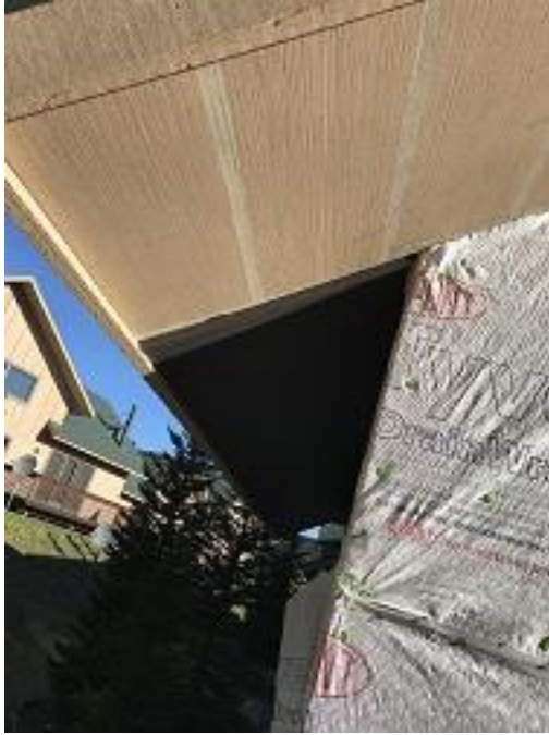
Bldg E4 Unit #31 Rear Soffit
