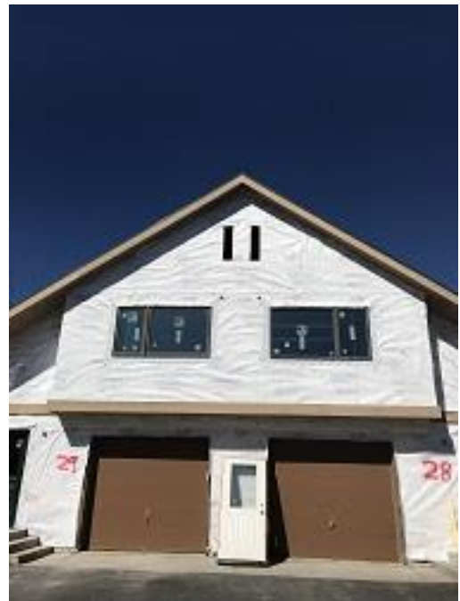
Bldg E4 Unit #28 & 29 Gable Vents
