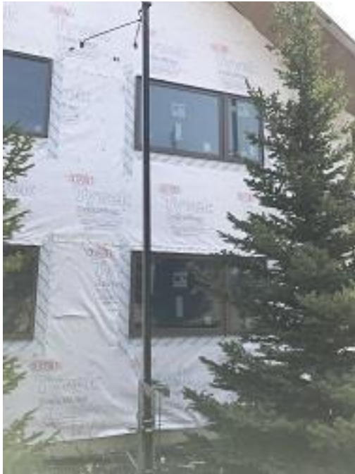
Bldg E4 Unit #29 Upper & Lower Windows
