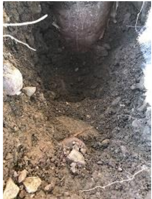
Bldg E5 Unit #44 Deck Pier Foundation
