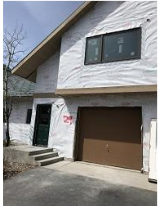
Bldg E4 Unit #29 Above Garage
