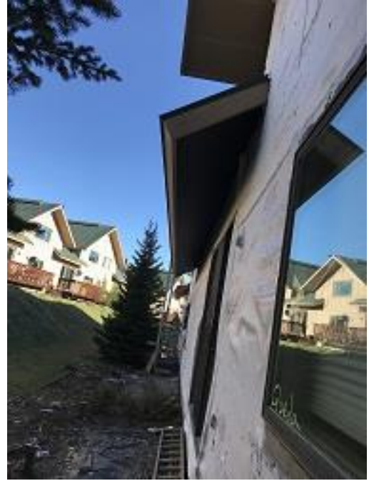
Bldg E4 Unit #30 & 29 Rear Soffit
