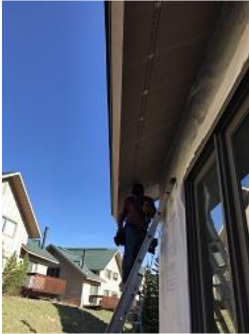
Bldg E3 Unit #28 Rear Cutouts Soffit Vents
