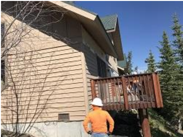
Building E7 Unit 49 Demo Continues
