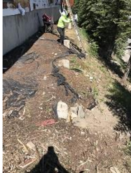
Building E7 Unit 49 Deck Pier Bracket Removed
