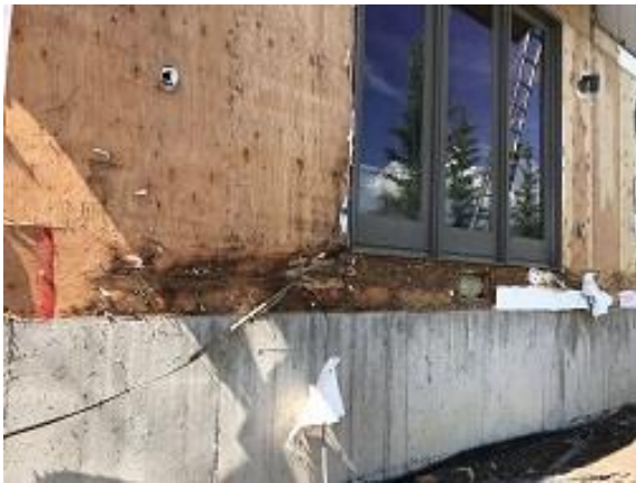
Building E7 Unit 49 Deck Blocking Area Defined
