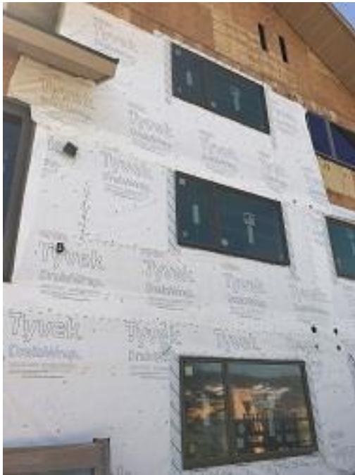
Building F1 Unit 16 & 17 Demo Continued
