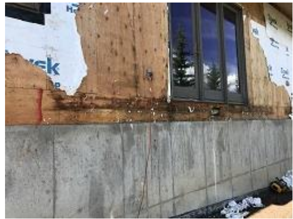
Building E7 Unit 50 Deck Pier Blocking Area Defined
