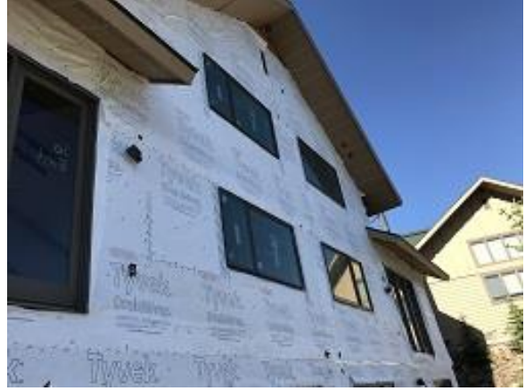
Building F1 Unit 17 Rear Upper Window Installed
