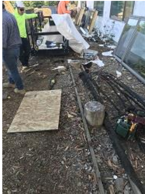
Building F1 Unit 17 Deck Brackets Removed
