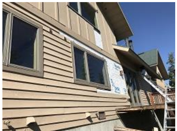
Building E7 Unit 49 & 50 Demo
