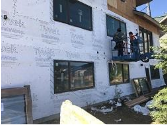
Building F1 Unit 16 & 17 Window Installation
