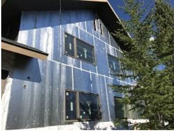
Building E3 Unit 24 & 25 New Attic Vents Cut In
