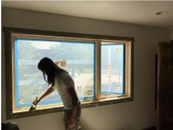
Building E3 Unit 27 Lower Back Window Urethane Application
