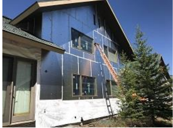
Building E3 Unit 26 & 27 Cut In Vents
