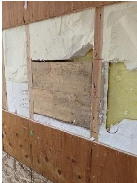
Building F1 Unit 16 Upper Deck Railing Blocking
