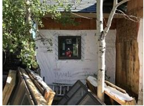
Building F1 Unit 17 Kitchen Window Installed
