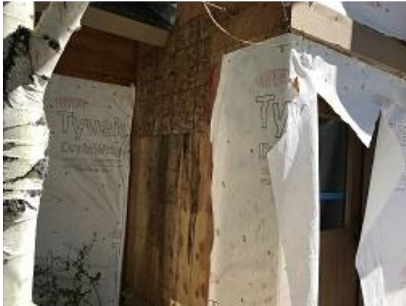
Building F1 Unit 17 Sheathing Replacement
