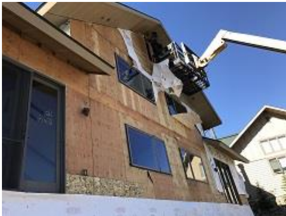
Building F1 Unit 16 & 17 Demo Continued
