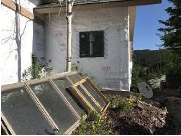
Building F1 Unit 16 Kitchen Window Installed
