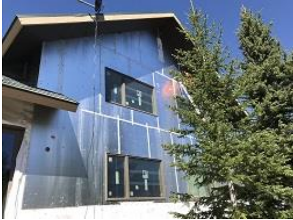
Building E3 Unit 24 & 25 Cut In Vents
