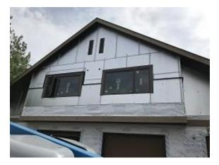
Building E3 Unit 24 & 25 Front Upper Window Flashing and Gable Vent Installation
