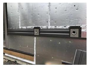
Building E3 Unit 26 & 27 Lap Siding and Vent Blocking
