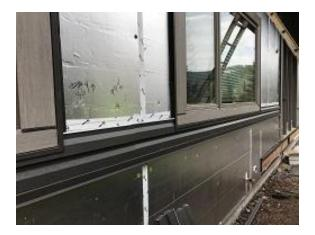
Building E3 Unit 27 & 26 Lap Siding Installed
