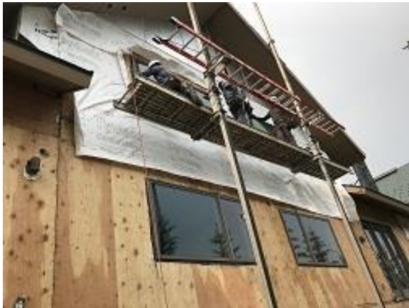
Building E7 Unit 49 & 50 Back Bedroom Window Replacement
