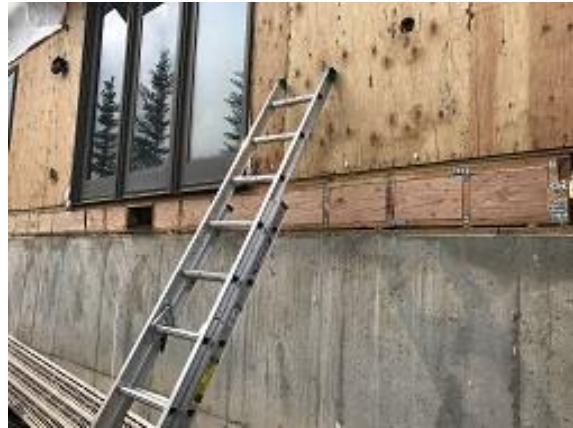
Building E7 Unit 50 Deck Ledger Blocking
