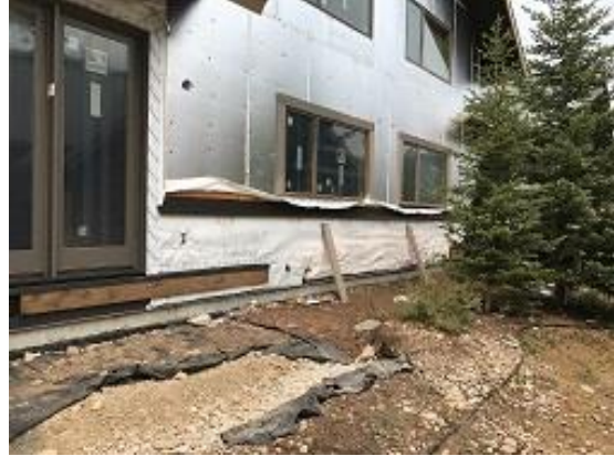
Building E3 Unit 26 & 27 Wainscot Flashing Installation
