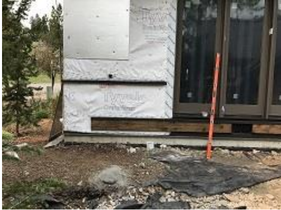
Building E3 Unit 27 Wainscot Flashing Installation
