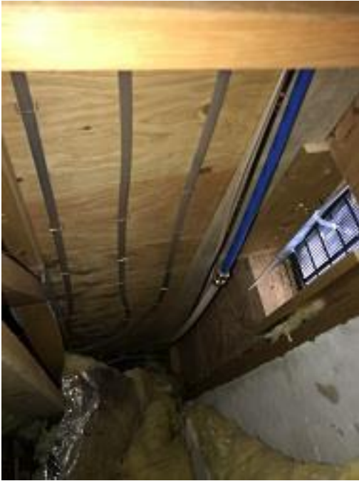
Building E3 Unit 27 Patio Door Subfloor and Repaired Radiant Heat Tubing
