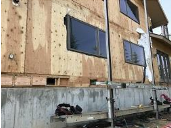
Building E7 Units 49 Deck Blocking Installation
