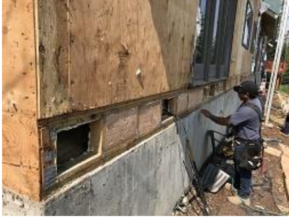
Building E7 Units 49 Deck Blocking Installation
