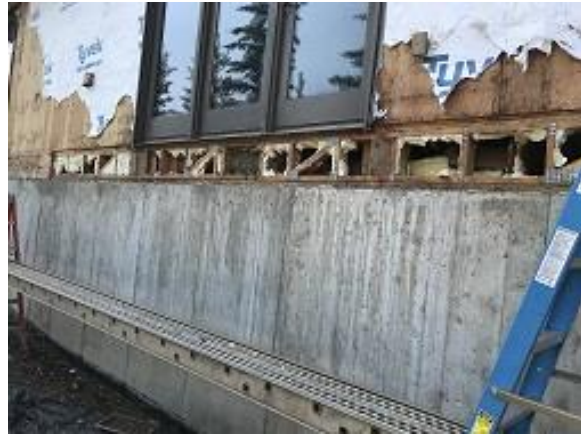
Building E7 Units 51 Deck Blocking Installation
