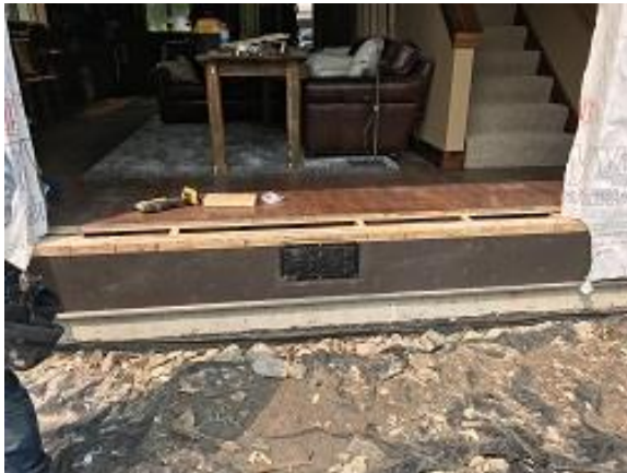
Building E3 Unit 27 Patio Door Threshold Prior to Installation
