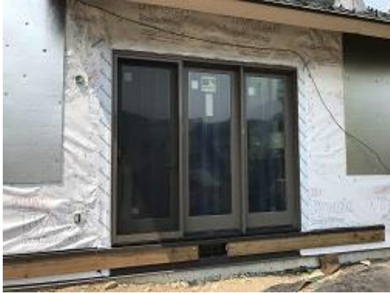
Building E3 Unit 24 Patio Door Installed
