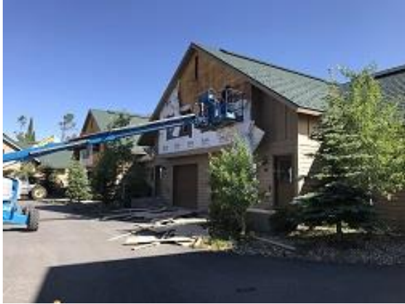
Building E7 Unit 49 & 50 Front Upper Bedroom Demo
