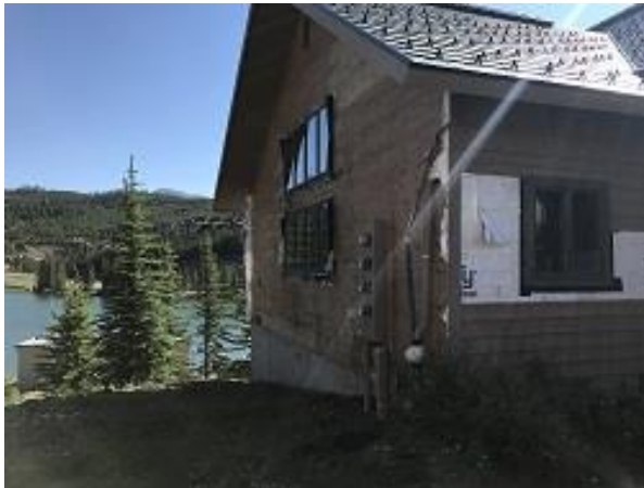
Building E7 Unit 52 Side Lower & Upper Window Demo
