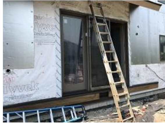
Building E3 Unit 25 Patio Door Installed
