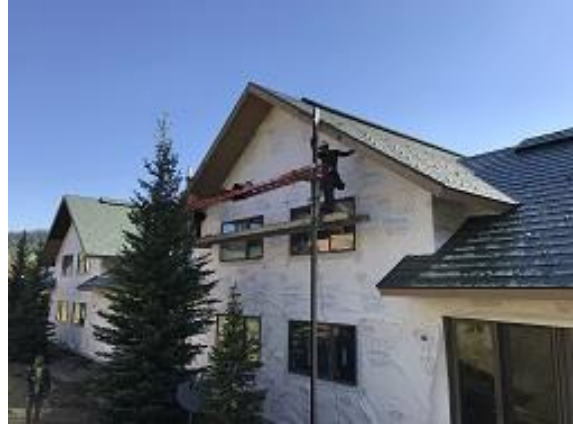
Building E4 Unit 30 & 31 Foam Installation
