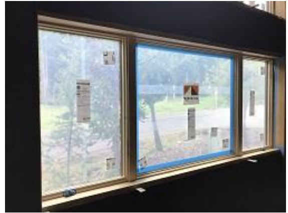
Building E3 Unit 27 Lower Livingroom Window Finish Applied
