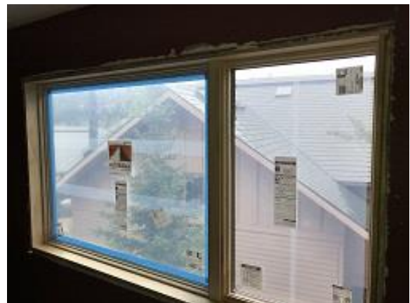
Building E3 Unit 27 Upper Back Bedroom Window Finish Applied
