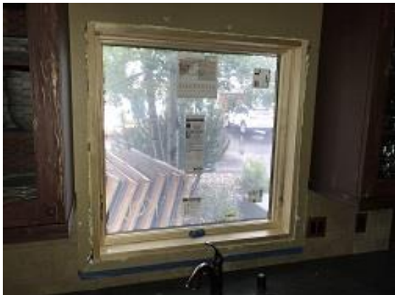
Building E3 Unit 27 Kitchen Window Finish Applied
