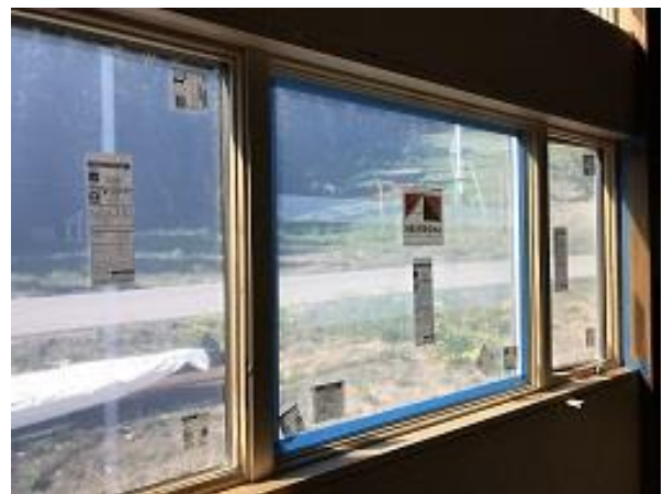
Building E4 Unit 31 Living Room
