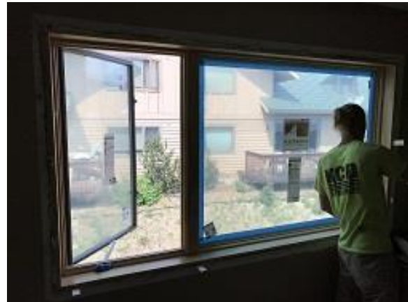
Building E2 Unit 21 Upstairs Back Bedroom Window Urethane Applied
