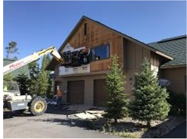
Building E7 Unit 51 & 52 Front Upper Bedroom Demo
