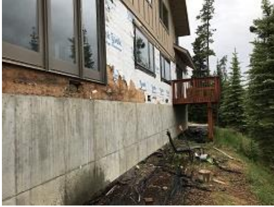
Building E7, Units 51 & 52 demo
