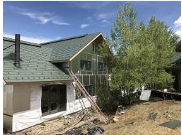
Building E1 Unit 10 & 11 Foam Board Installation
