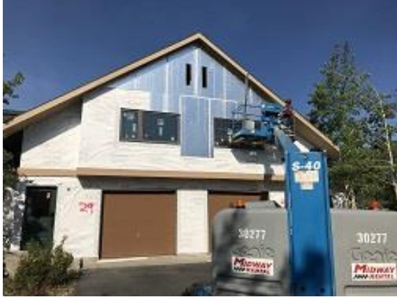
Building E4 Unit 28 & 29 Foam Installation
