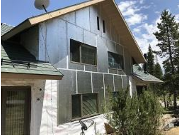
Building E1 Unit 8 & 9 Foam Board Installation
