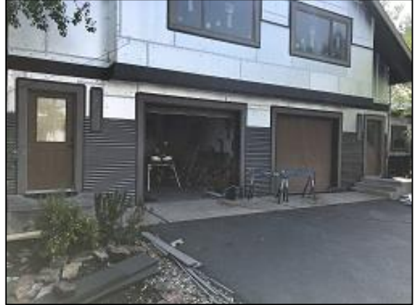
Building E3 Units #24 & #25 Front Corrugated Installation
