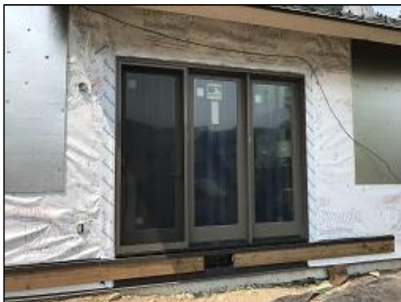
Building E3 Unit #24 Patio Door Installed
