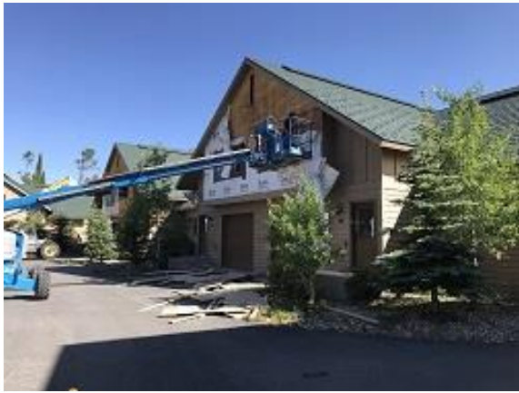
Building E7 Unit #49 & #50 Front Upper Bedroom Demo
