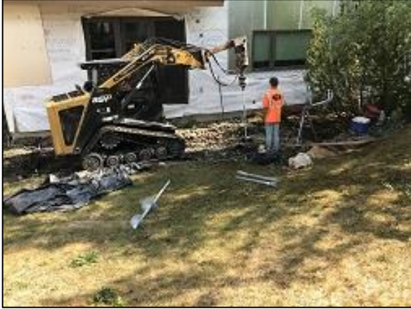
Building E3 Unit #27 Begin Deck Helical Piers Installation
