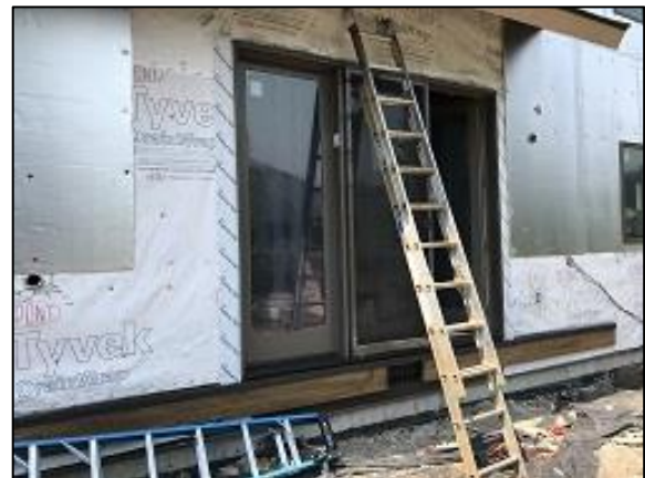
Building E3 Unit #25 Patio Door Installed
