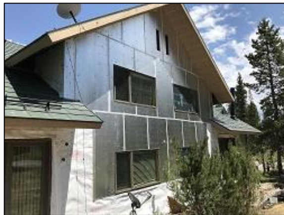
Building E1 Unit #8 & #9 Foam Board Installation
