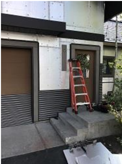
Building E3 Unit 25 Front Door Light & Address Blocking Installed
