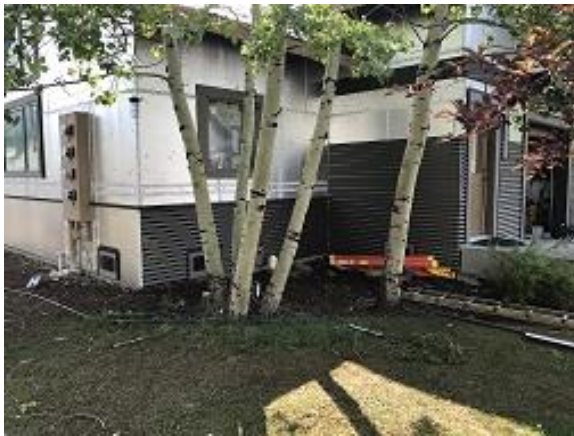
Building E3 Unit 24 Kitchen & Entry Siding Installed
