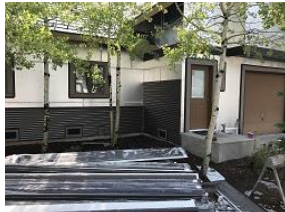
Building E3 Unit 26 Kitchen Windows Corrugated Siding Installed
