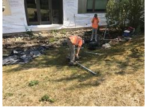
Building E3 Unit 11 Deck Helical Piers Installation
