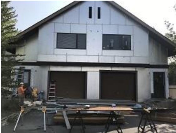
Unit 26 & 27 Garage Belly Band Installed
