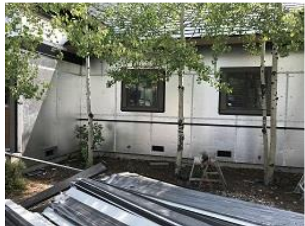
Unit 25 & 26 Kitchen Window Timbertech Trim and J Channel Installed
