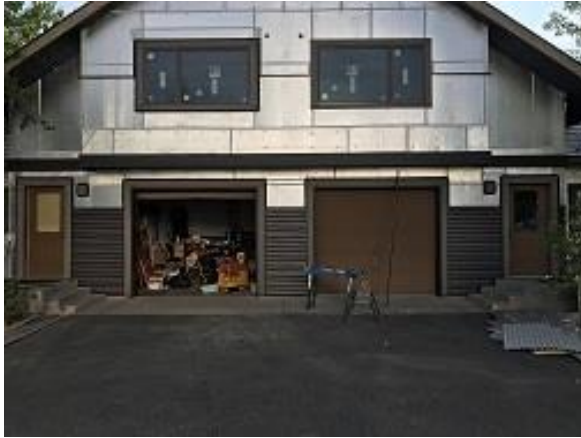
Building E3 Unit 24 & 25 Corrugated Siding Installed
