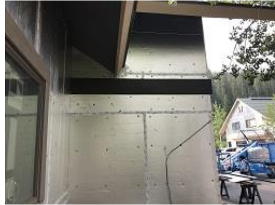
Unit 24 Belly Band Steel Installed
