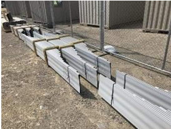
Bridger Steel Delivery
