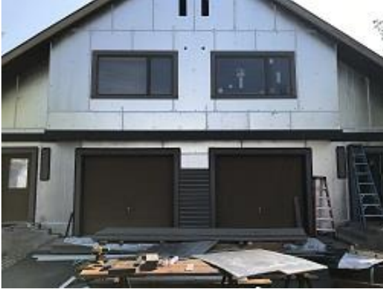
Building E3 Unit 25 & 26 Corrugated Siding Installed
