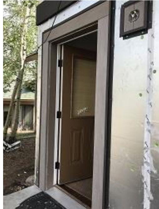
Unit 24 Front Door Timbertech Trim and J Channel Installed
