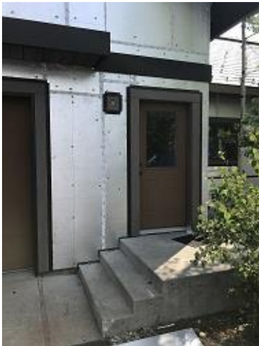
Unit 25 Front Door Timbertech Trim and J Channel Installed
