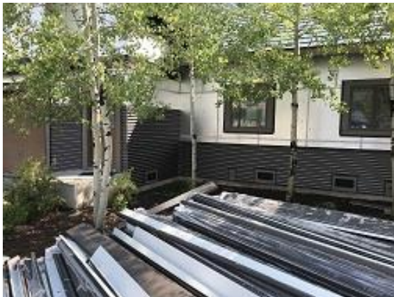
Building E3 Unit 25 & 26 Kitchen Windows Corrugated Siding Installed
