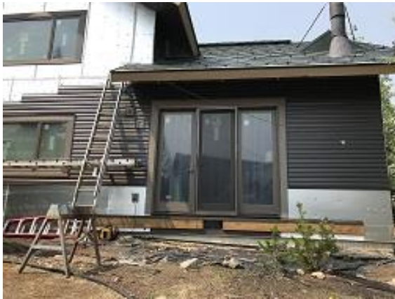
Building E3 Unit 24 Back Siding Install
