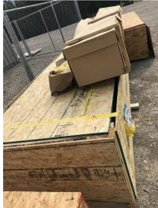
Bridger Steel Siding Delivered
