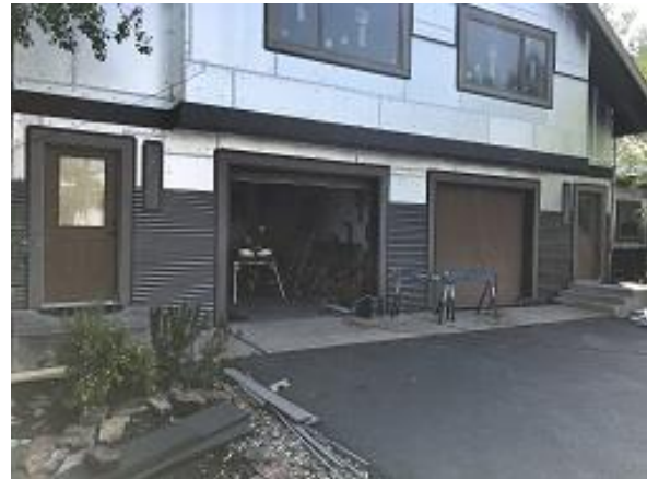
Building E3 Unit 24 & 25 Front Corrugated Installed
