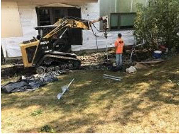
Building E3 Unit 11 Begin Deck Helical Piers Installation
