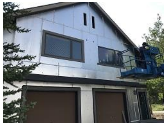
Building E3 Unit 26 & 27 Front Upper Windows Trim Installed
