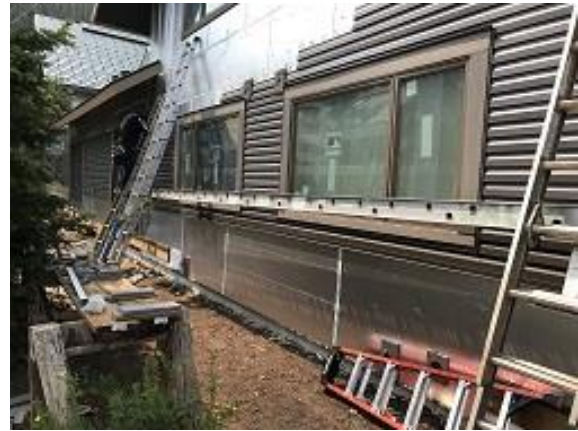
Building E3 Units 24 & 25 Back of Building Siding
