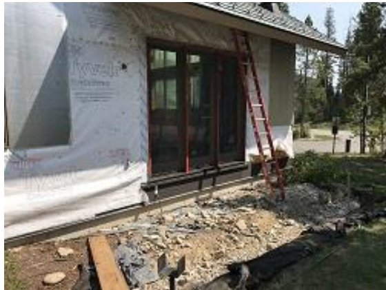
Building E1 Unit 8 Deck Door & Flashing Installed
