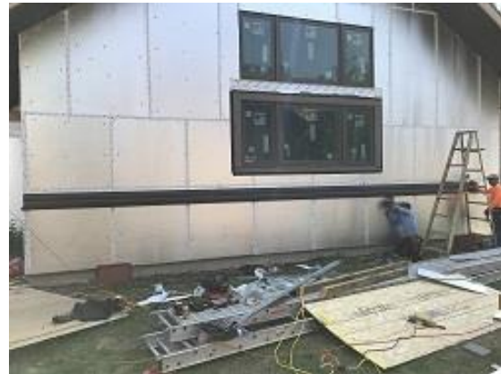
Building E1 Unit 11 Side Lap Siding Installed
