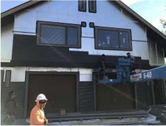
Building E3 Unit 26 & 27 Front Lap Siding Installed
