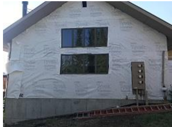
Building E7 Unit 52 Side Tyvek installed
