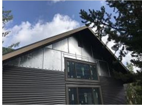
Building E3 Unit 27 Side Board & Batten Siding J Channel Installation
