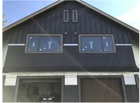
Building E3 Unit 24 & 25 Front Lap Siding Installed
