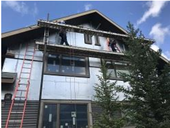
Building E3 Unit 26 & 27 Back Board & Batten Siding Corner Installation
