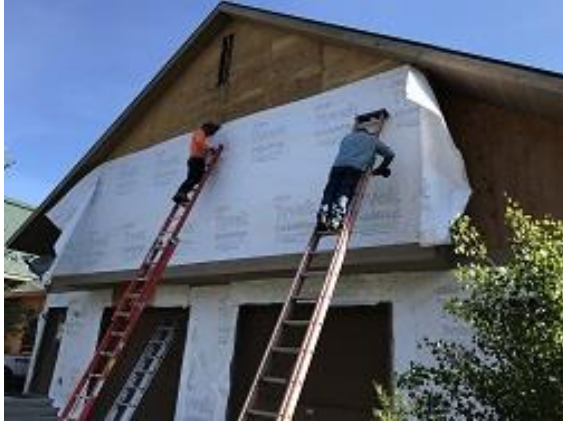
Building E7 Units 49 & 50 Tyvek Installed
