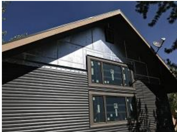
Building E3 Unit 27 Side Board & Batten J Channel Installed
