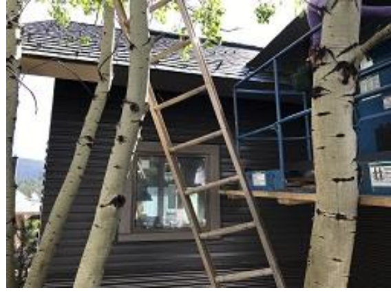
Building E3 Unit 24 Fascia Trim Installed
