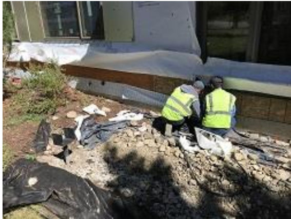
Building E1 Unit 8 base flashing tape Installed
