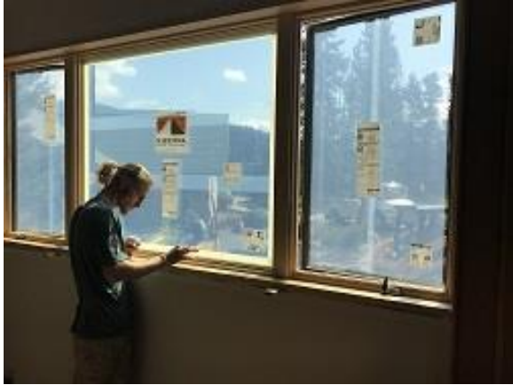
Building E1 Unit 8 Interior Lower Living Room Window Finish Applied
