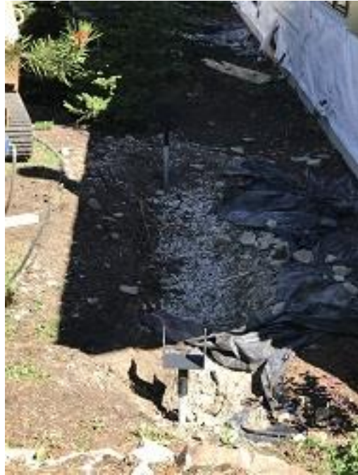
Building E4 Unit 31 Helical Piers Installed
