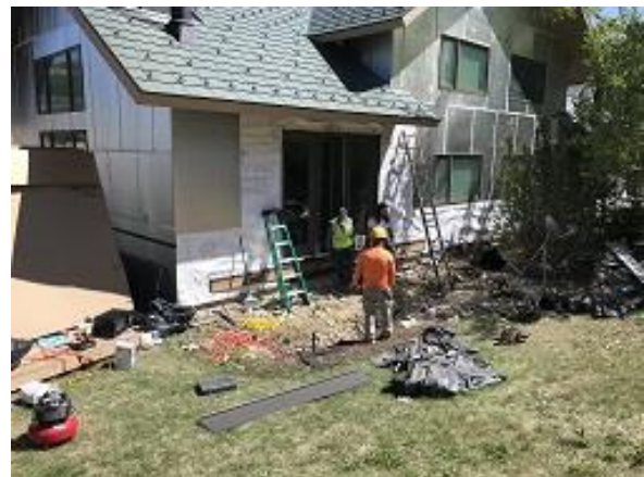
Building E1 Unit 11 Deck Door Reinstalled
