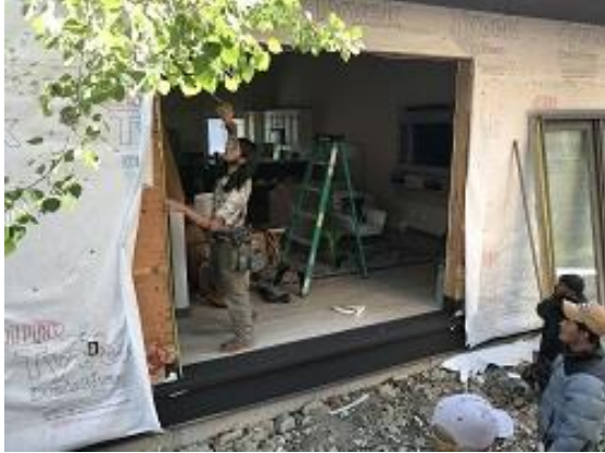
Building E1 Unit 10 Door Pan & Deck Ledger Flashing Installed
