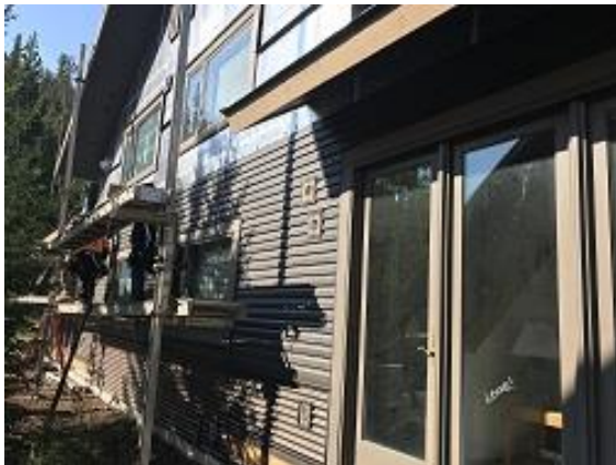
Bldg E3 Units 26 & 27 Back Lap Siding Installed
