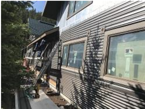
Building E3 Unit 24 & 25 Lap Siding Installed
