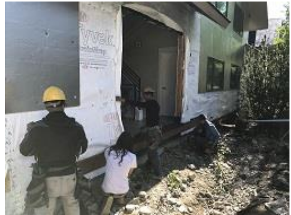
Building E1 Unit 11 Deck Ledger & Door Flashing Installed
