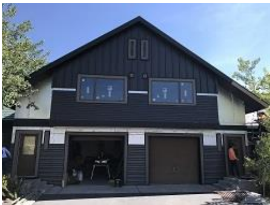
Building E3 Unit 24 & 25 Fascia Installed
