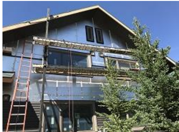
Building E3 Unit 26 & 27 Back Board & Batten J Channel Installed
