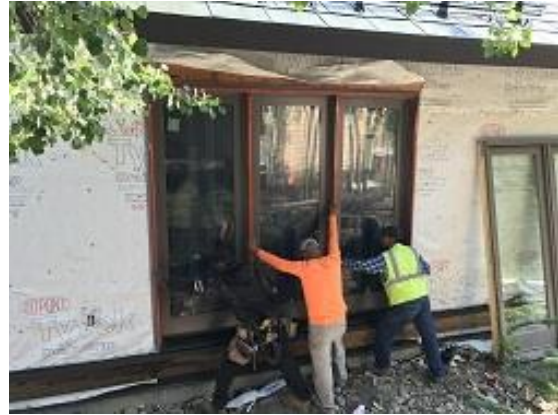
Building E1 Unit 10 Deck Door Installed
