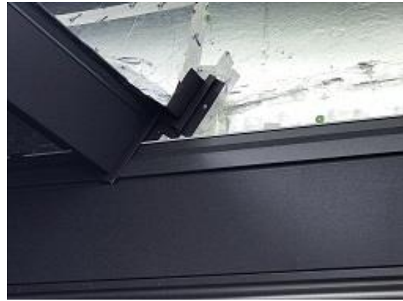
Building E3 Unit 24 Front Diverter & J Channel Installation
