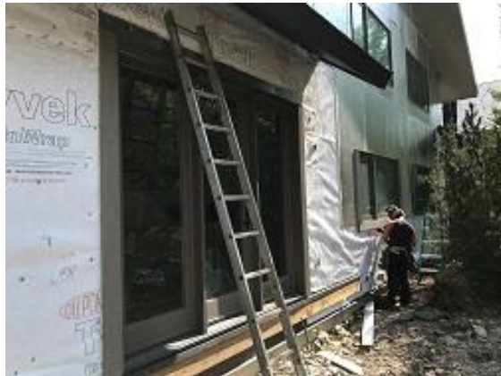
Building E1 Unit 11 Back Window & Door Trim Installed
