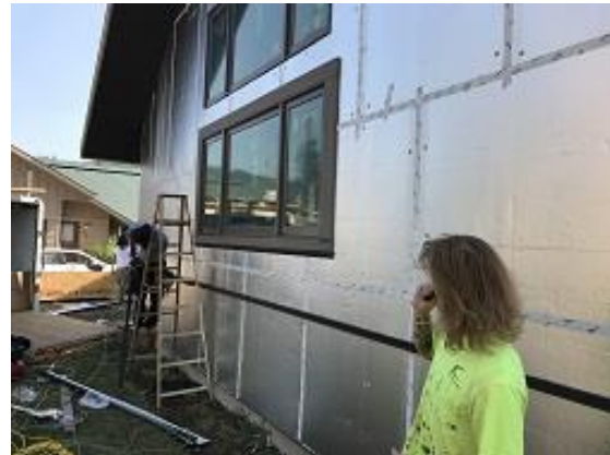
Building E1 Unit 11 Side Window Trim, J Channel Installed
