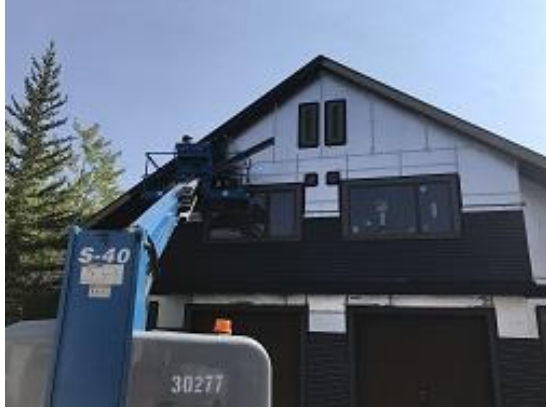
Building E3 Units 26 & 27 Front Facsia Installed
