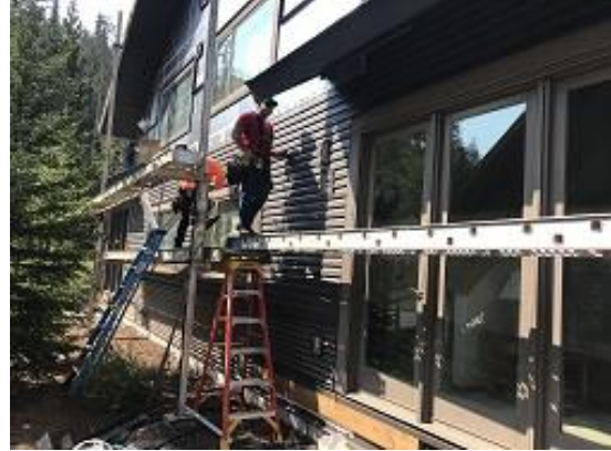
Building E3 Units 26 & 27 Back Lap Siding Installed
