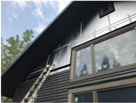
Building E3 Unit 27 Side J Channel Installed
