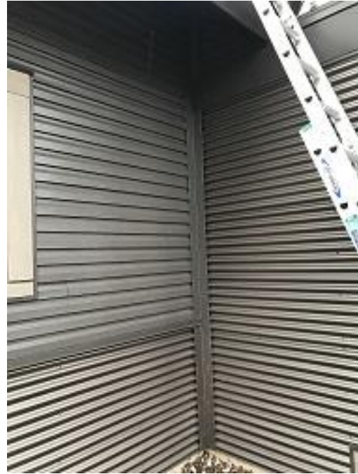
Building E3 Unit 24 Front Inside Corner Installed
