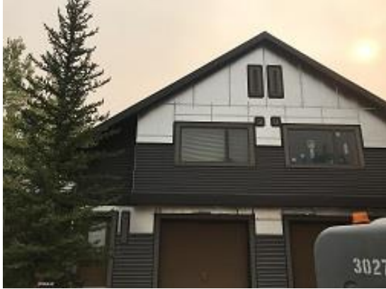
Building E3 Unit 26 & 27 Front Lap Siding Installed
