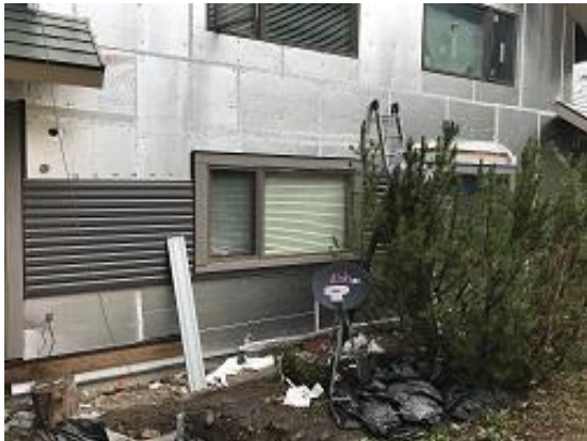
Building E1 Unit 10 Back Lap Siding Installed
