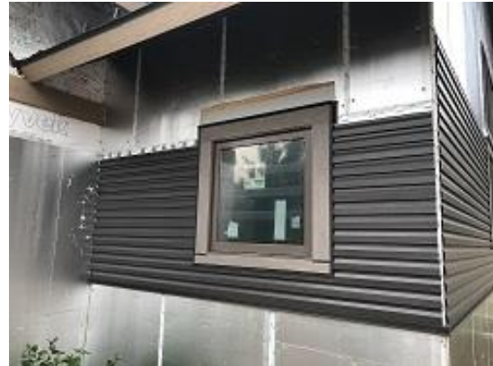
Building E1 Unit 11 Front Lap Siding Installed
