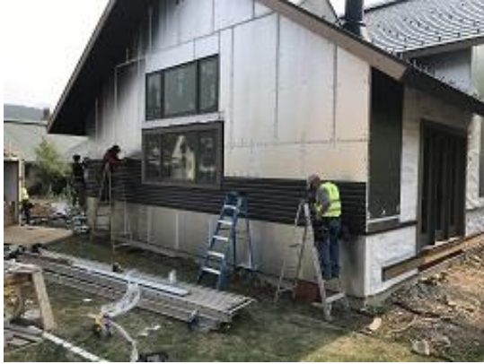
Building E1 Unit 11 Side Lap Siding Installed
