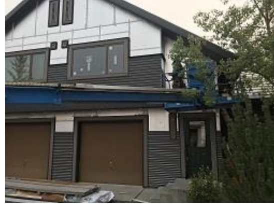
Building E3 Unit 27 Front Lap Siding Installed
