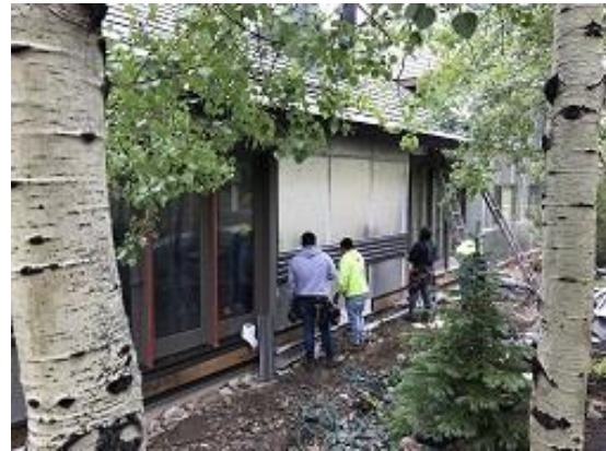
Building E1 Units 9 & 10 Back Lap Siding Installed
