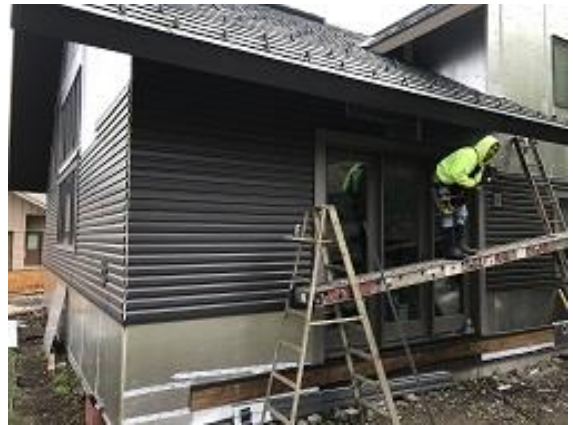
Building E1 Unit 11 Back Lap Siding Installed
