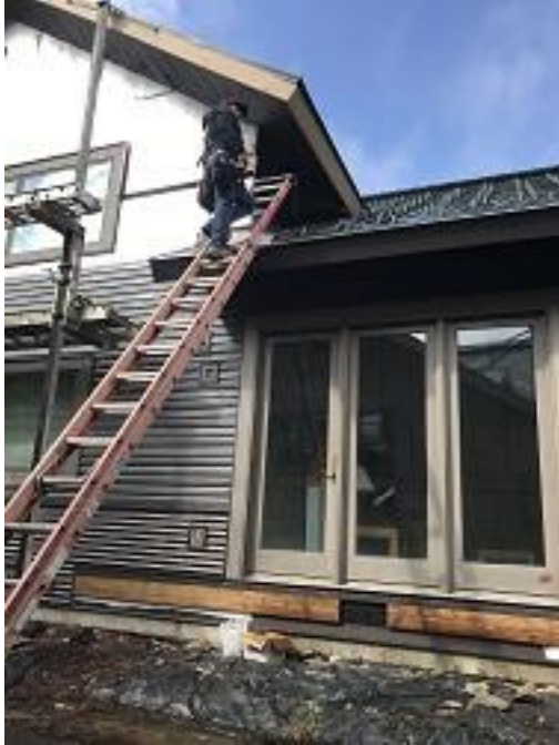
Building E3 Unit 25 Back Flashing and J Channel Installed
