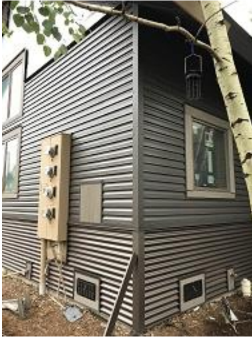
Building E3 Unit 24 Front Corner Installed
