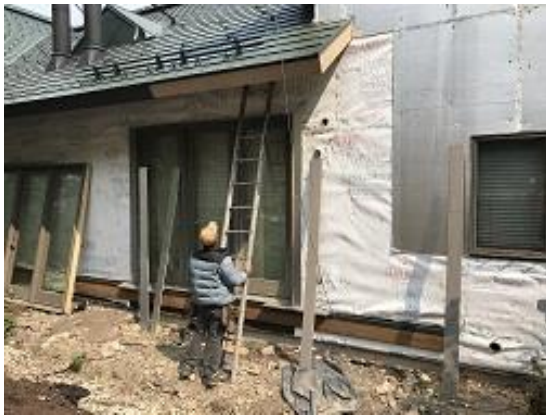
Building E1 Unit 9 Back Door Trim & J Channel Installed
