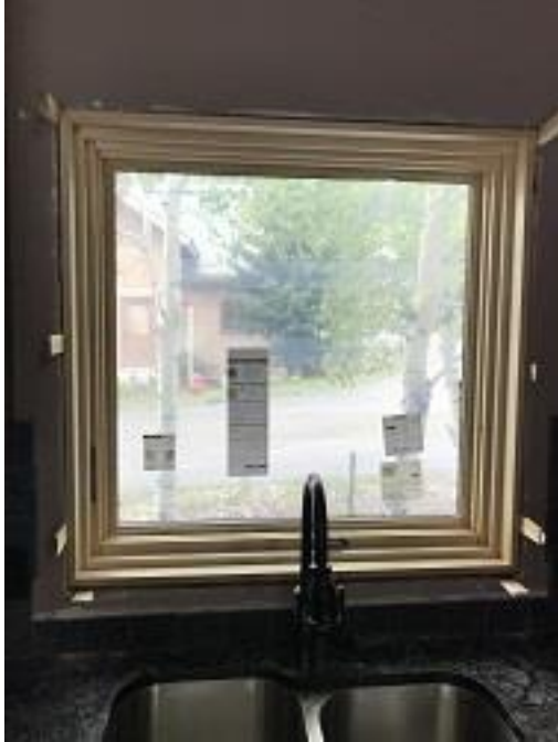
Building F1 Unit 17 Kitchen Window Replaced with Correct Window
