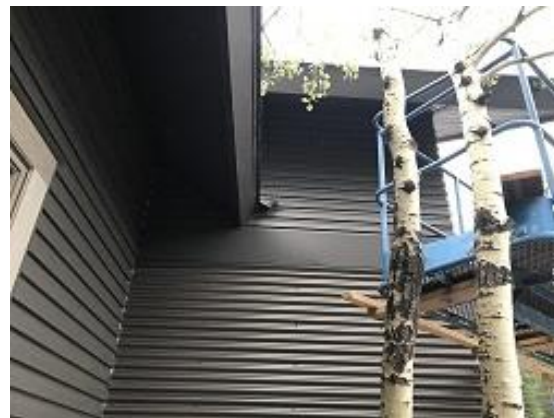
Building E3 Unit 26 Front Upper Lap Siding Installed
