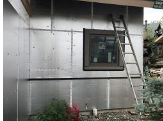
Building E1 Unit 11 Front Window Trim & J Channel Installed
