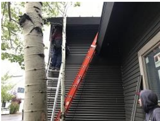
Building E3 Unit 25 Front Upper Lap Siding Installed
