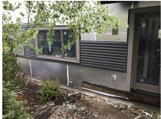
Building E1 Unit 9 Back Lap Siding Installed
