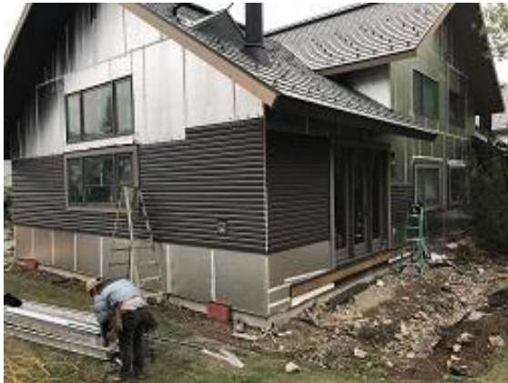
Building E1 Unit 11 Side & Back Lap Siding Installed
