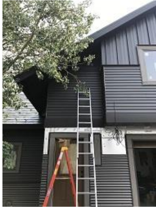
Building E3 Unit 24 Front Lap Siding Completed
