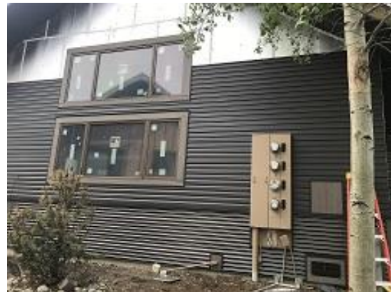
Building E3 Unit 24 Side Lap Siding Completed
