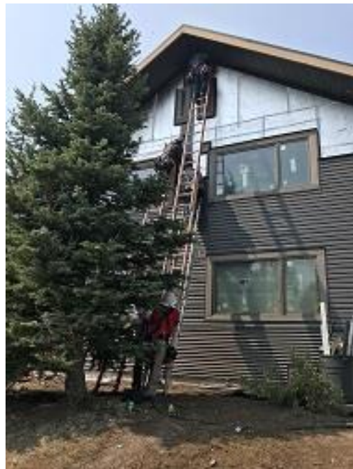
Building E3 Units 24 & 25 Back Board and Batten Siding Installed
