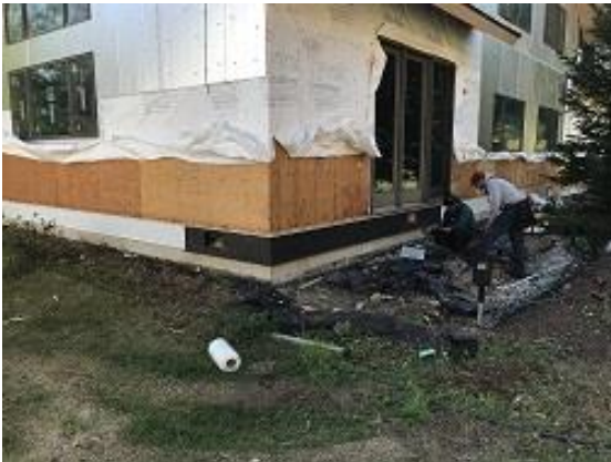
Building E4 Unit 28 Back Base Flashing Installed
