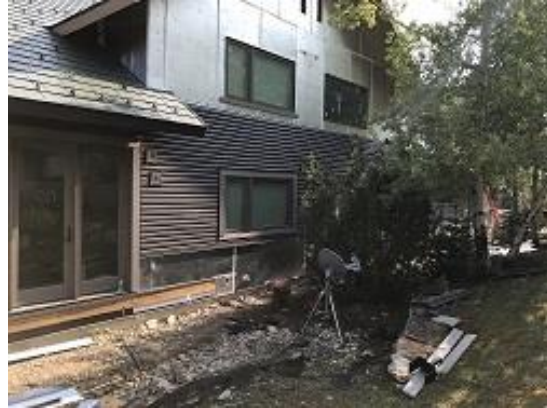
Building E1 Unit 11 & 10 Back Lap Siding Installed
