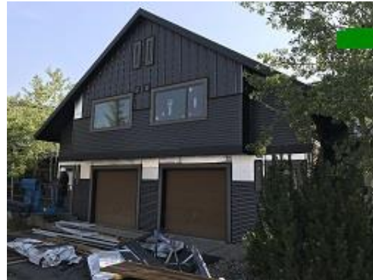
Building E3 Units 26 & 27 Front Board and Batten Installed
