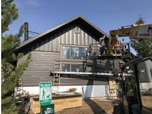
Building E1 Unit 8 Side Board and Batten Installed
