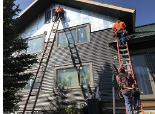
Building E3 Unit 28 Back Board & Batten Flashing Installed
