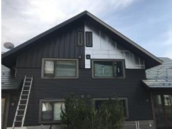
Building E1 Units 8 & 9 Board and Batten Installed
