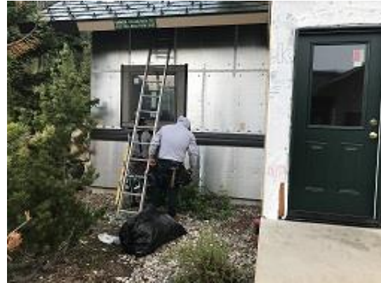
Building E1 Unit 8 Lap Siding Installed
