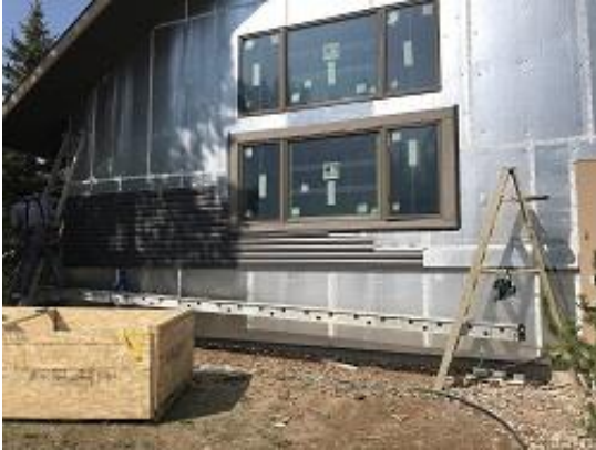
Building E1 Unit 8 Side Lap Siding Installed
