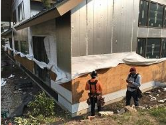
Building E4 Unit 31 Base Flashing Installed
