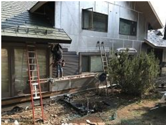
Building E1 Unit 9 Back Lap Siding Installed
