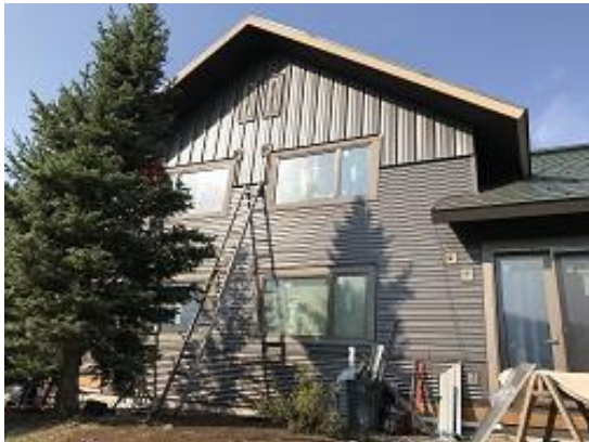
Building E3 Units 24 & 25 Back Board and Batten Installed
