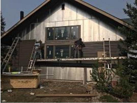
Building E1 Unit 8 Side Lap Siding Installed
