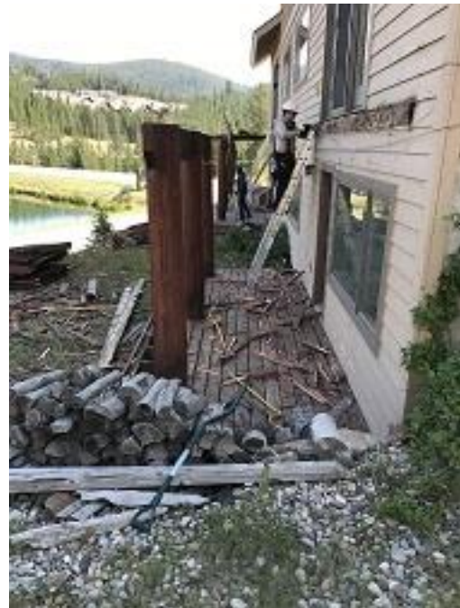
Building F2 Unit 19 Deck Demo
