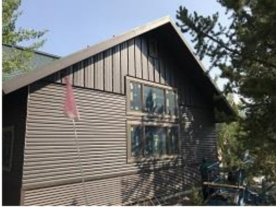
Building E3 Unit 27 Side Board & Batten Installed
