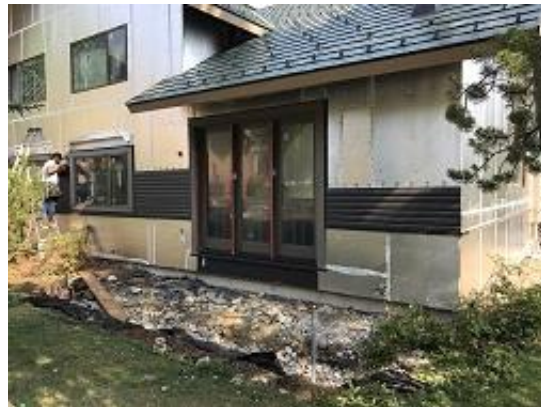
Building E1 Unit 8 Back Lap Siding Installed
