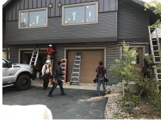
Building E3 Units 24 & 25 Front Corrugated Siding Installed
