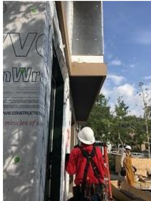
Building E4 Units 28 & 29 Soffit Installed
