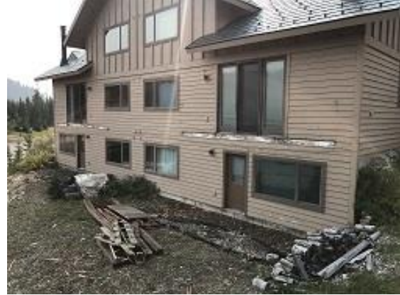
Building F2 Units 18 & 19 Deck Demo Completed
