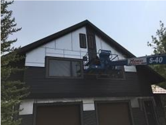
Building E3 Units 26 & 27 Front Board and Batten Siding Installed
