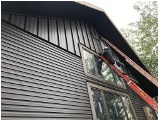
Building E3 Unit 24 Board and Batten Installed
