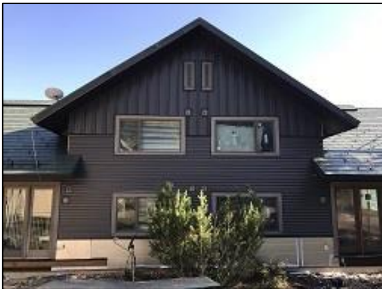
Bldg E1 Units #8 & #9 Rear Board & Batten Siding
