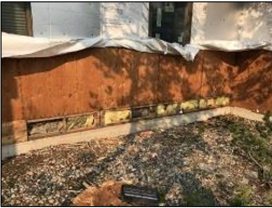
Bldg E4 Units #29 & #30 Front Sheathing Repair
