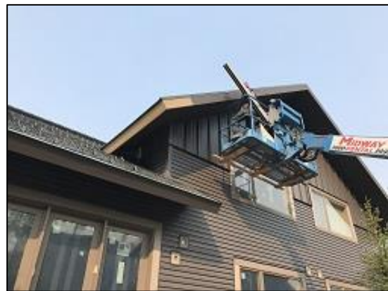
Bldg E3 Unit #27 Rear Fascia Installation
