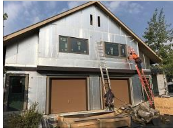
Bldg E4 Units #28 & #29 J-Channel Installation
