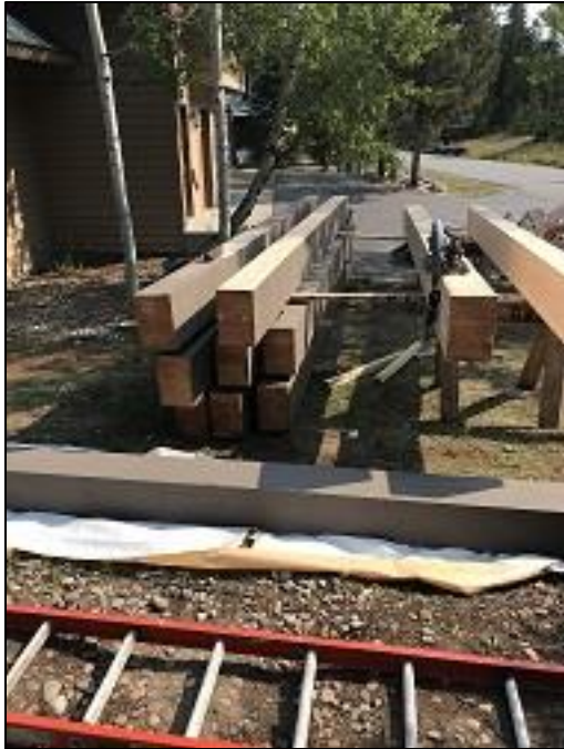
Painting of Deck Beams
