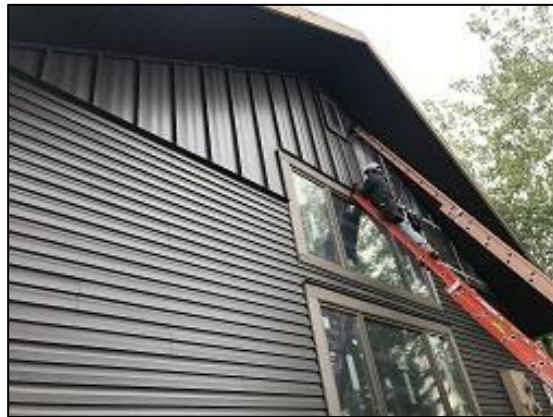
Bldg E3 Unit #24 Board and Batten Installed
