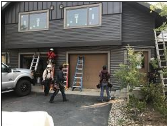
Bldg E3 Units #24 & #25 Front Corrugated Siding
