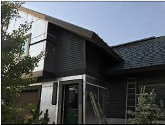
Bldg E1 Unit #11 Front Lap Siding Installed
