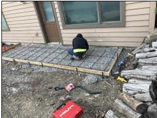
Bldg F2 Unit #19 Concrete Patio Prep
