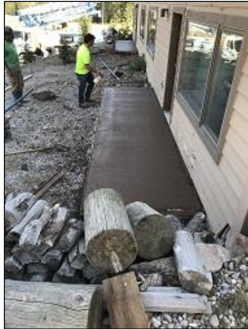
Bldg F2 Units #18 & #19 Concrete Patios Installed
