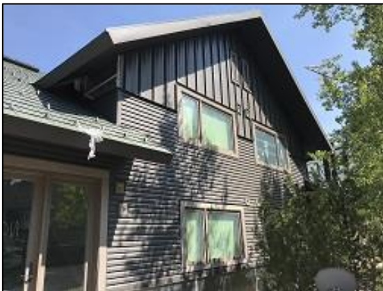
Bldg E1 Units #10 & #11 Rear Board & Batten
