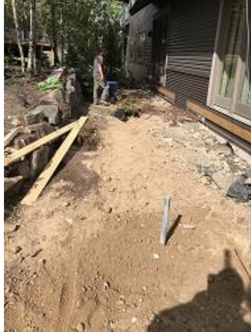
Building E1 Units 9 & 10 Fill Dirt Installation
