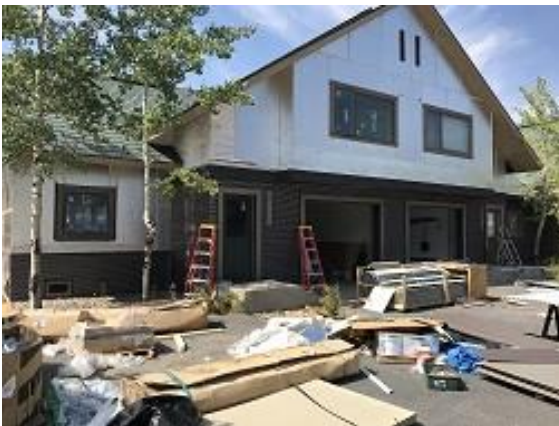
Building E4 Unit 31 & 30 Front Corrugated Siding Installed
