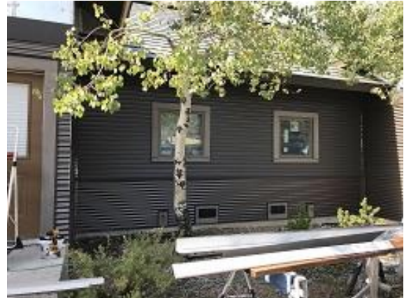
Building E4 Units 30 & 29 Front Lap Siding Installed
