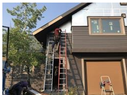
Building E4 Unit 29 Front Lap Siding Installation
