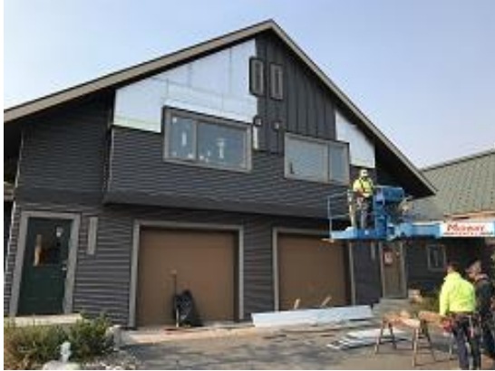
Building E1 Units 8 & 9 Board and Batten Siding Installation
