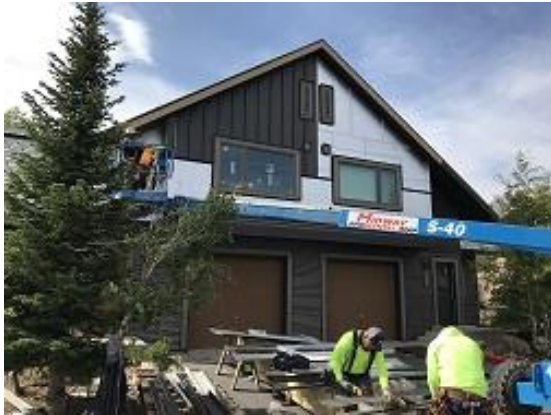
Building E1 Units 10 & 11 Board and Batten Siding Installation
