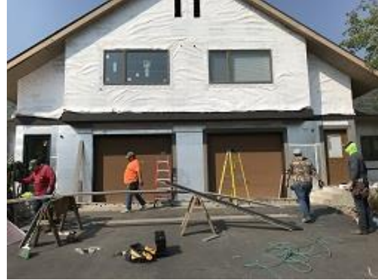
Building E2 Units 20 & 21 Foam Board & Door and Window Trim Installation
