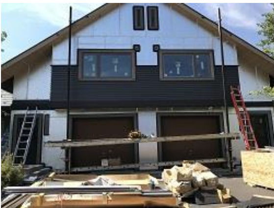
Building E4 Units 28 & 29 Front Lap Siding Installed
