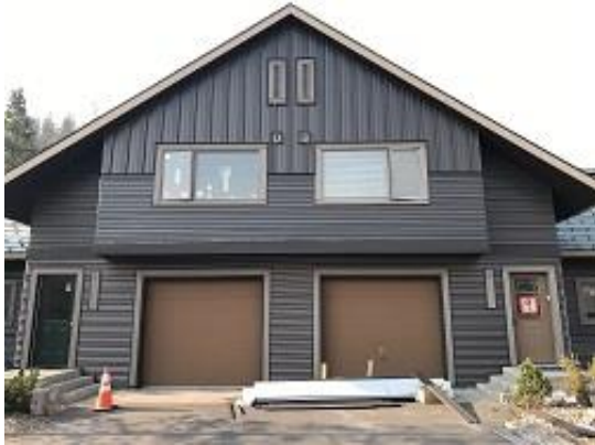
Building E1 Units 8 & 9 Front Board and Batten Siding Installation
