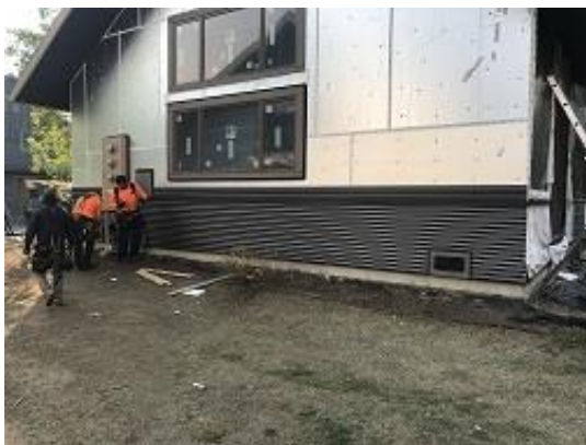
Building E4 Unit 28 Side Lap Siding Installation
