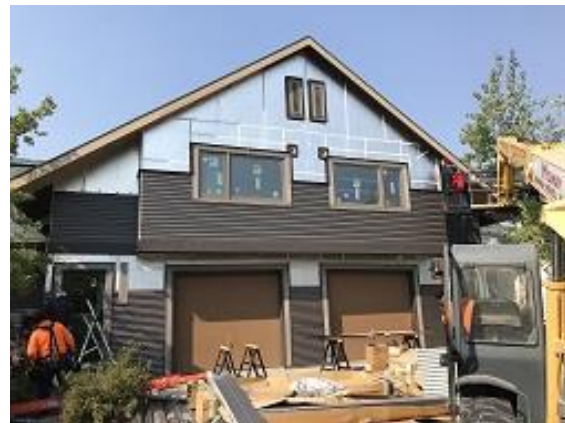
Building E4 Units 30 & 31 Corrugated & Board and Batten Siding Installation
