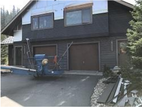
Building E1 Units 8 & 9 Front Lap Siding Installed
