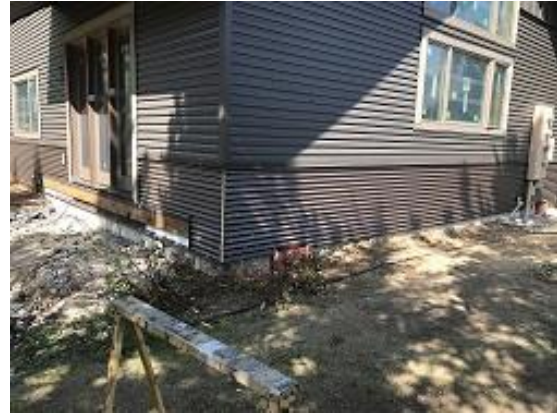
Building E1 Unit 8 Corrugated Siding Installed
