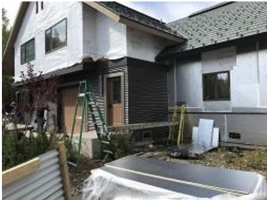
Building E2 Unit 20 Corrugated Siding Installation
