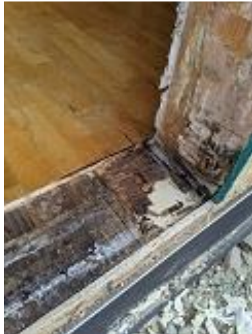
Building E4 Unit 28 Deck Door Installation
