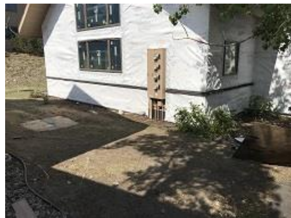
Building E2 Unit 23 Wainscoting & Base Flashing Installation
