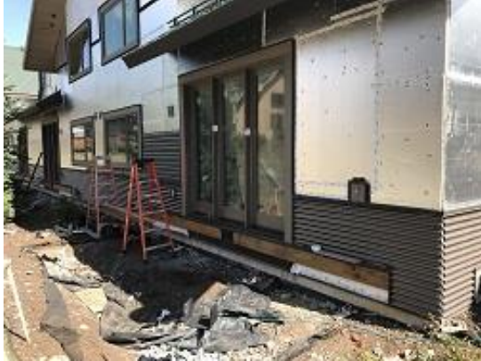
Building E2 Unit 23 Back Corrugated Siding Installed
