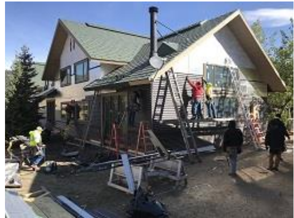
Building E2 Unit 23 Back & Side Lap Siding Installed
