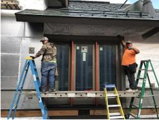
Building E2 Unit 23 Deck Door Installation
