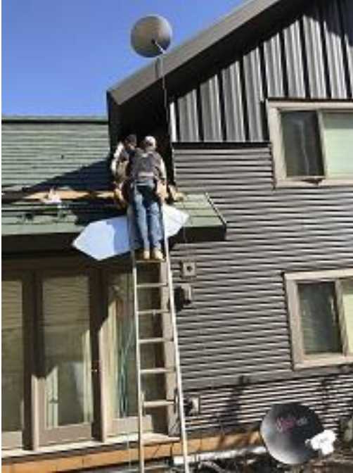
Building E1 Unit 9 Back Lap & Board and Batten Siding Installed
