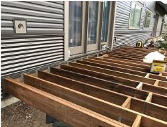
Building E3 Unit 27 Deck Framing Installed
