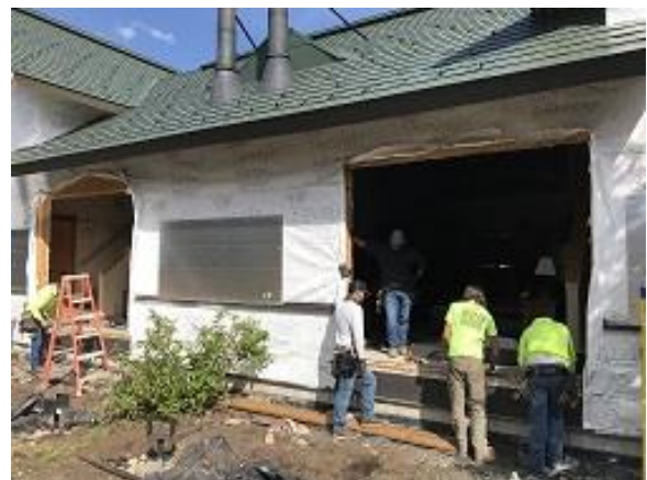
Building E2 Units 21 & 22 Deck Door Threshold Pan Flashing Installed
