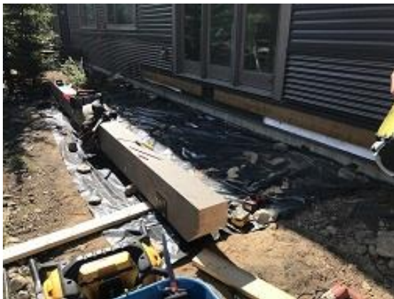
Building E3 Unit 26 Deck Framing Began
