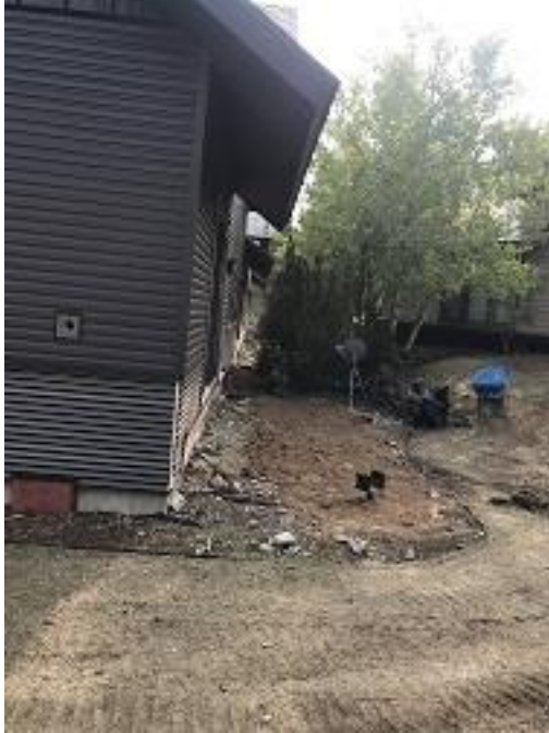
Building E1 Unit 11 Deck Back Fill Installed
