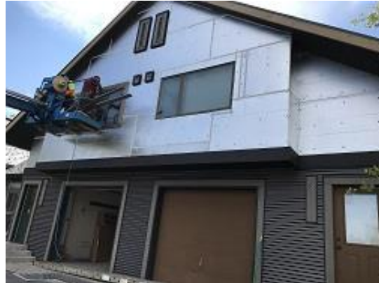
Building E2 Units 20 & 21 Front Window Trim and J Channel Installed
