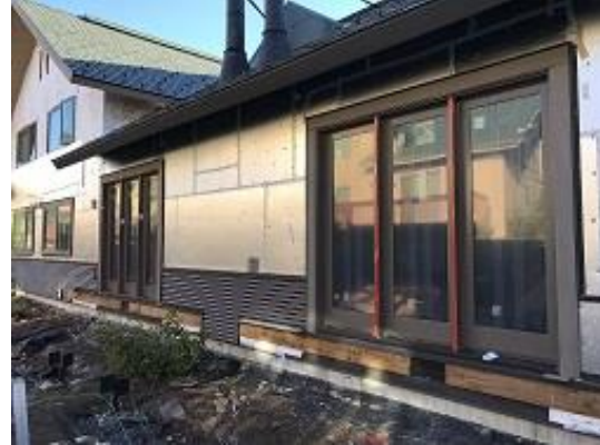
Building E2 Units 21 & 22 Deck Door Trim and J Channel Installation
