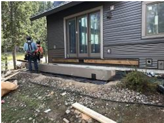
Building E3 Unit 27 Deck Framing Began
