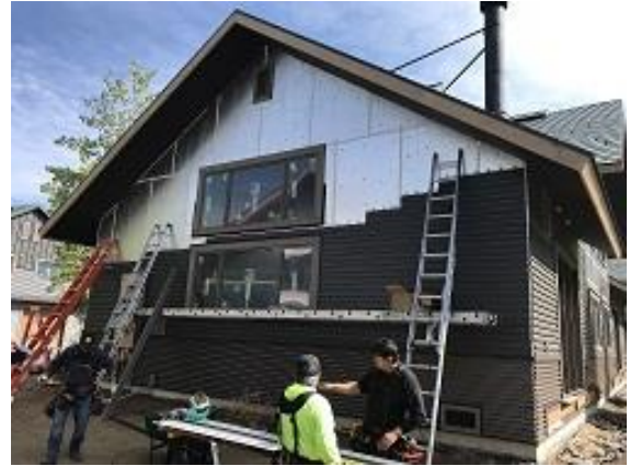
Building E4 Unit 28 Side Lap Siding Installed
