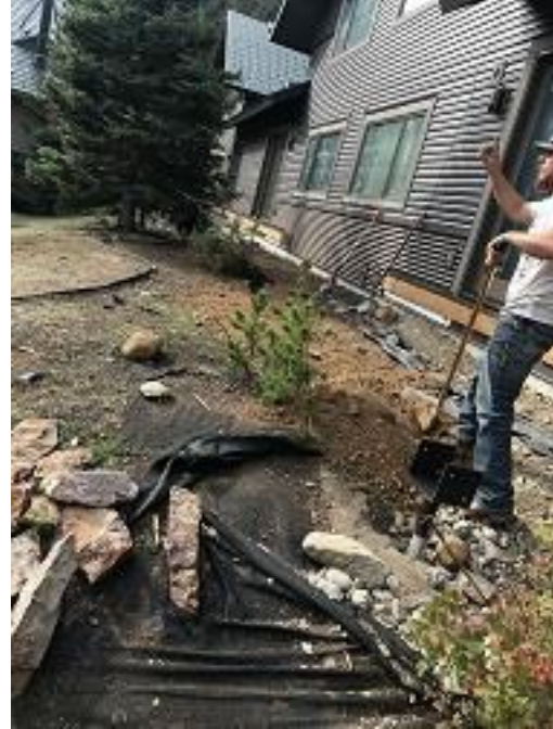
Building E3 Unit 24 Deck Back Fill Installed
