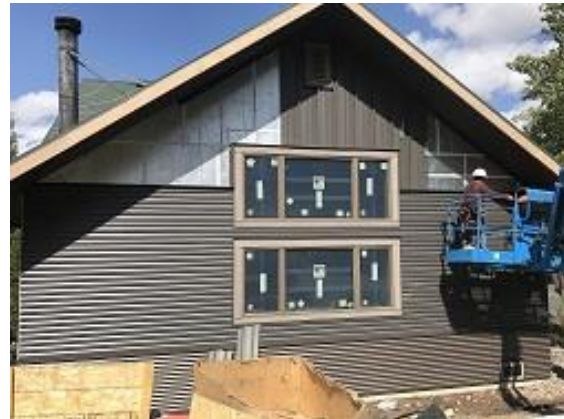
Building E4 Unit 31 Side Board and Batten Siding Installed
