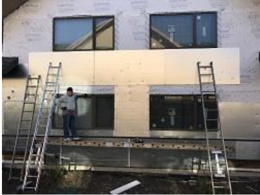
Building E2 Units 20 & 21 Back Foam Board and J Channel Installed
