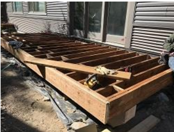
Building E3 Unit 26 Deck Framing Completed
