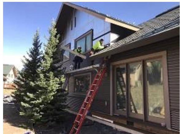
Building E4 Units 28 & 29 Back Lap Siding Installed
