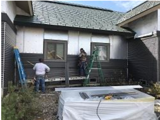
Building E2 Units 21 & 22 Front Lap Siding and J Channel Installed
