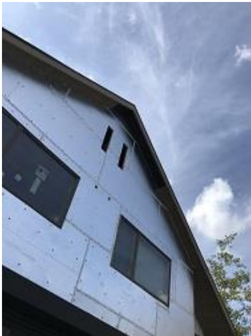
Building E2 Units 20 & 21 Front Soffit Installed
