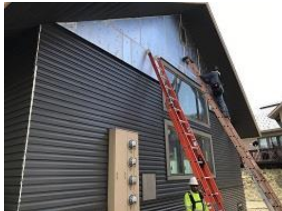
Building E4 Unit 28 Side Lap Siding Installed
