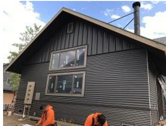
Building E4 Unit 28 Side Board and Batten Installation
