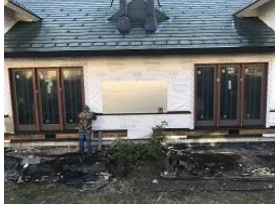
Building E2 Units 21 & 22 Back Foam Board and J Channel Installed
