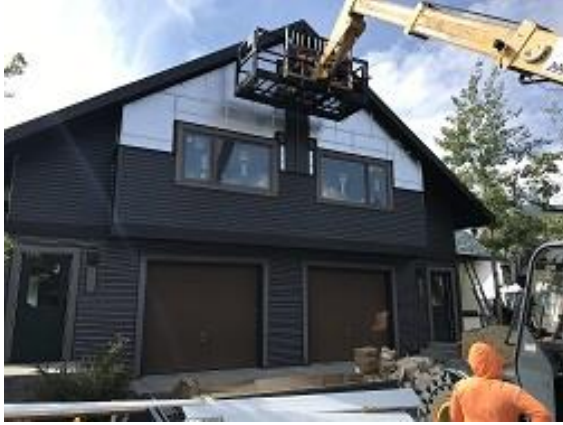
Building E4 Units 28 & 29 Board and Batten Siding Installed
