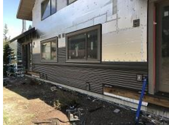
Building E2 Units 20 & 21 Back Lap Siding Installed
