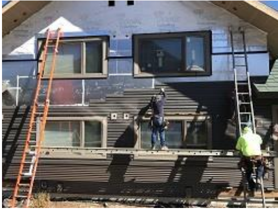
Building E2 Units 20 & 21 Back Lap Siding Installed
