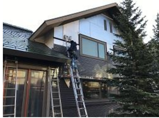
Building E2 Unit 22 Back Lap Siding Installed
