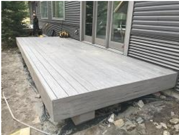
Building E3 Unit 26 Deck Fascia Installed
