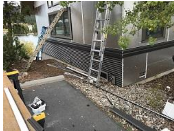
Building F1 Unit 17 Side Corrugated Siding Installed
