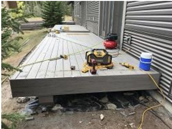
Building E3 Unit 25 Decking Installed
