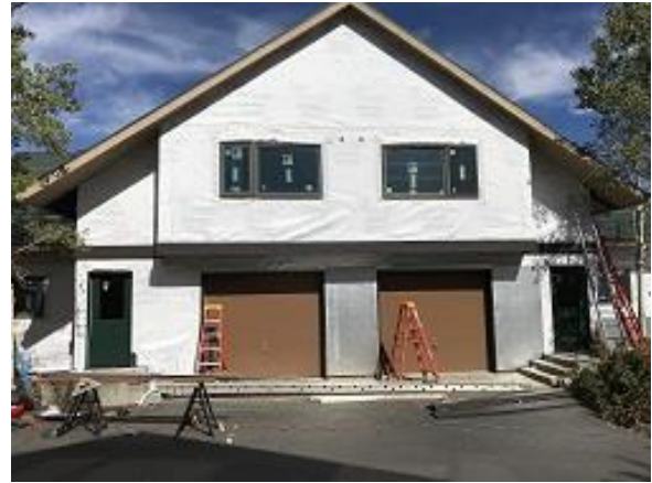
Building F1 Units 16 & 17 Front Foam Board Installed
