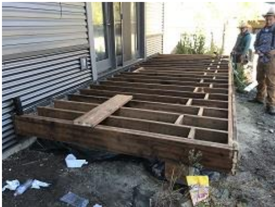
Building E3 Unit 24 Deck Framing Completed
