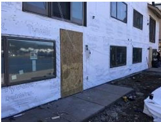
Building F1 Units 16 & 17 Back Base Flashing Installed
