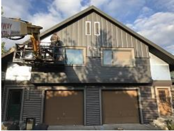
Building E2 Units 22 & 23 Front Board and Batten Siding Installed
