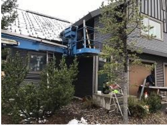
Building E1 Unit 8 Front Lap Siding Installed
