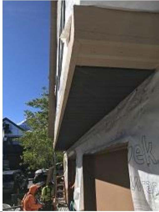
Building F1 Units 16 & 17 Soffit Installed
