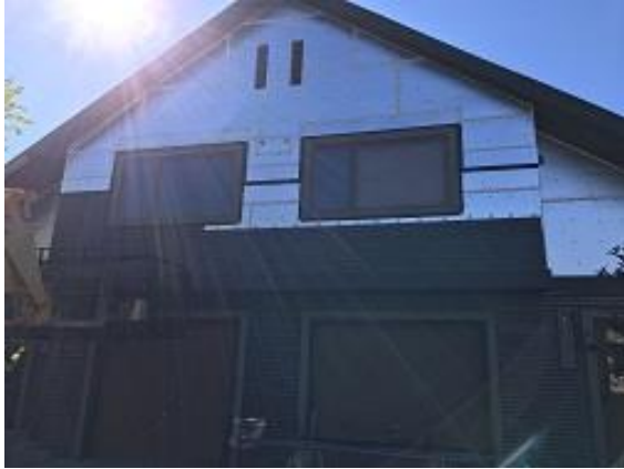
Building E2 Units 22 & 23 Front Lap Siding Installed
