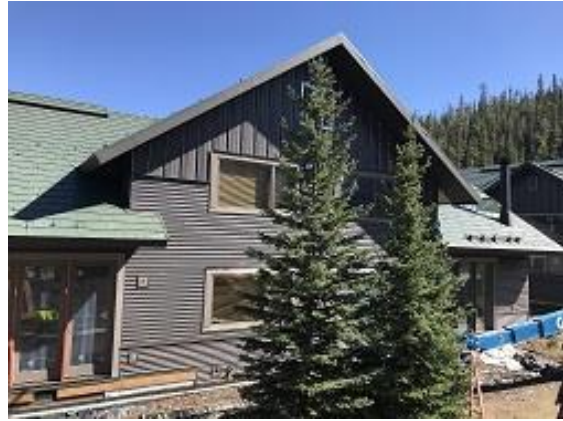
Building E2 Units 22 & 23 Back Board and Batten Siding Installed
