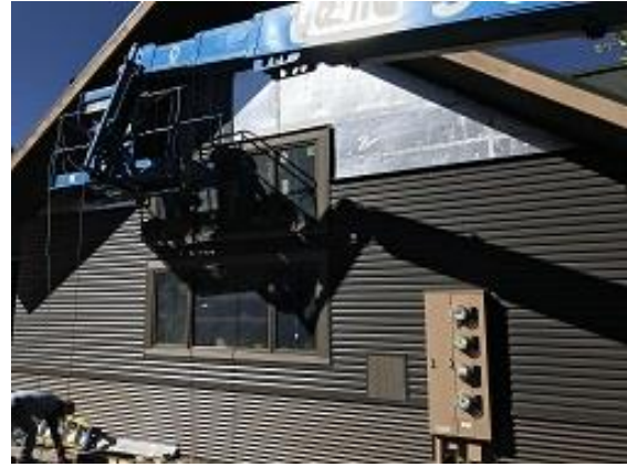
Building E2 Unit 23 Side Board and Batten Siding Installed
