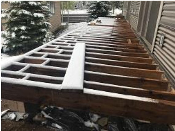
Building E3 Unit 25 Deck Framing Completed
