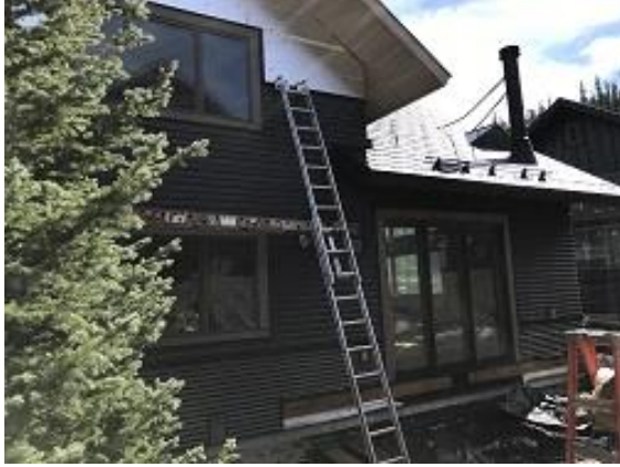
Building E2 Unit 23 Back Lap Siding Installed
