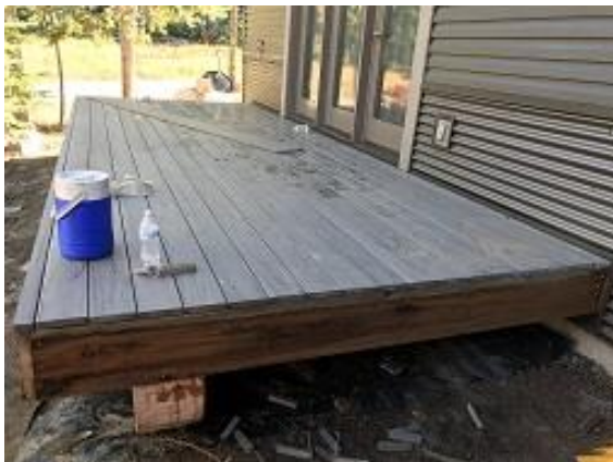
Building E3 Unit 27 Decking Installed
