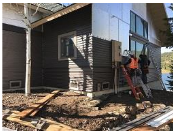
Building F1 Unit 16 Side Lap Siding Installed
