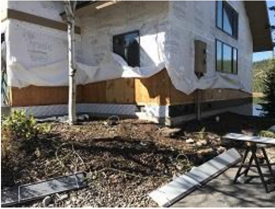
Building F1 Unit 16 Base Flashing Installed
