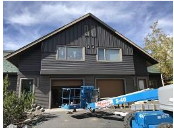
Building E2 Units 20 & 21 Front Fascia Installed
