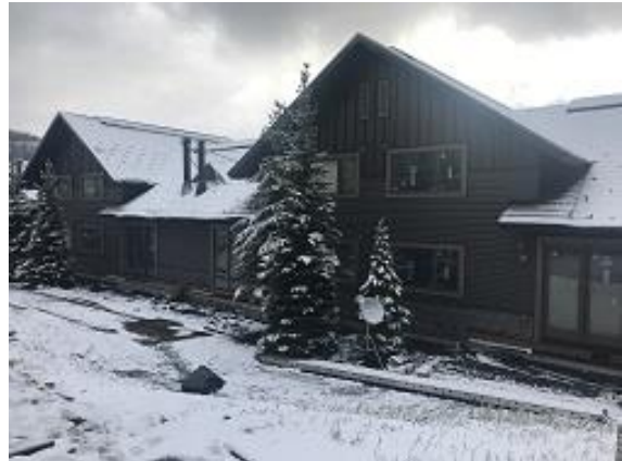
Building E4 Units 28 - 31 Back Board and Batten Completed
