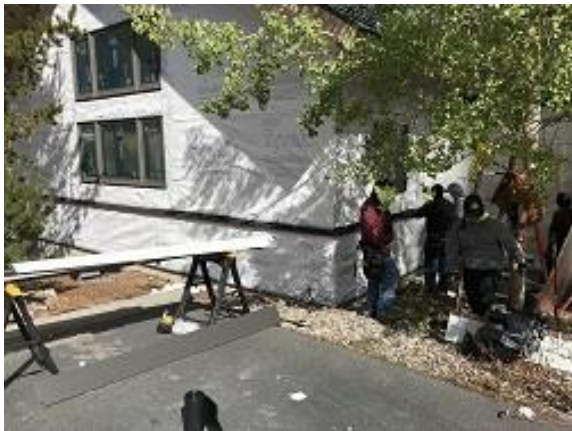
Building F1 Unit 17 Side & Front Wainscot Flashing and Foam Board Installed
