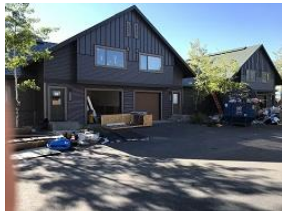
Building E4 Units 28 - 31 Siding Completed
