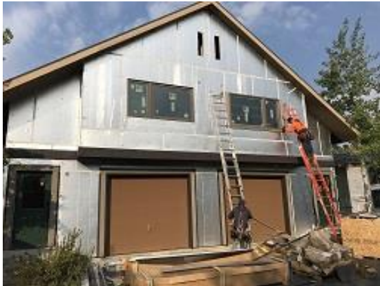
Building E4 Units 28 & 29 Front J Channel Installed
