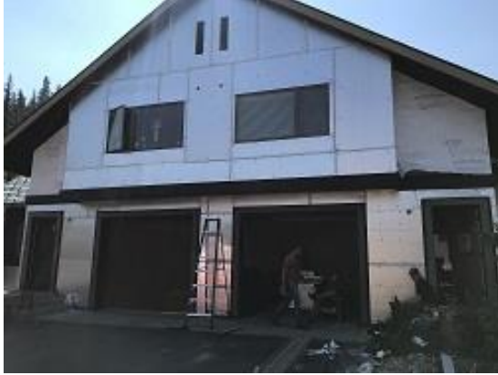
Building E1 Units 8 & 9 Garage Trim and Foam Board Installed
