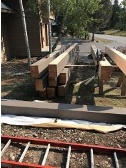
Deck Beam Painting
