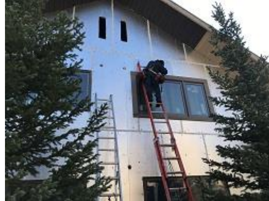
Building E4 Unit 29 Back Window Trim Installed
