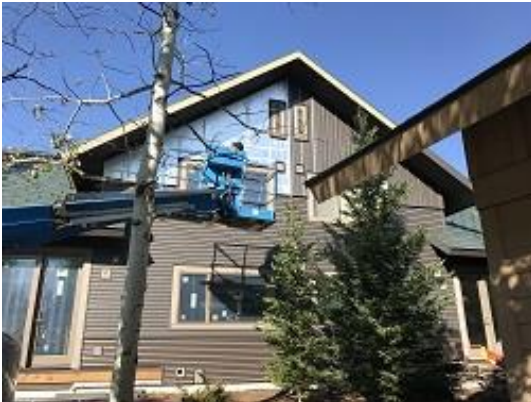
Building E3 Unit 27 Back Board and Batten Siding Installed
