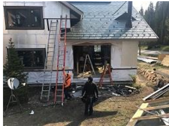
Building E4 Unit 31 Deck Door Installed
