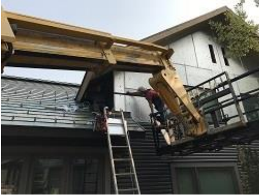
Building E1 Unit 11 Back Soffit and Fascia Installation Continued
