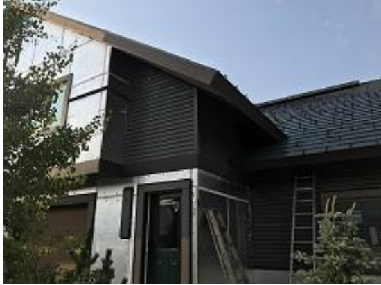
Building E1 Unit 11 Front Lap Siding Installed
