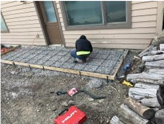
Building F2 Unit 19 Concrete Patio Prep
