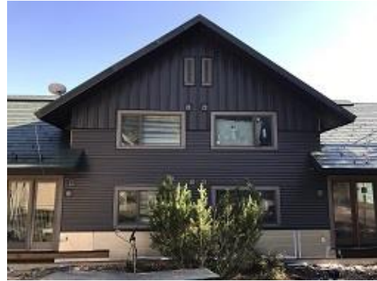
Building E1 Units 8 & 9 Back Board and Batten Siding Installed
