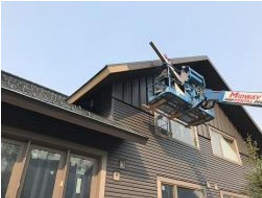
Building E3 Unit 27 Back Fascia Installation
