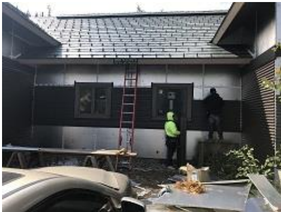
Building E1 Units 9 & 10 Front Lap Siding Installed
