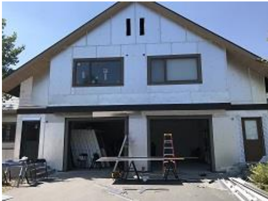
Building E4 Units 30 & 31 Garage Trim, Foam Board and J Channel Installed
