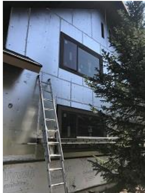
Building E4 Units 28 Foam Board and J Channel Installed
