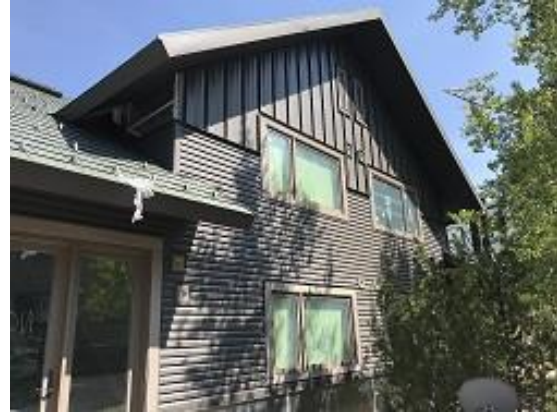
Building E1 Units 10 & 11 Back Board and Batten Installed
