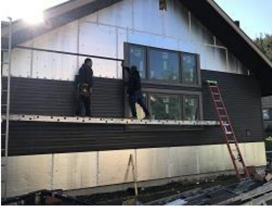
Building E1 Unit 11 Side Lap Siding Installed
