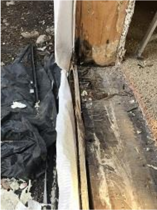
Building E4 Unit 31 Deck Door Framing Damage Repaired
