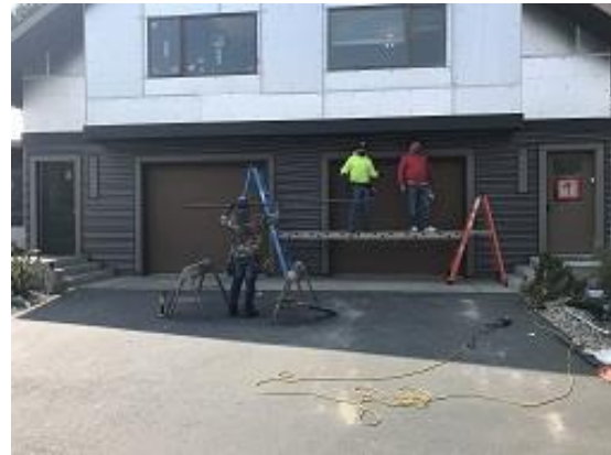
Building E1 Units 8 & 9 Front Corrugated Siding Installed
