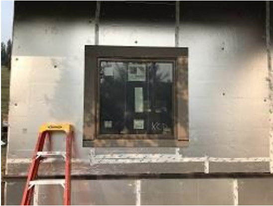
Building E4 Unit 31 Front Window Trim, Base Flashing & Foam Board Installation
