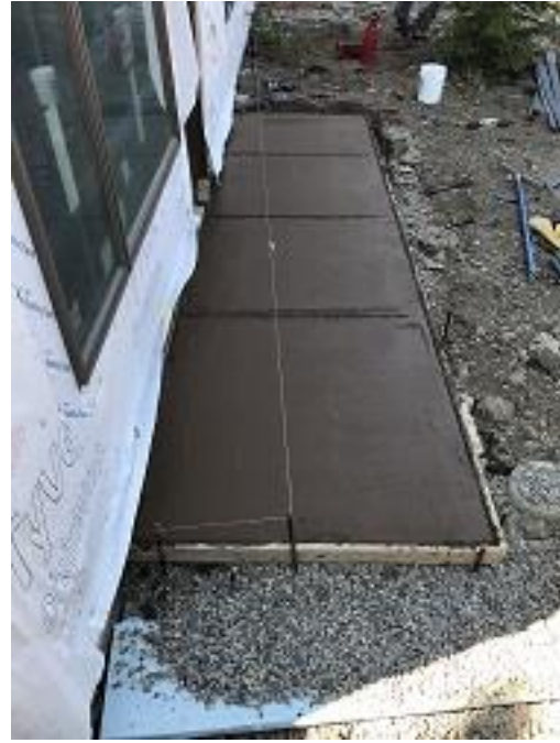
Building F1 Units 16 & 17 Concrete Patios Installed
