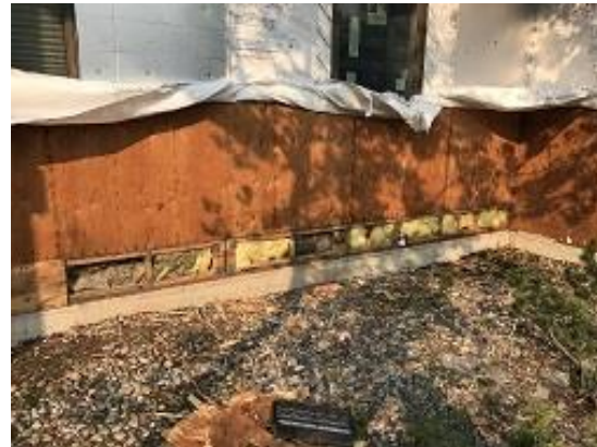
Building E4 Units 29 & 30 Front Sheathing Repair
