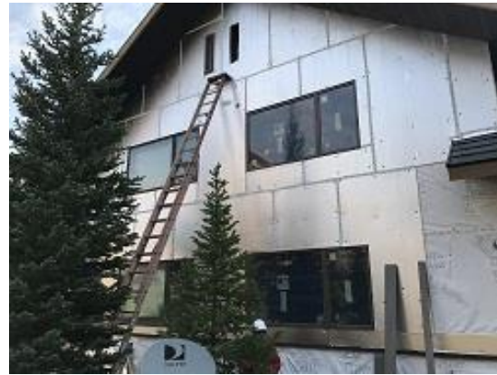
Building E4 Units 30 & 31 Back Vents & J Channel Installed
