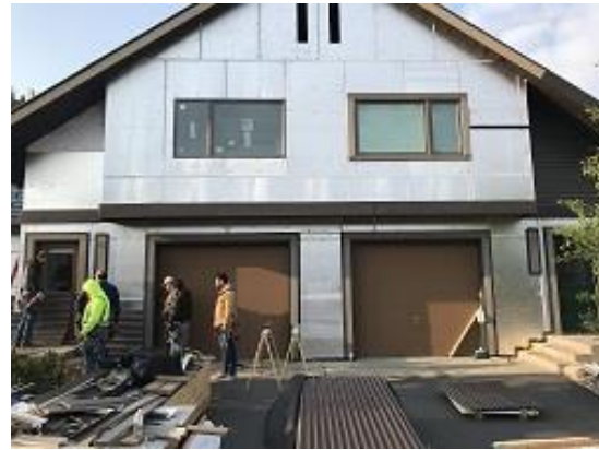
Building E1 Unit 10 Front Corrugated Siding Installed
