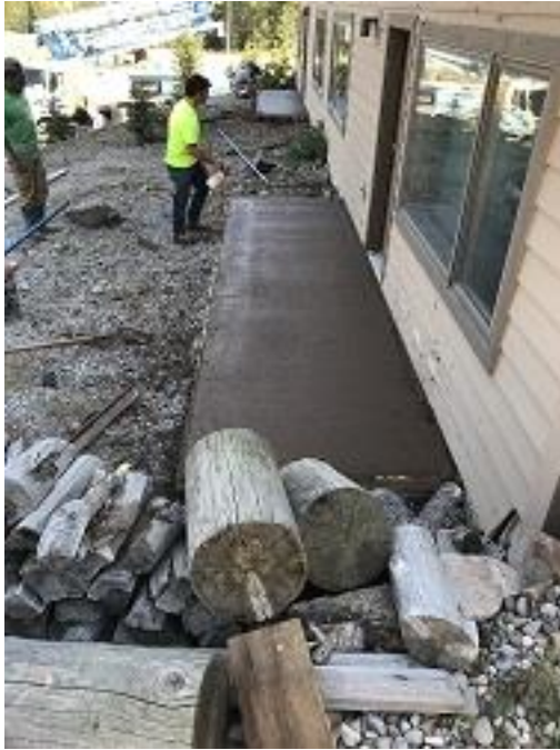
Building F2 Units 18 & 19 Concrete Patios Installed
