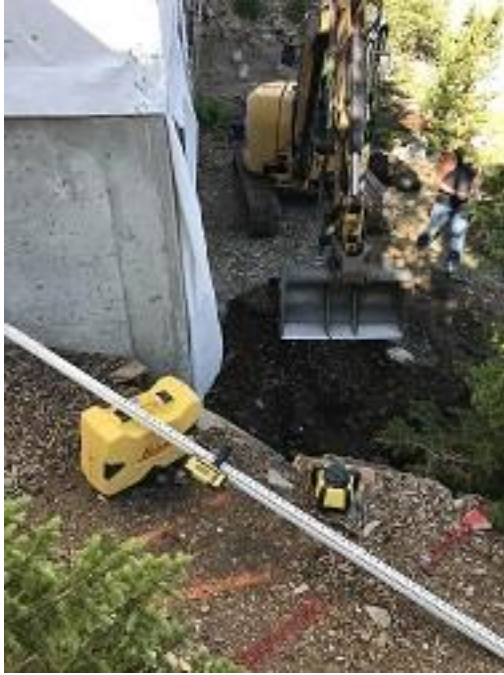
Building F1 Unit 16 Concrete Patio Preparation Continued
