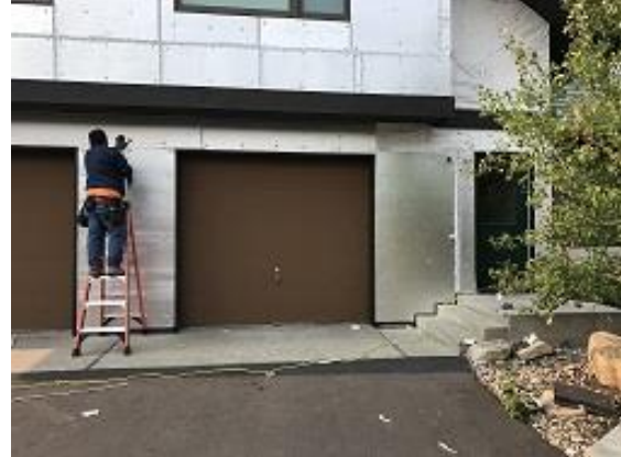
Building E1 Unit 10 & 11 Front Garage Foam Board and Trim Installation
