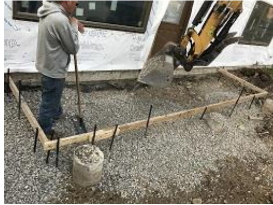
Building F1 Unit 16 Concrete Patio Prep
