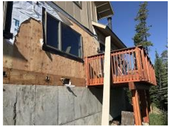
Building E7 Unit 52 Siding Demo Continued
