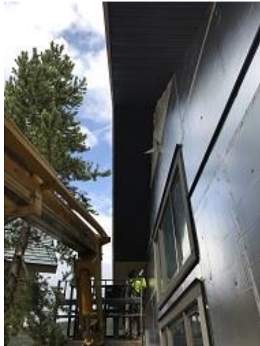
Building F1 Unit 17 Side Soffit Installed
