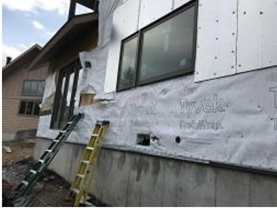
Building E7 Unit 49 Back Base & Wainscot Flashing Installed
