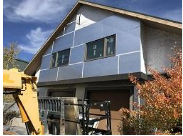
Building E7 Units 49 & 50 Front Foam Board Installed
