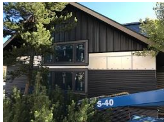
Building F1 Unit 17 Side Board and Batten Siding Installed
