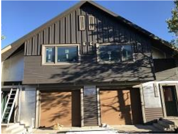
Building F1 Units 16 & 17 Front Board and Batten Siding Installed
