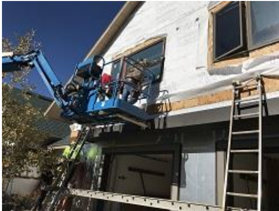
Building E7 Unit 50 Front Upper Window Installed
