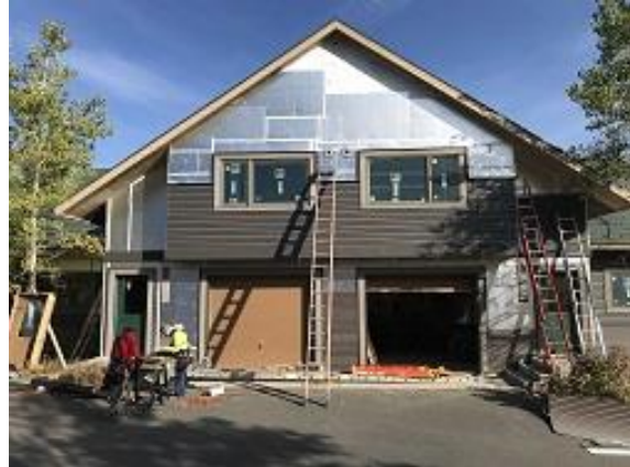
Building F1 Units 16 & 17 Front Lap Siding Installed
