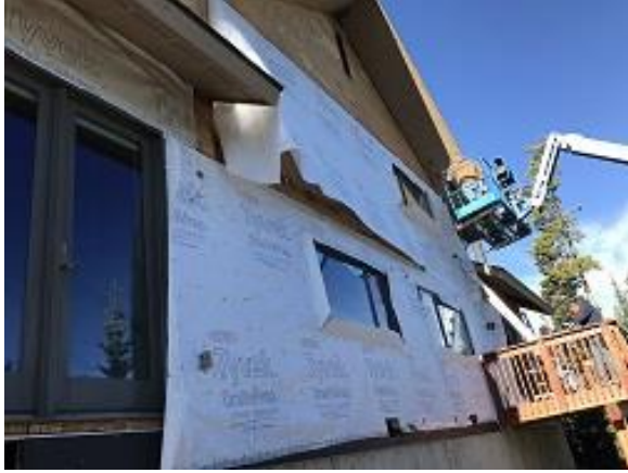
Building E7 Units 51 & 52 Back Tyvek Installed
