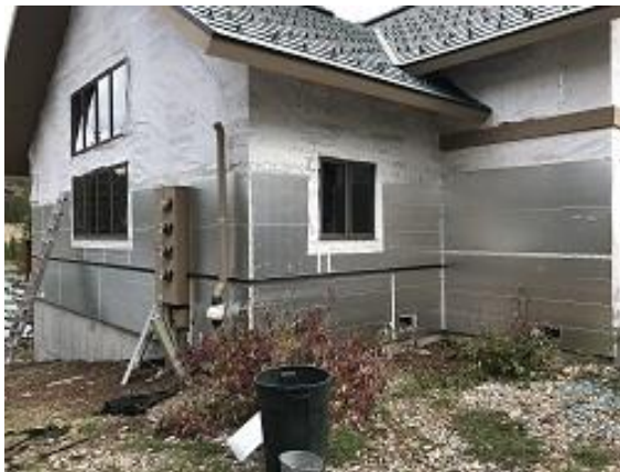
Building E7 Unit 52 Side Wainscot Flashing & Foam Board Installed
