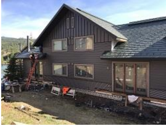
Building E2 Units 20 & 21 Back Board and Batten Siding Installed
