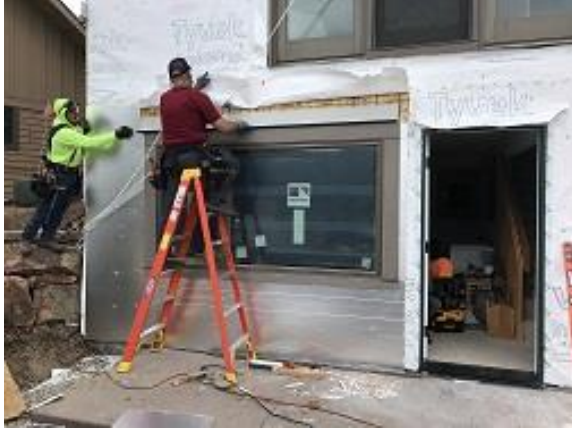
Building F1 Unit 16 Back Window Trim & Foam Board Installed
