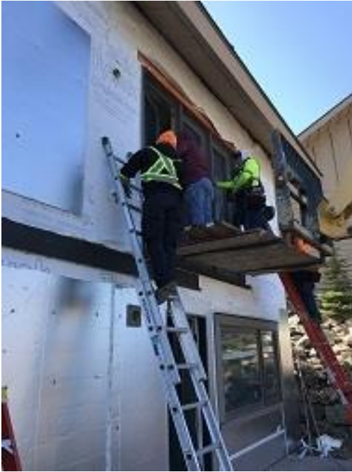
Building F1 Unit 17 Deck Door Installed
