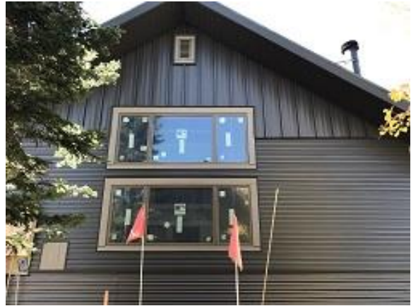
Building F1 Unit 16 Side Board and Batten Siding Installed
