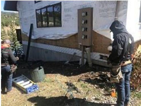
Building E7 Unit 52 Side Base Flashing Tape Installed
