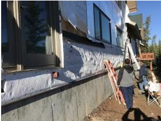
Building E7 Unit 49 Back Wainscot Flashing Installed
