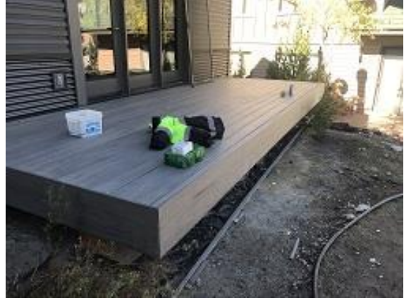
Building E3 Unit 24 Decking Completed
