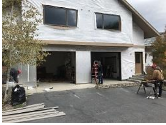
Building E7 Units 49 & 50 Front Garage Door Metal & Foam Board Installed
