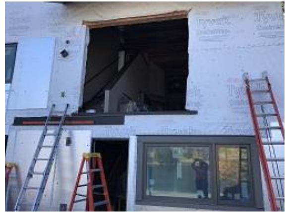
Building F1 Unit 17 Deck Door Flashing Installed
