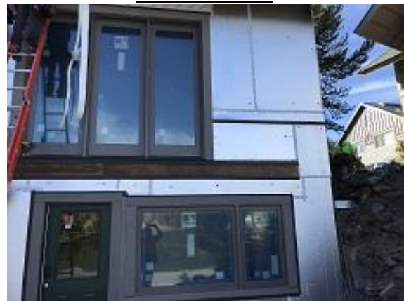
Building F1 Unit 17 Back Wainscot Flashing and J Channel Installed
