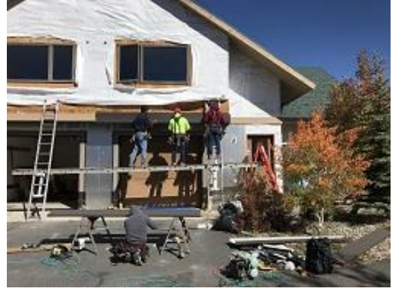
Building E7 Units 49 & 50 Front Belly Band Installed
