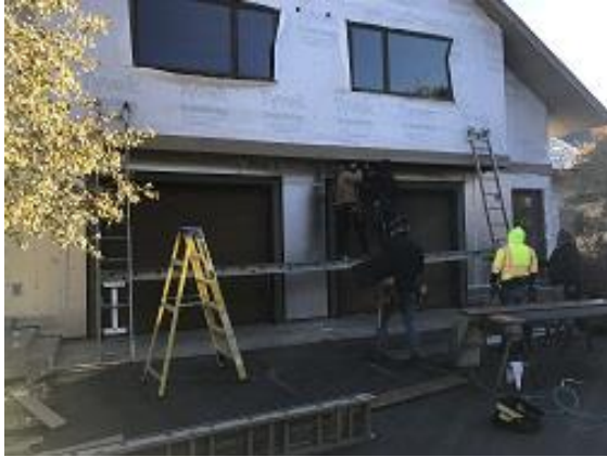
Building E7 Units 49 & 50 Front Soffit Installed
