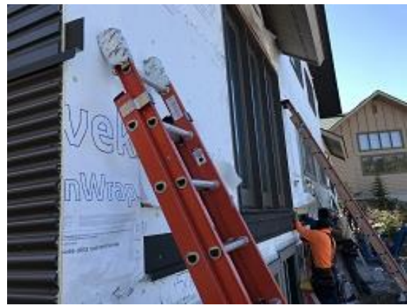
Building F1 Unit 16 Back Deck Door and Ledger Flashing Installed
