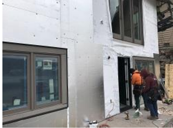
Building F1 Unit 17 Back Window Trim & Foam Board Installed
