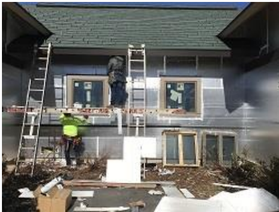
Building E7 Units 50 & 51 Front Kitchen Windows, Trim & Foam Board Installed
