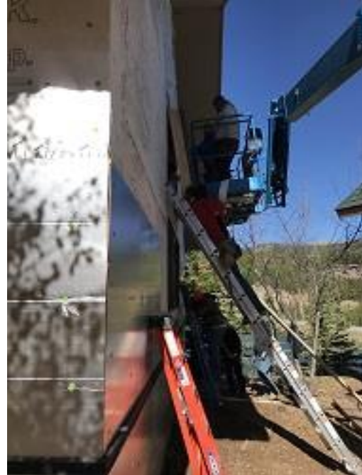
Building E7 Unit 49 Side Windows Installed
