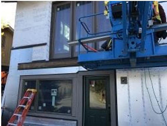
Building F1 Units 16 & 17 Back Wainscot Flashing and J Channel Installed
