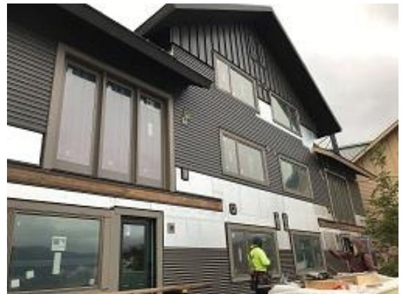
Building F1 Units 16 & 17 Back Lap & Corrugated Siding Installed
