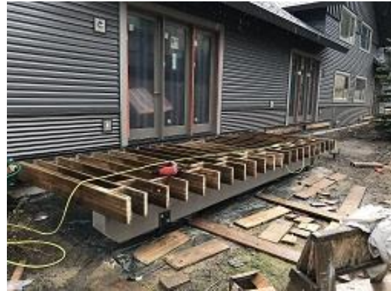
Building E2 Unit 21 Deck Framing Installed
