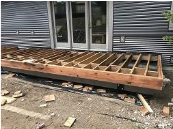
Building E4 Unit 30 Deck Framing Completed
