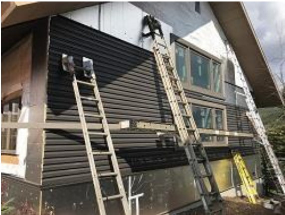
Building E7 Unit 49 Side Lap Siding Installed
