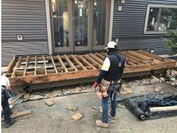
Building E4 Unit 28 Deck Framing Completed
