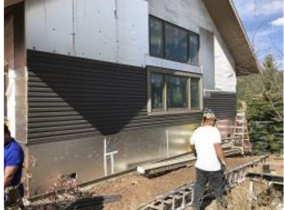
Building E7 Unit 49 Lap Siding Installed
