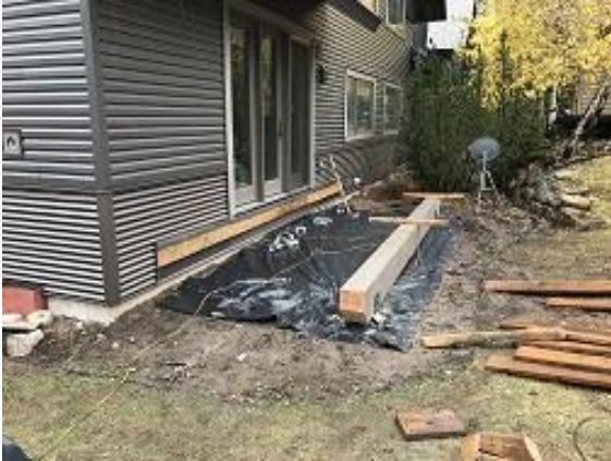
Building E1 Unit 11 Deck Framing Began
