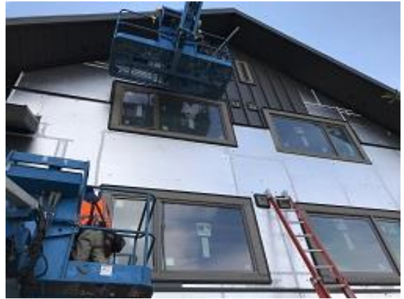
Building F1 Units 16 & 17 Board and Batten Siding Installed
