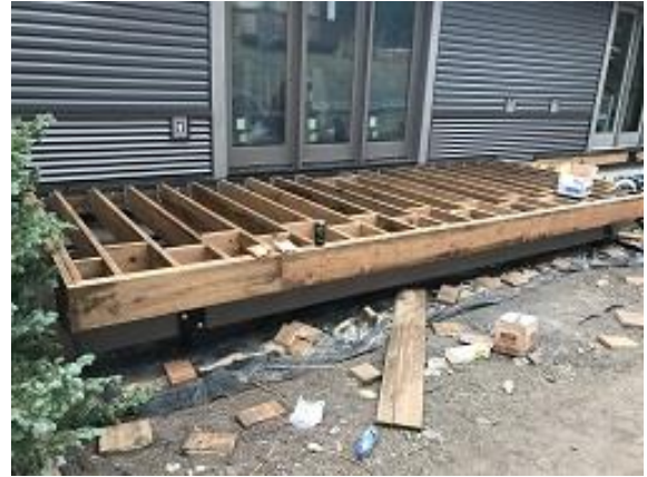
Building E4 Unit 29 Deck Framing Completed
