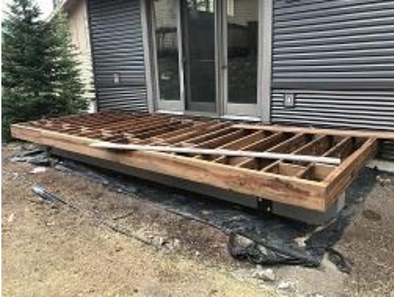
Building E2 Unit 20 Deck Framing Completed
