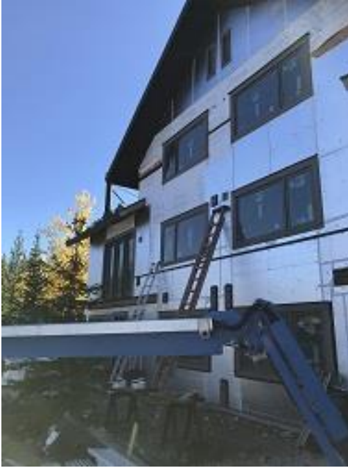
Building F1 Unit 16 & 17 J Channel, Blocking Installed
