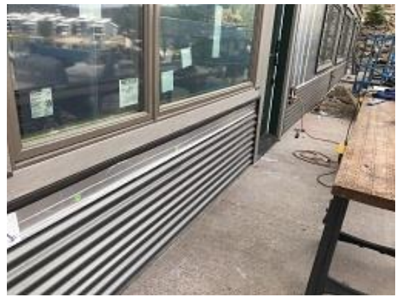
Building F1 Unit 16 Back Corrugated Siding Installed
