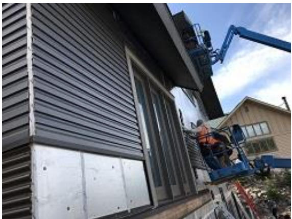
Building F1 Unit 16 Lap Siding Installed
