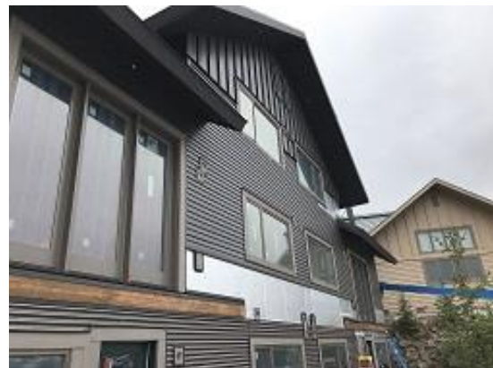
Building F1 Units 16 & 17 Lap and Corrugated Siding Installed
