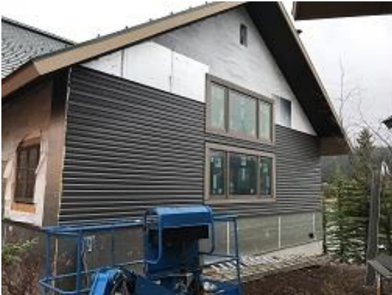
Building E7 Unit 49 Side Lap Siding Installed
