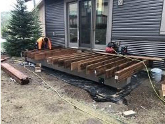
Building E2 Unit 20 Deck Framing
