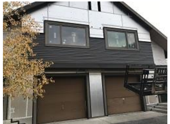
Building E7 Units 49 & 50 Front Lap Siding Installed
