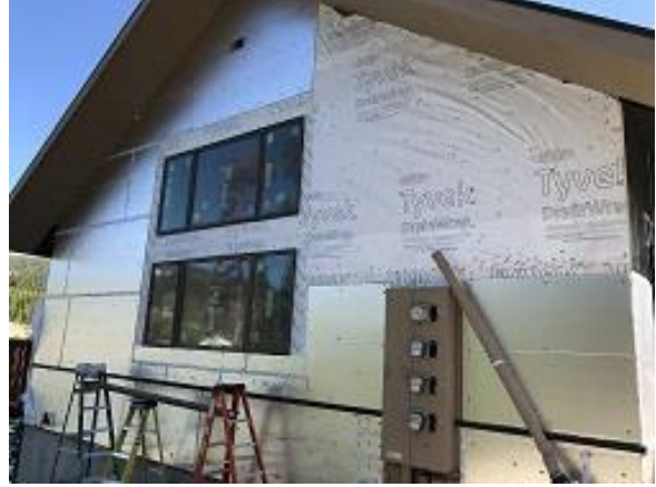
Building E7 Unit 52 Side Foam Board Installed
