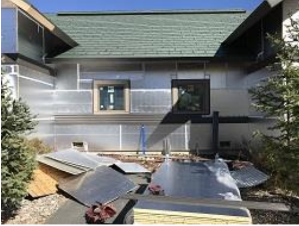
Building E7 Units 50 & 51 Front Lap Siding Installed
