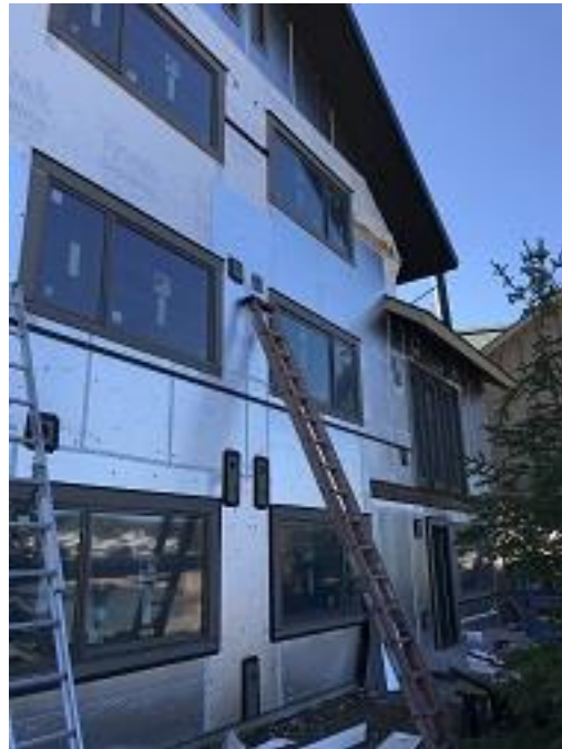
Building F1 Unit 16 & 17 J Channel Blocking Installed
