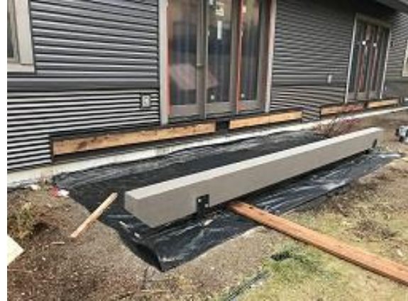
Building E2 Unit 21 Deck Framing Began
