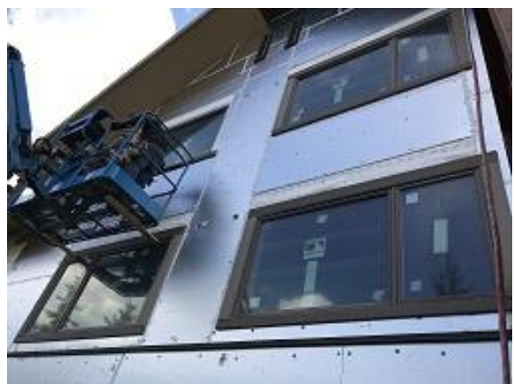
Building E7 Units 51 & 52 Window Trim Installed
