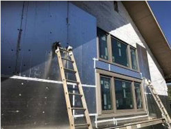
Building E7 Unit 49 Side Foam Board Installed
