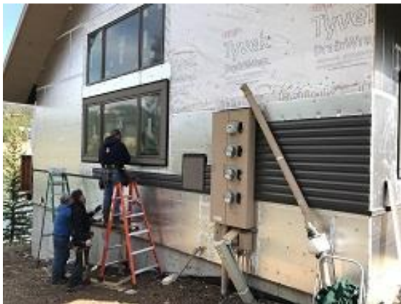
Building E7 Unit 52 Lap Siding Installed
