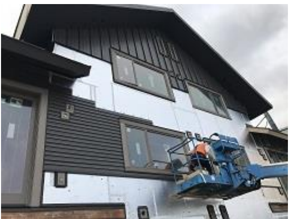
Building F1 Units 16 & 17 Back Lap Siding Installed
