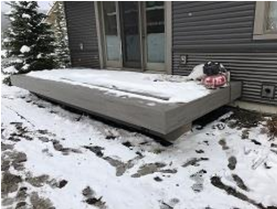
Building E2 Unit 20 Decking Installation Completed
