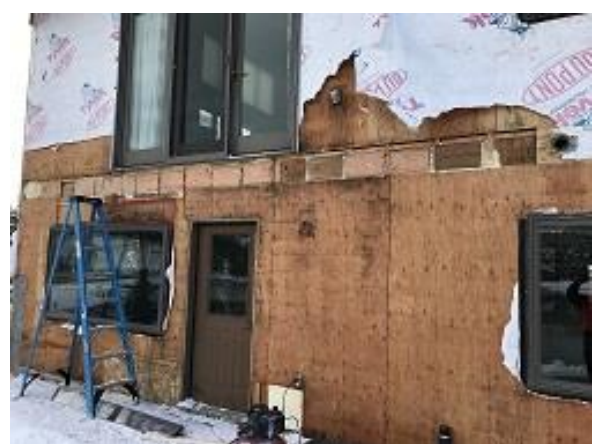
Building F2 Unit 18 Deck Ledger Blocking Installation
