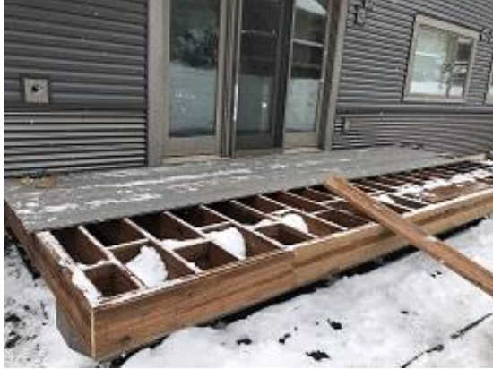
Building E2 Unit 20 Decking Installation Continued
