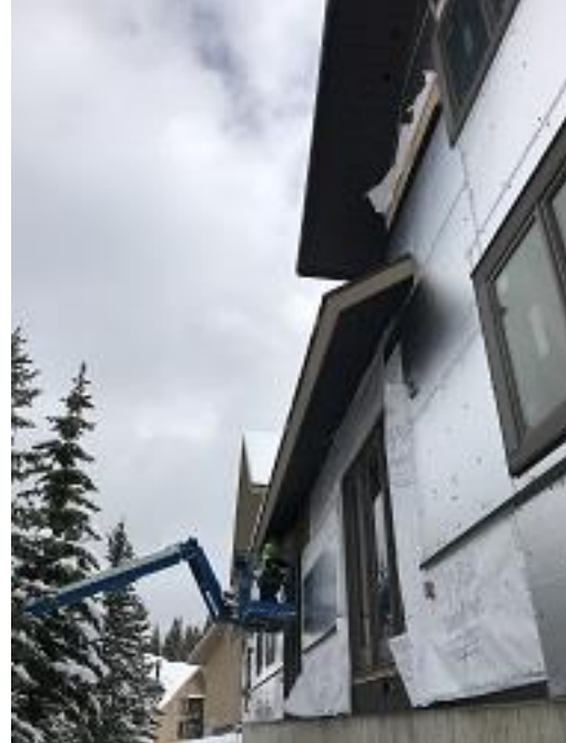
Building E7 Units 50 & 51 Back Fascia & Soffit Installation Continued
