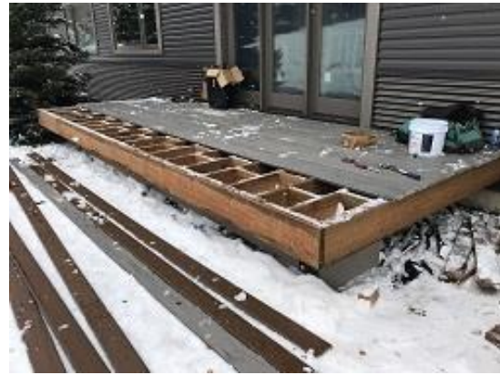
Building E4 Unit 29 Decking Installation Continued
