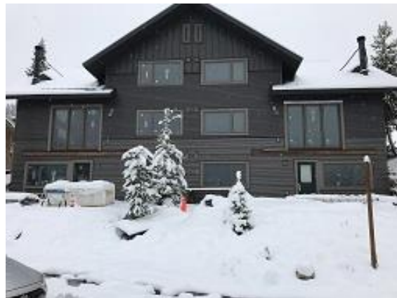
Building F1 Units 16 & 17 Back Siding Completed
