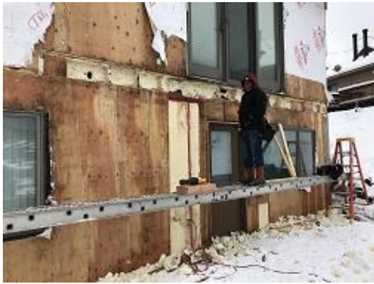
Building F2 Unit 19 Deck Ledger Blocking Installation
