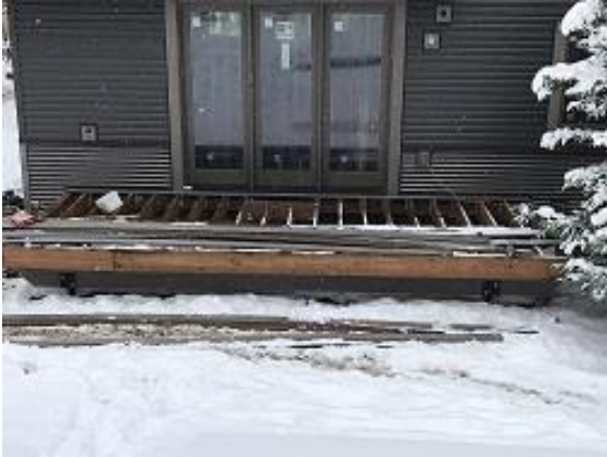
Building E4 Unit 28 Deck Railing Blocking and Decking Installation Began
