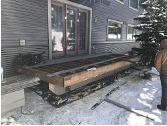
Building E2 Unit 22 Decking Installation Began
