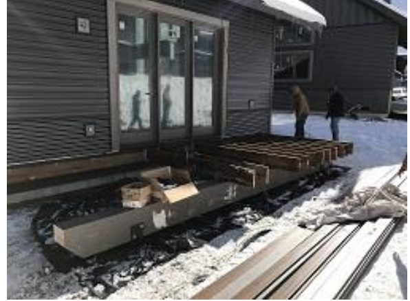
Building E2 Unit 23 Deck Framing Began
