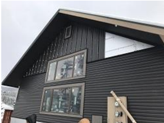
Building E7 Unit 52 Board and Batten Siding Installed
