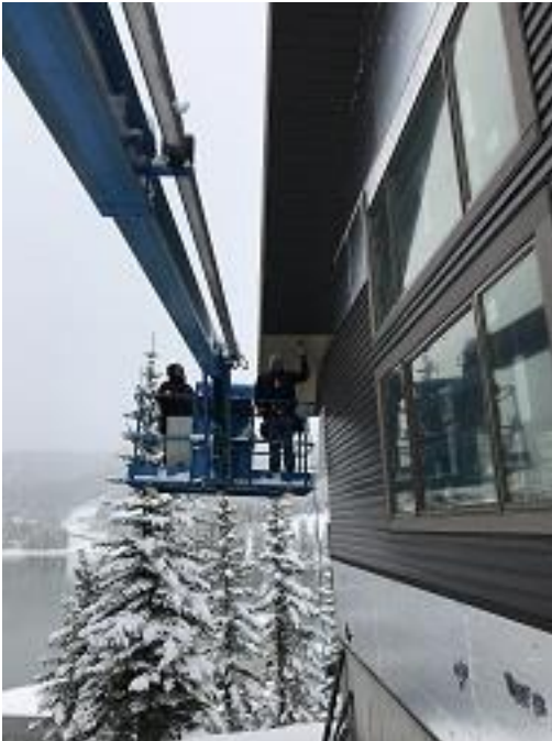
Building E7 Unit 52 Side Soffit Installed
