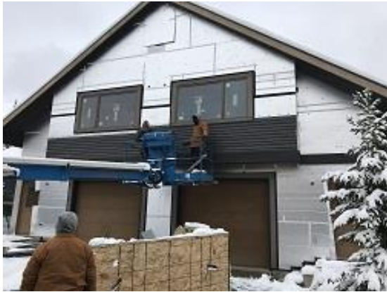
Building E7 Units 51 & 52 Lap Siding Installed
