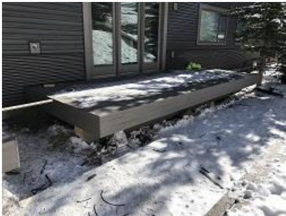
Building E4 Unit 30 Decking Completed
