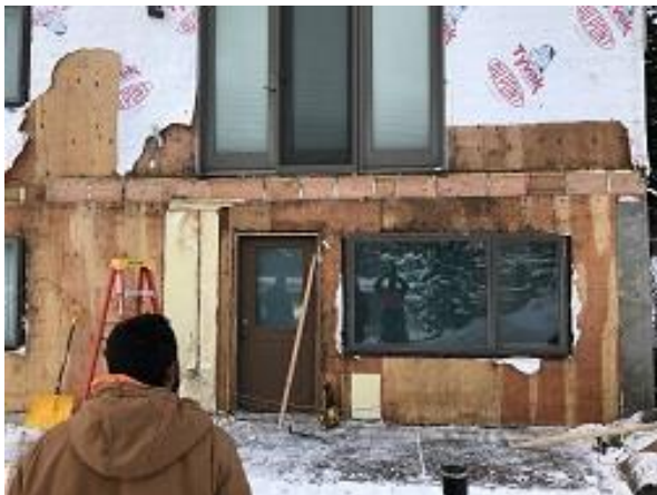
Building F2 Unit 19 Deck Ledger Blocking Installation
