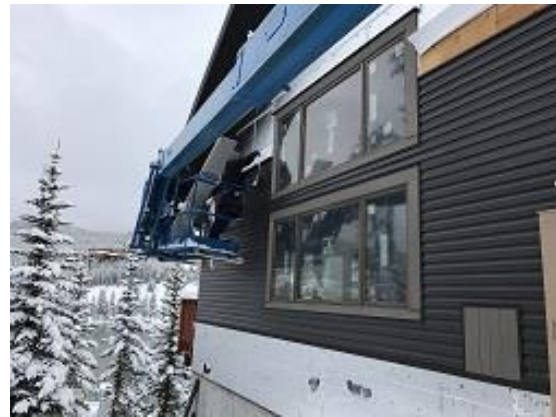
Building E7 Unit 52 Side J Channel Installed
