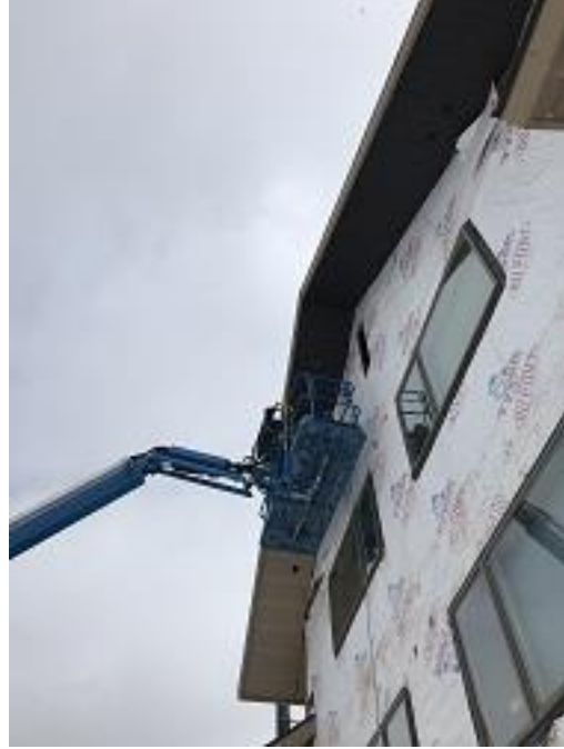
Building F2 Units 18 & 19 Fascia & Soffit Installation
