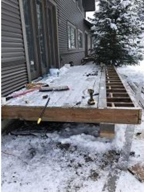
Building E4 Unit 28 Decking Installation Continuing
