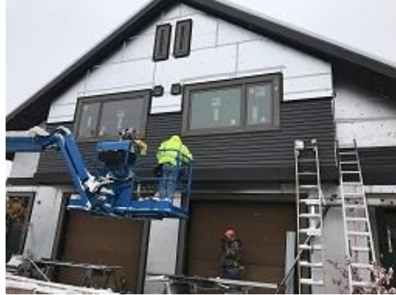
Building E7 Units 49 - 50 Board and Batten Siding Installation Began
