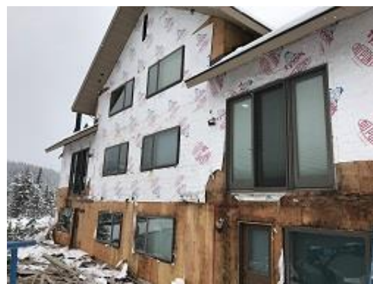
Building F2 Units 18 & 19 Siding Demo Progress
