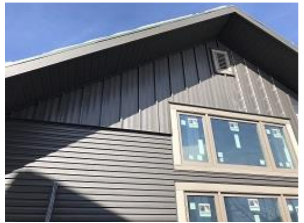
Building E7 Unit 49 Side Board and Batten Siding Installation
