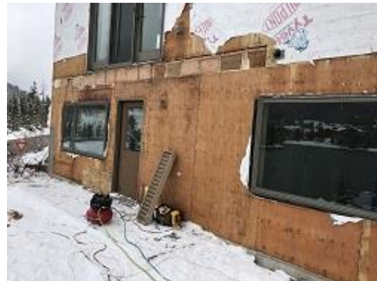
Building F2 Unit 18 Deck Ledger Blocking Installation
