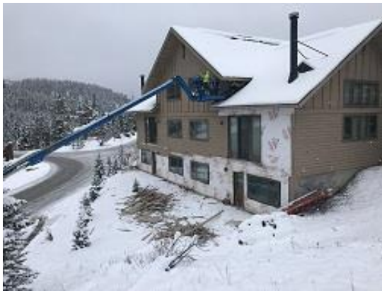
Building F2 Units 18 & 19 Siding Demo Began
