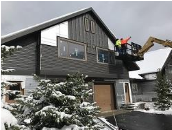
Building E7 Units 51 & 52 Front Board and Batten Siding Installation
