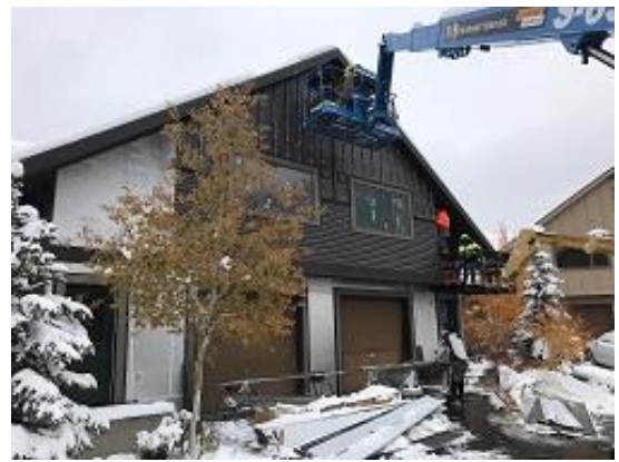
Building E7 Units 49 & 50 Board and Batten Siding Installed
