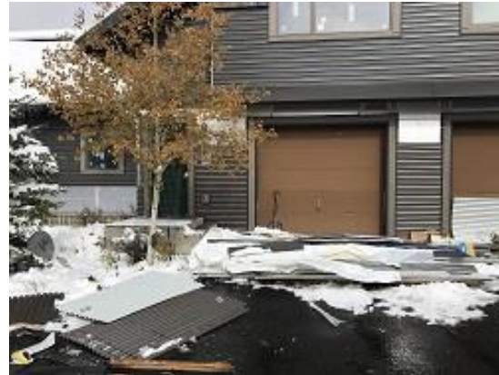
Building E7 Units 49 & 50 Corrugated Siding Installed
