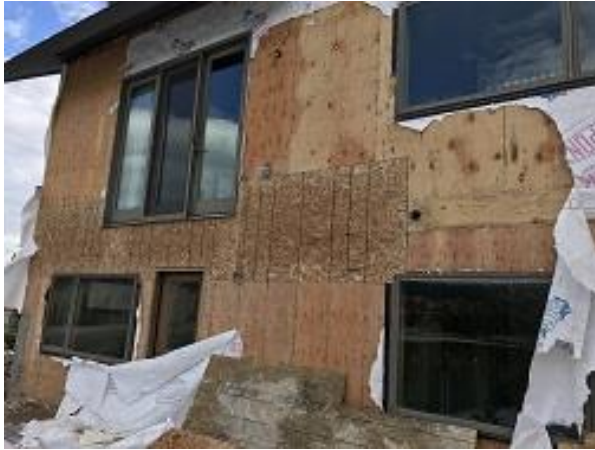
Building F2 Unit 18 Back Deck Sheathing Installation
