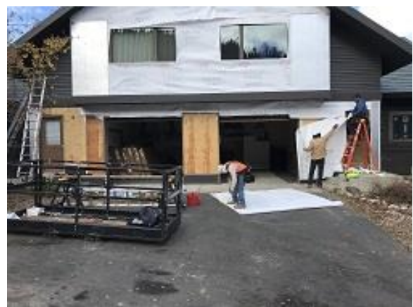
Building F2 Units 18 & 19 Tyvek Installation
