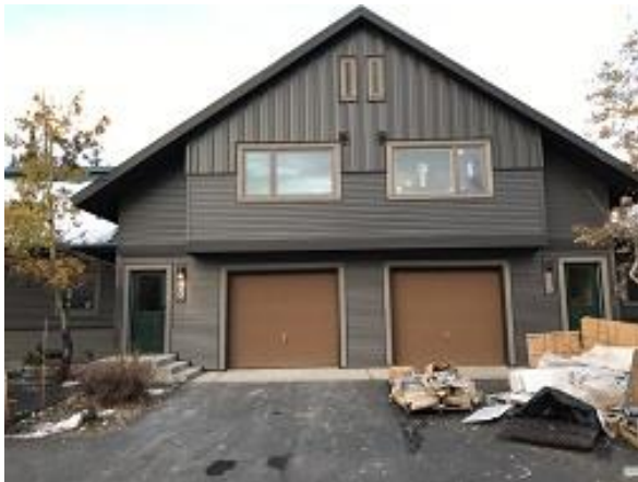
Building E4 Units 28 & 29 Addresses Applied
