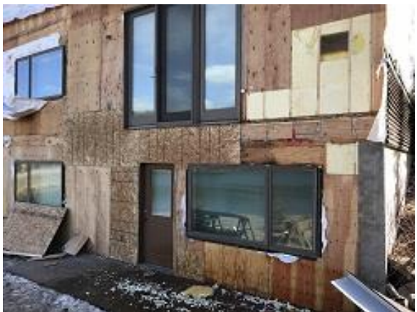
Building F2 Unit 19 Deck Blocking Sheathing Installation
