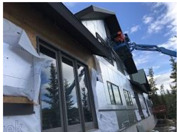
Building E7 Units 49 & 50 Back Board and Batten Siding Installation
