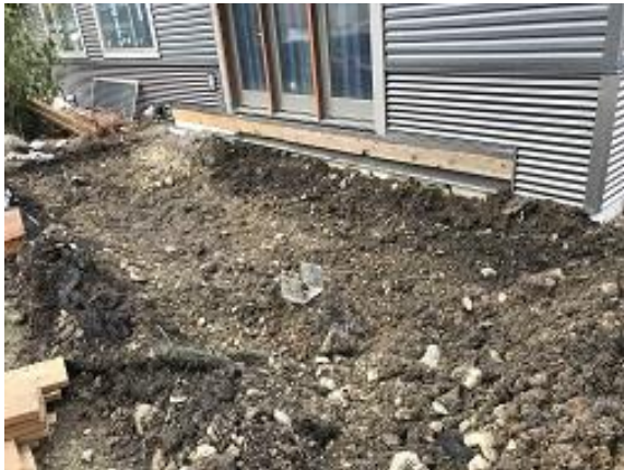
Building E1 Unit 8 Deck Area Grading
