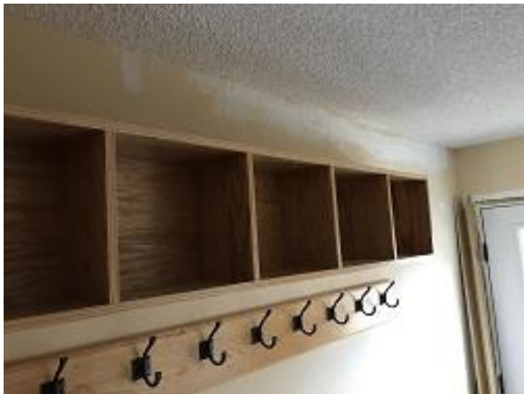
Building E4 Unit 28 Entry Interior Drywall Repair Progressing
