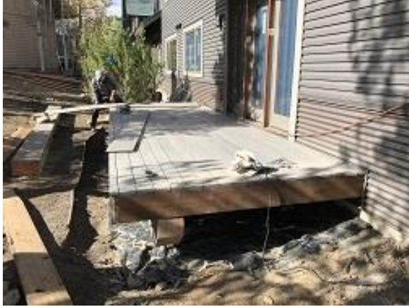
Building E1 Unit 8 Decking Installation
