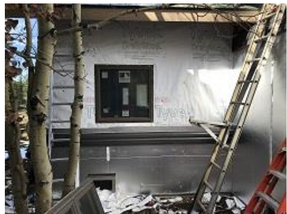
Building F2 Unit 19 Kitchen Window, Wainscot Flashing & Foam Insulation Installation
