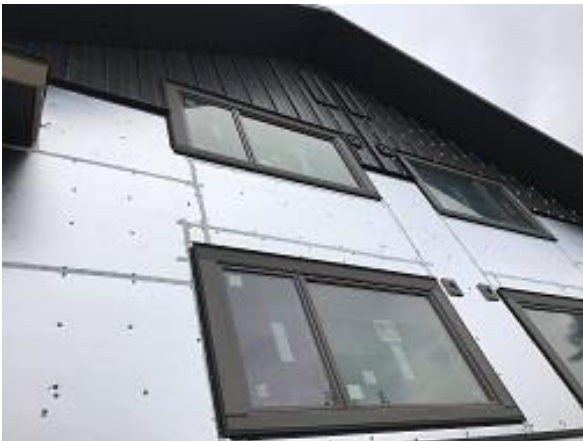
Building E7 Units 51 & 52 Back Board and Batten Installation
