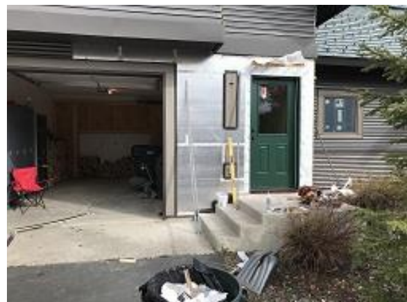
Building E7 Unit 51 Front Door Installation
