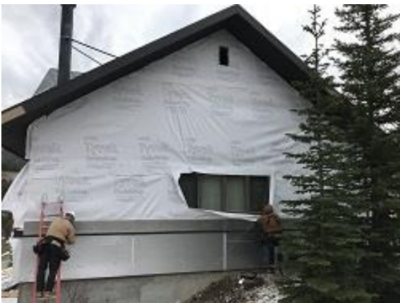
Building F2 Unit 19 Side Base & Wainscot Flash Installation
