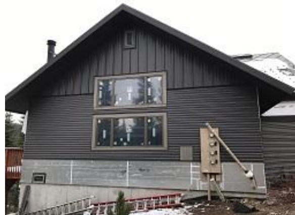
Building E7 Unit 52 Side Siding Installation
