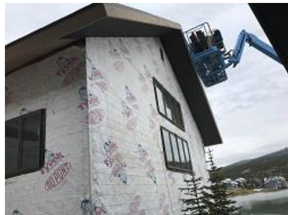
Building F2 Unit 18 Side Fascia & Soffit Installation
