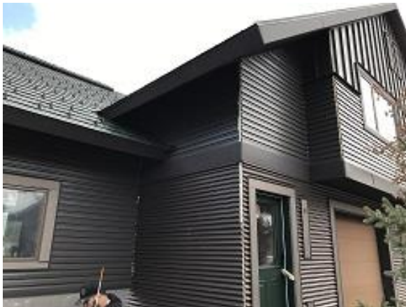
Building E7 Unit 50 Side Lap Siding & Diverter Installation
