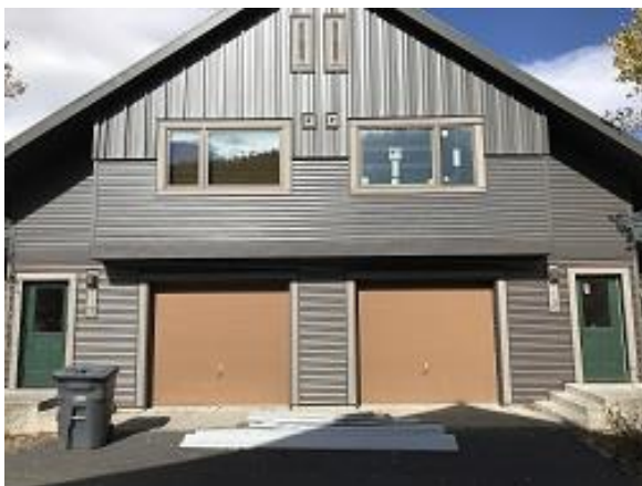
Building F1 Units 16 & 17 Addresses and Lighting Installation
