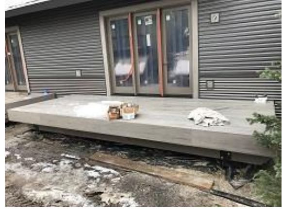
Building E2 Unit 22 Deck Complete
