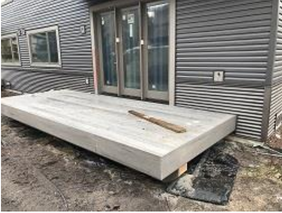
Building E2 Unit 23 Deck Complete
