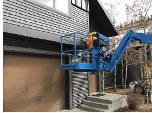
Building E3 Unit 25 Front Caulking Applied
