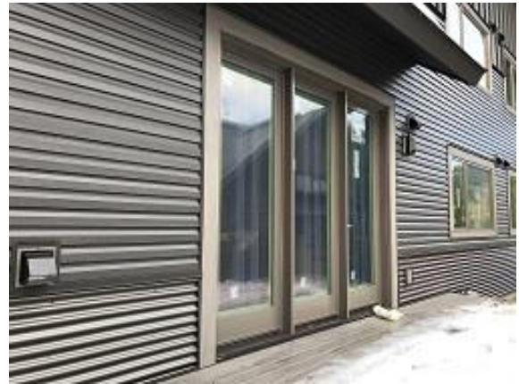
Building E3 Unit 24 Back Vents Installed
