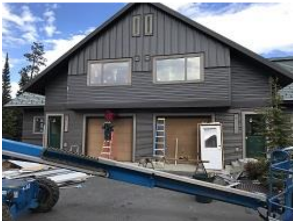
Building E7 Units 51 & 52 Front Corrugated Siding Installation
