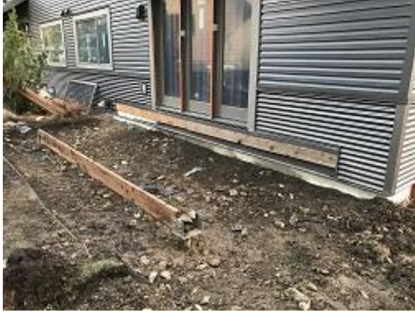
Building E1 Unit 8 Deck Grading Completed
