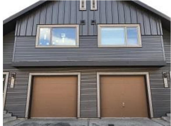
Building E1 Units 8 & 9 Addresses Applied
