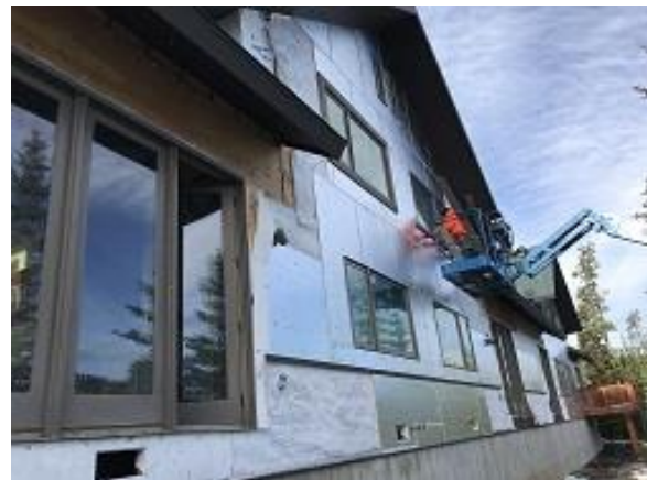
Building E7 Units 49 & 50 Back Window Trim Installation
