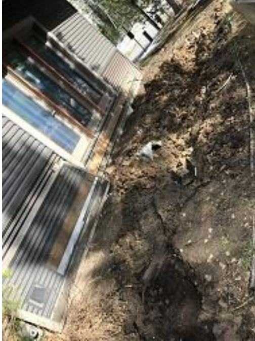
Building E1 Unit 8 Deck Area Grading
