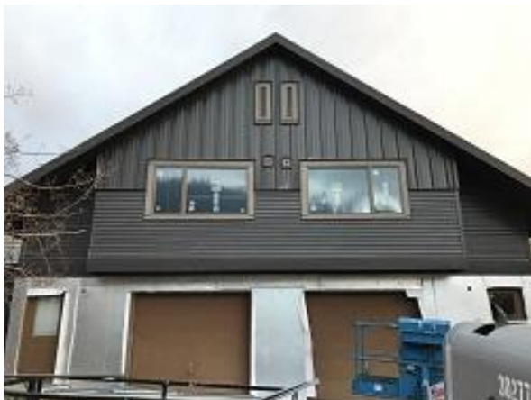
Building F2 Units 18 & 19 Board and Batten Install
