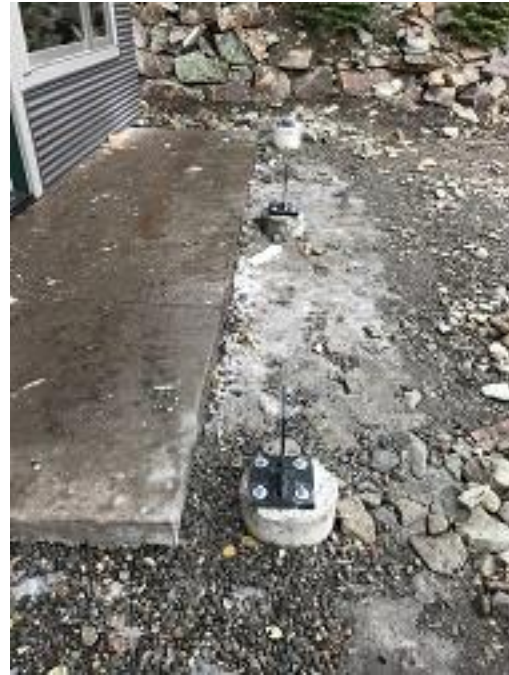
Building F1 Unit 17 Deck Knife Plates Install
