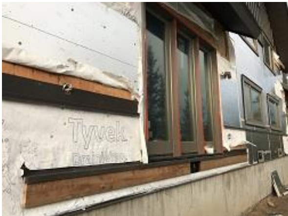
Building E7 Unit 49 Deck Door Installed
