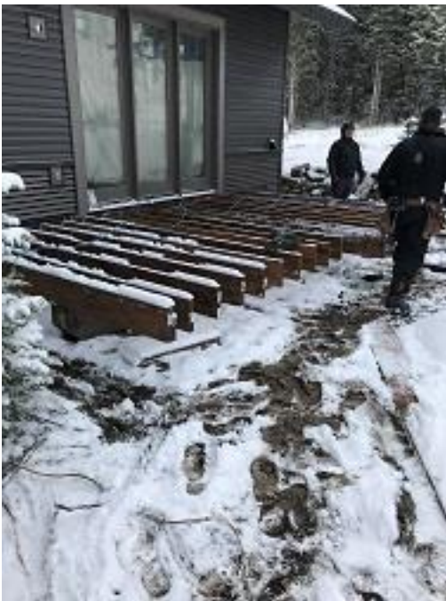
Building E41 Unit 31 Deck Framing
