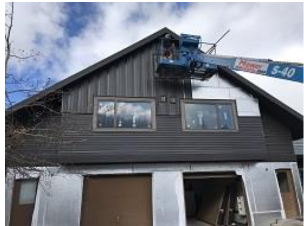
Building F2 Units 18 & 19 Front Board and Batten Siding Installation
