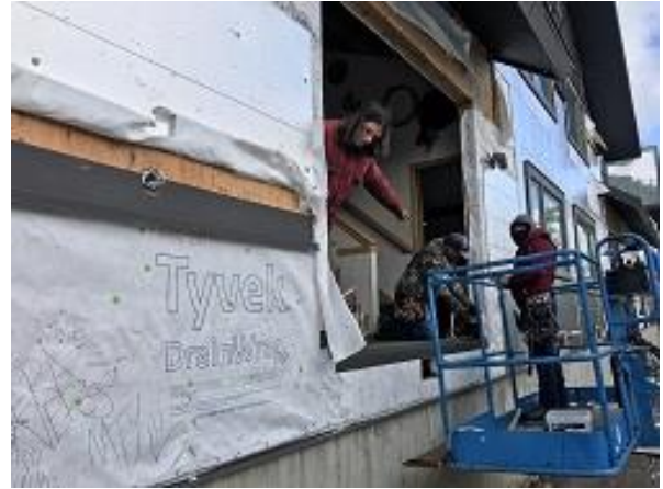
Building E7 Unit 49 Deck Door Installation
