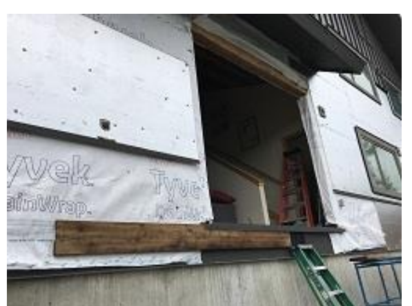
Building E7 Unit 51 Deck Door Installation
