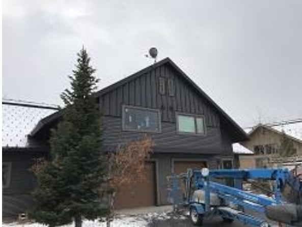
Building E1 Units 10 & 11 Satellite Dishes Installation
