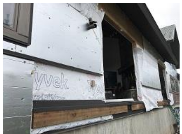
Building E7 Unit 50 Deck Door Installation
