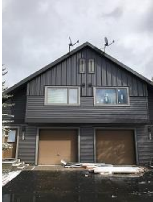
Building E3 Units 26 & 27 Satellite Dish Installation
