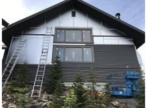
Building F2 Unit 18 Side Lap Siding Installation
