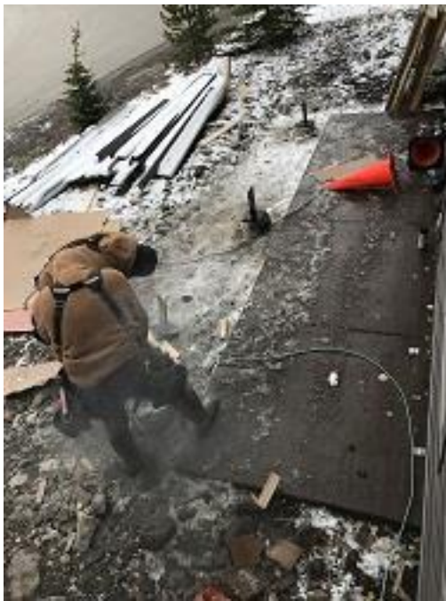
Building F1 Unit 17 Deck Knife Plates Installation
