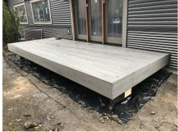
Building E1 Unit 08 Decking Installation
