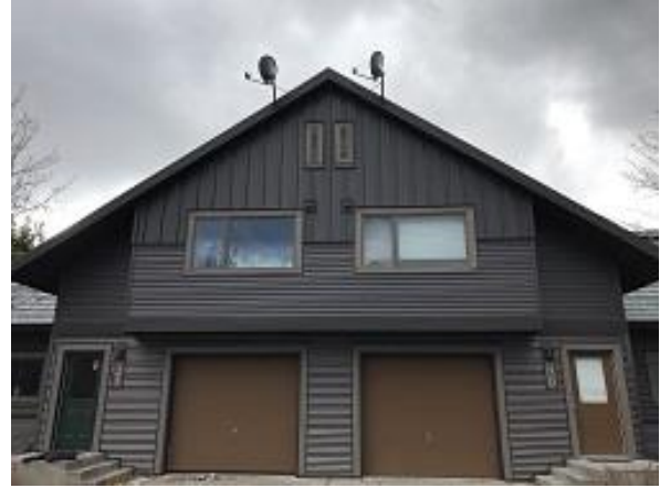
Building E4 Units 30 & 31 Satellite Dishes Installed
