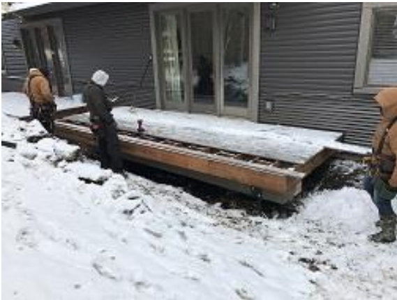
Building E1 Unit 09 Decking Installation
