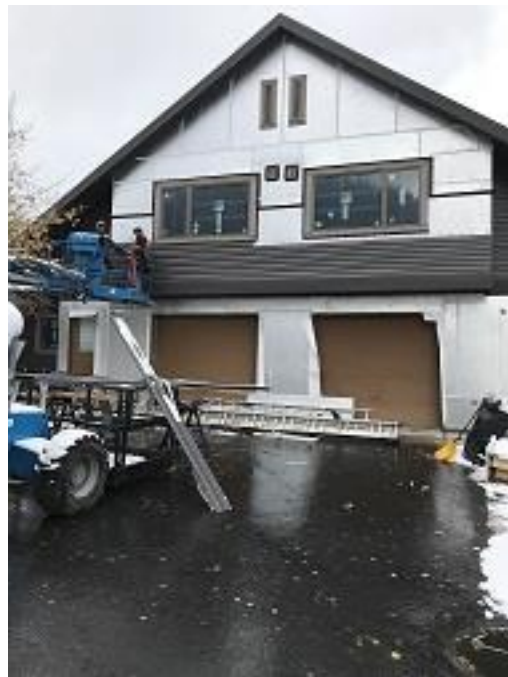
Building F2 Units 18 & 19 Front Lap Siding Installation
