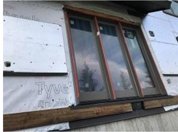
Building E7 Unit 51 Deck Door Installed
