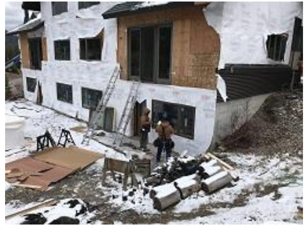
Building F2 Unit 19 Back Window Installation
