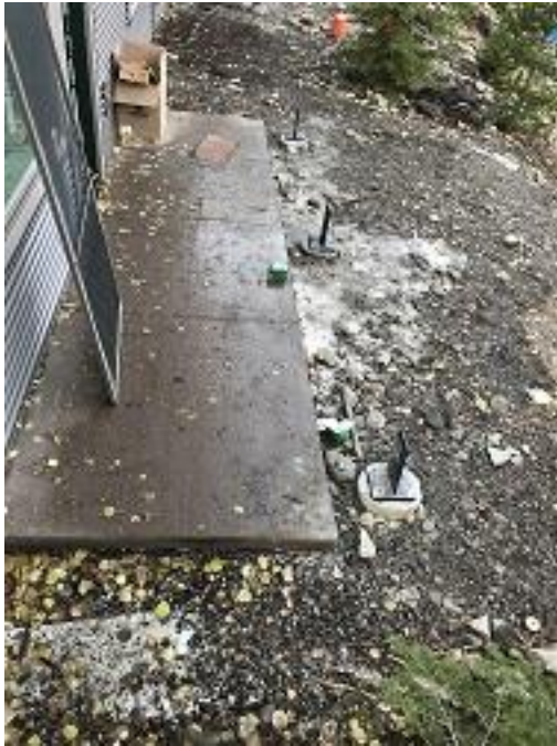
Building F1 Unit 16 Deck Knife Plates Installed
