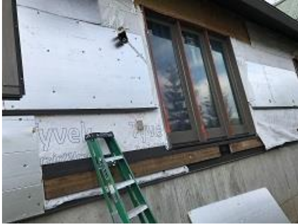
Building E7 Unit 50 Deck Door Installed
