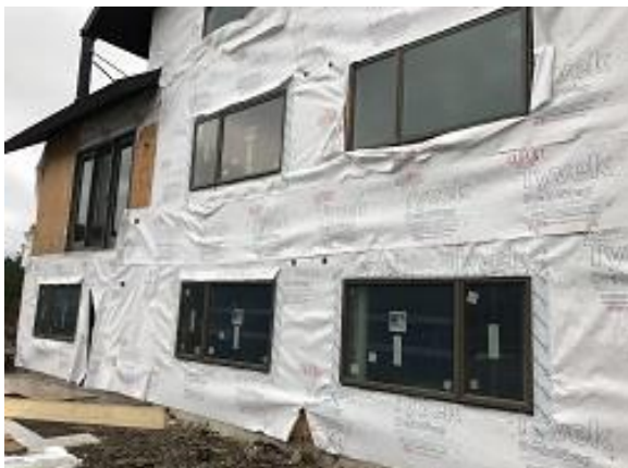
Building F2 Units 18 & 19 Back Window Install
