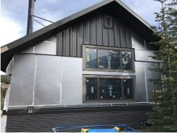
Building F2 Unit 19 Side Board and Batten Siding Installation
