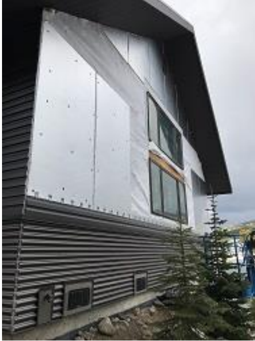
Building F2 Unit 18 Side Windows Install
