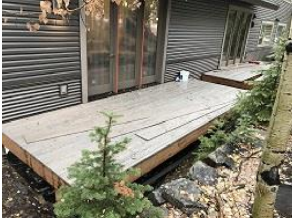
Building E1 Unit 10 Decking Installation
