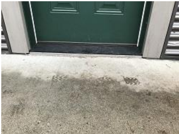
Building E2 Unit 23 Threshold Support Install
