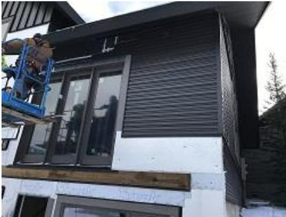
**Building F2 Unit 19 Back Lap Siding Install**
