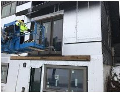
Building F2 Unit 19 Back Wainscot Flashing Installed
