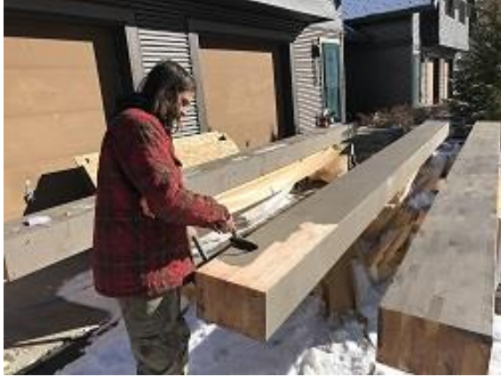
Building E7 Unit 50 GLULAM Painting
