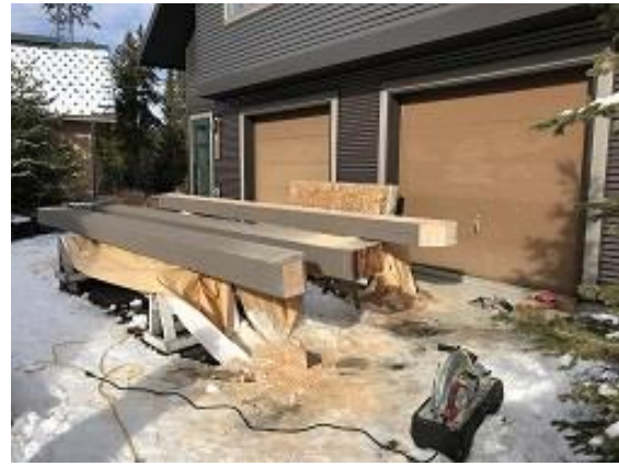
Building E7 Units 49 & 50 GLULAM Preparation
