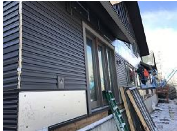
Building E7 Unit 49 Back Lap Siding Install
