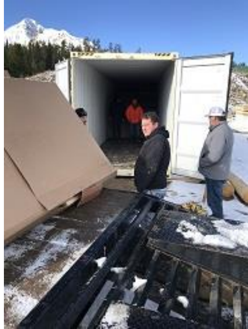
Windows Removed From Garages and Loaded Into Conex For Storage
