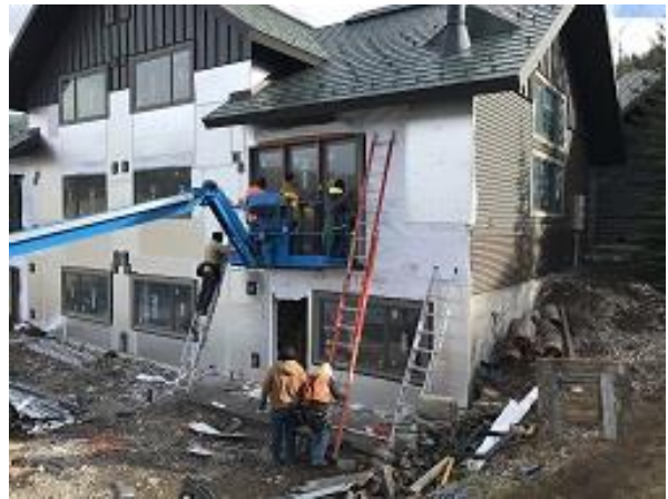
Building F2 Unit 19 Back Deck and Lower Door Installation
