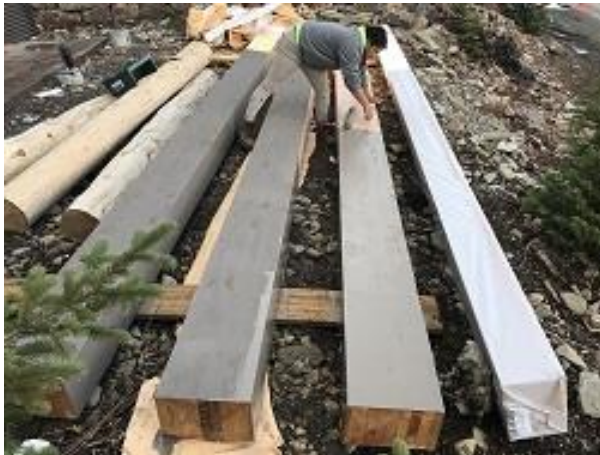
Building F1 & F2 Units 16 - 19 Deck GLULAM's Painted
