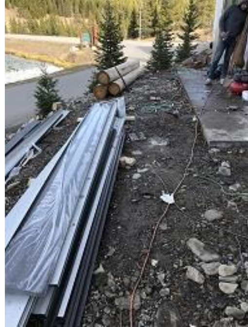
Building F2 Unit 18 Deck Knife Plates Installation
