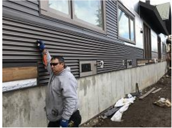
Building E7 Units 49 & 50 Back Corrugated Siding Installation
