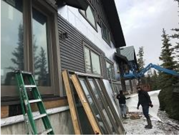
Building E7 Units 49 & 50 Back Lap Siding Installation
