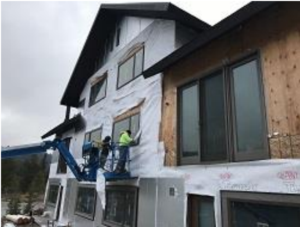
Building F2 Units 18 & 19 Back Windows Installation
