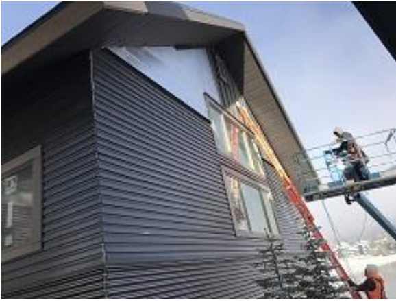
Building F2 Unit 18 Side Board and Batten Installation
