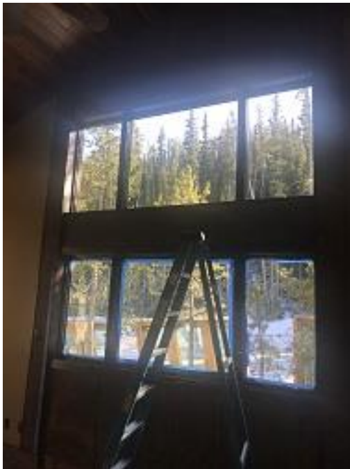
Building E3 Unit 27 Living Room Trim Installed and Finished
