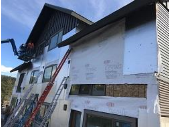
Building F2 Units 18 & 19 Back Board and Batten Siding Installation
