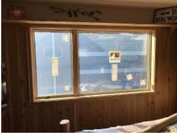
Building E3 Unit 27 Front Upper Interior Trim Installation and Finishing
