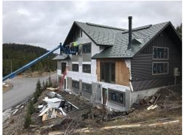
Building F2 Units 18 & 19 Back Window Trim Installation
