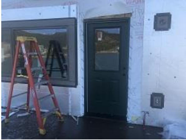
Building F2 Unit 18 Back Lower Door Installed
