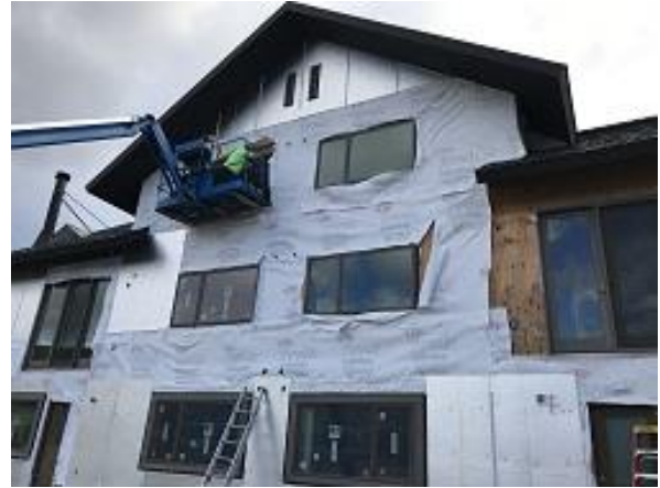
Building F2 Unit 18 Back Upper Window Install
