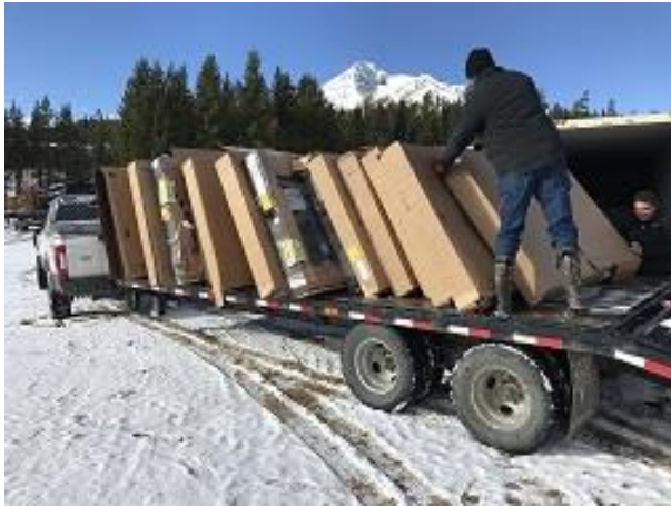
Windows Removed From Garages and Loaded Into Conex For Storage
