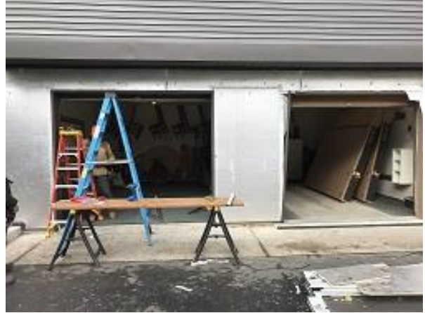
Building F2 Units 18 & 19 Garage Door Flashing Installation
