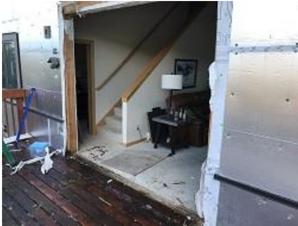
Building E7 Unit 52 Deck Door Installation
