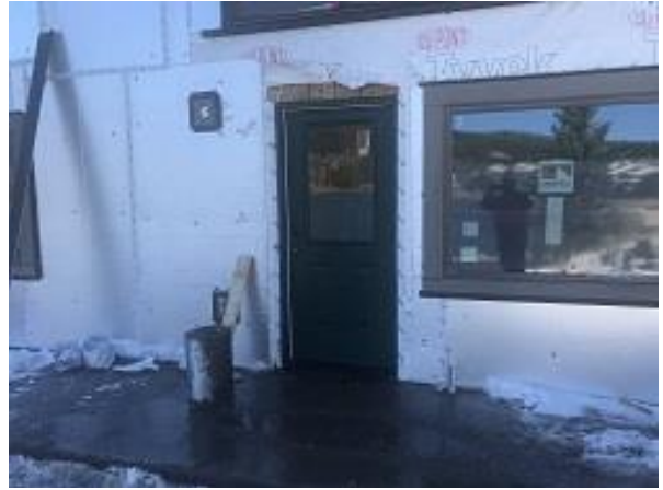
Building F2 Unit 19 Back Lower Door Installed
