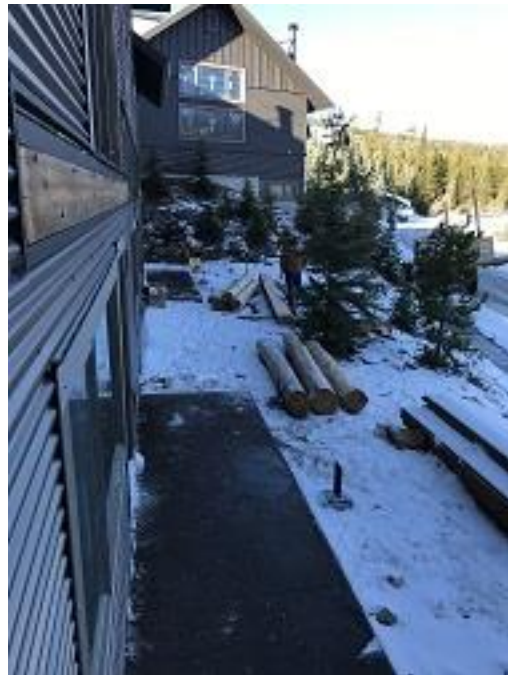
Building F1 & F2 Units 16 - 19 Deck GLULAM's Painted
