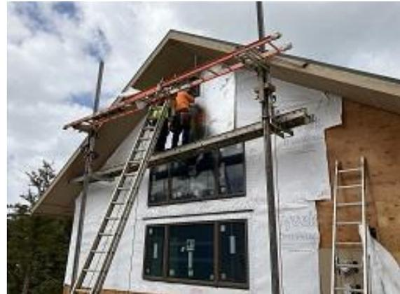
**Building E8 Unit 58 Side Insulation and Gable Vent Installed**
