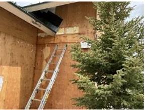
Building E8 Unit 56 Front Sheathing Removed with Moisture Higher Than 10%
