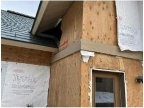
Building E8 Unit 58 Sheathing Removed with Moisture Higher Than 10%
