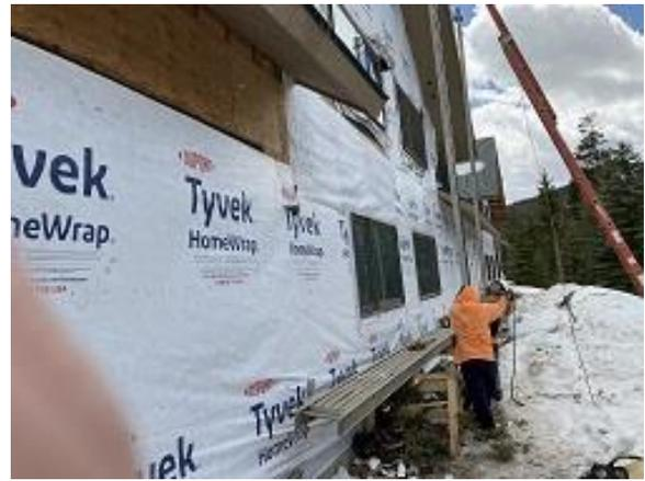
**Building E8 Unit 55 Back Window & Tyvek Installed**
