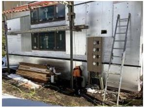
Bldg E8 Unit 58 Side Wainscot, Base Flashing & Insulation Installed
