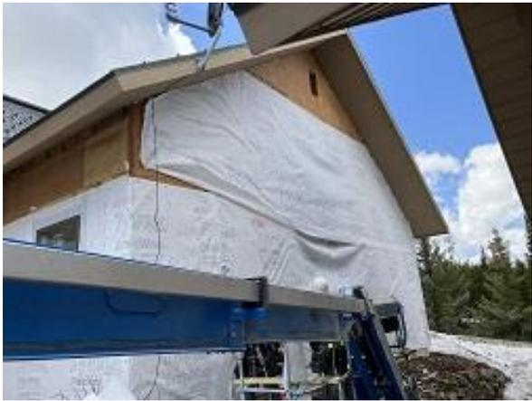
**Building E8 Unit 55 Side Tyvek Installed**
