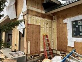
Building E8 Unit 57 Sheathing Removed with Moisture Higher Than 10%
