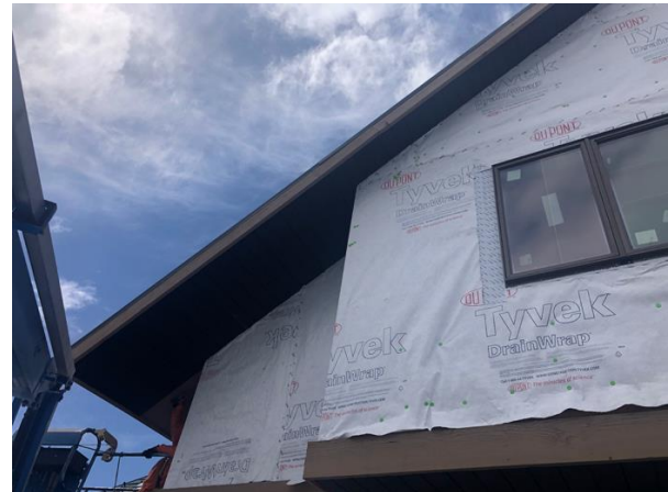
Building E8 Unit #58 Soffit in Progress
