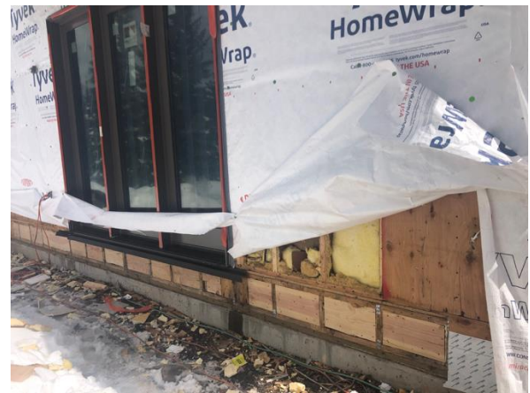
Building E8 Unit #58 Blocking at Deck
