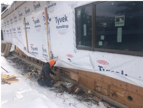
Building E8 Unit #57 Blocking in Progress
