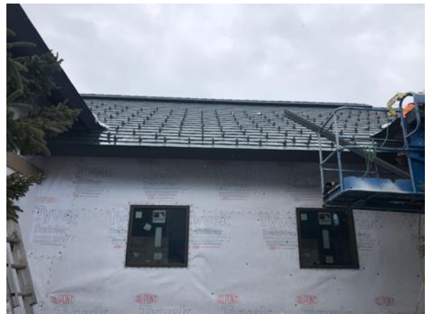
Building E8 Units 57 & 56 Kitchen Windows
