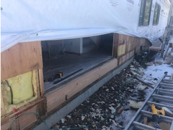
Building E8 Unit #55 Blocking in Progress
