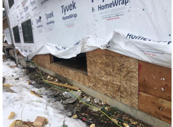
Building E8 Unit #56 Sheathing Complete
