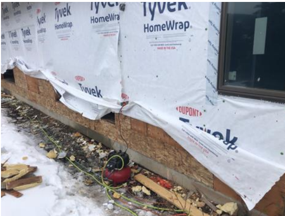
Building E8 Unit #57 Sheathing Complete
