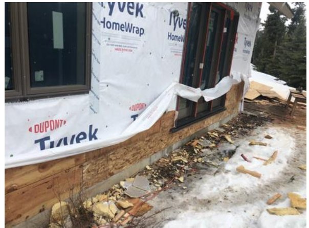
Building E8 Unit #58 Sheathing Complete
