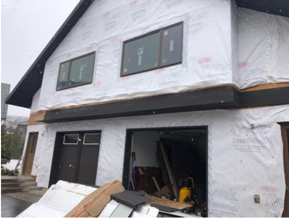
Building E8 Unit 58 & 57 Belly Band
