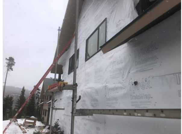
Building E8 Unit 55 Drain Wrap
