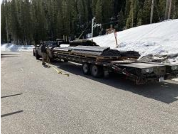
Delivery of Building E6 Siding Materials
