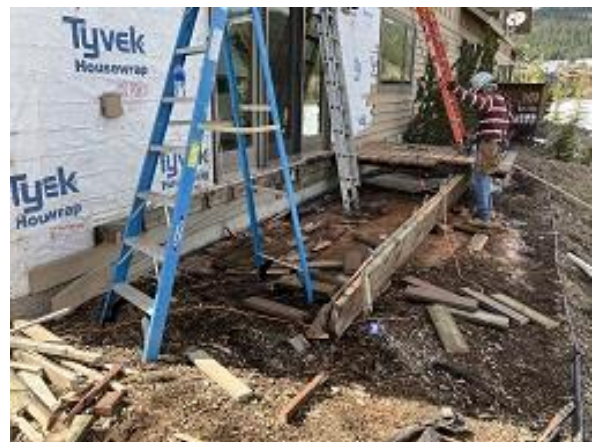
Building E5 Unit 41 Back & Deck Demo
