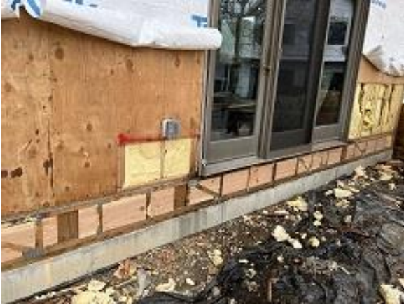
Building E9 Unit 61 Deck Blocking Installed
