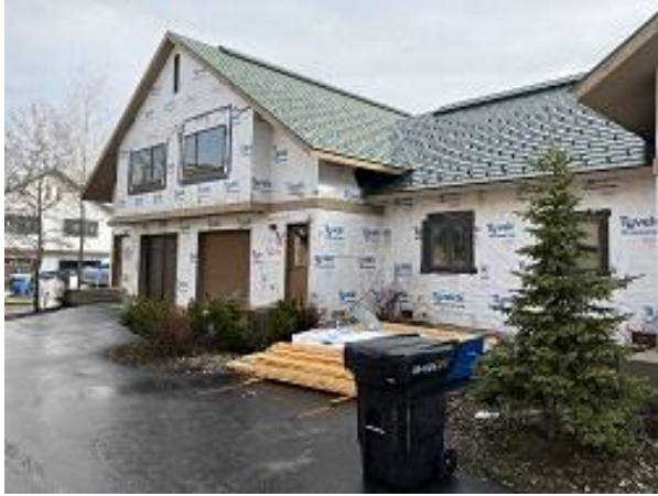
Building E9 Unit 61 & 62 Front Demo Complete
