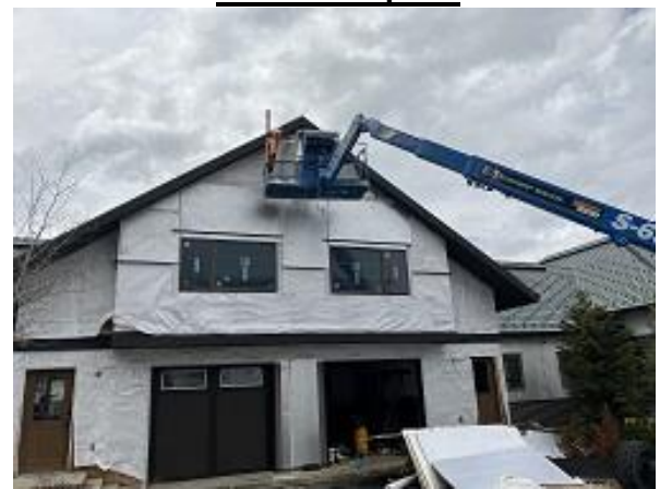
Bldg E8 Units 57 & 58 Front Snap Batten & Window Flashing & Insulation Installed
