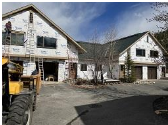
Building E5 Units 41 - 44 Front Siding Demo Completed
