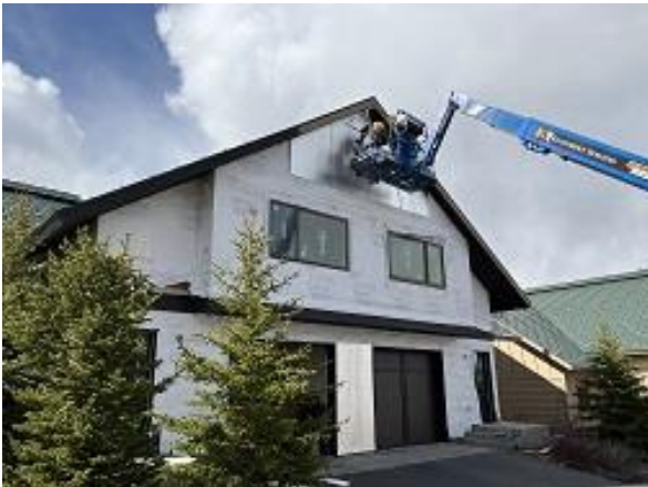
Building E8 Unit 55 & 56 Front Gable Insulation Installed
