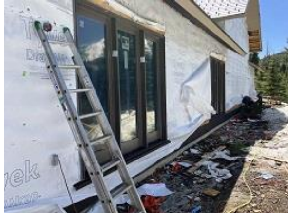
Building E8 Units 56 & 57 Deck Doors Installed
