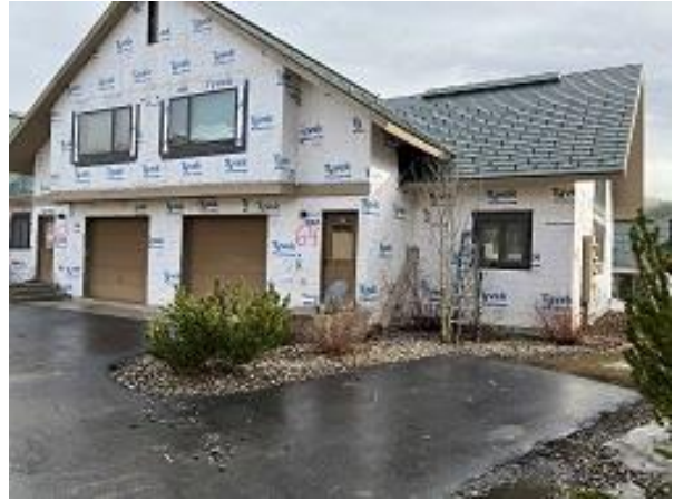
Building E9 Unit 63 & 64 Front Demo Complete
