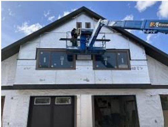
Building E8 Unit 57 & 58 Snap Batten J Channel Installation
