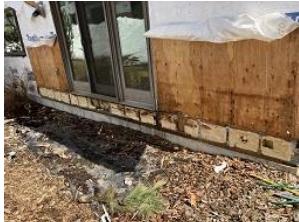
Building E6 Unit 45 Deck Door Substrate
