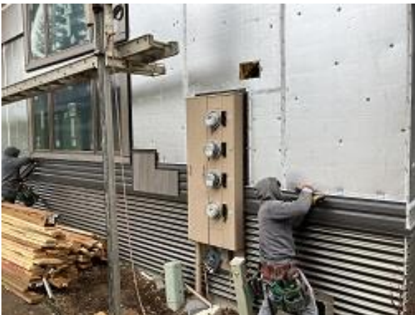
Building E8 Unit 58 Side Lap Siding Installation Began
