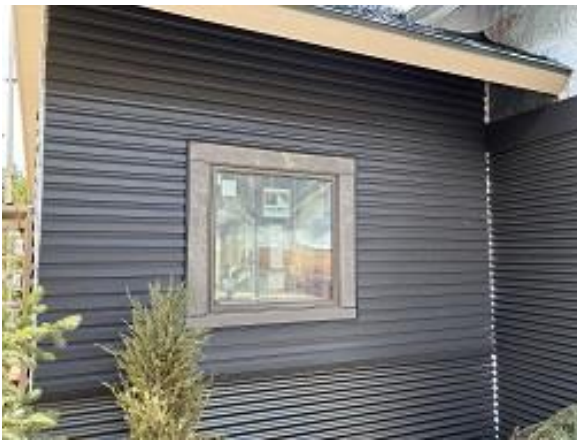
Building E8 Unit 58 Front Lap Siding Installed
