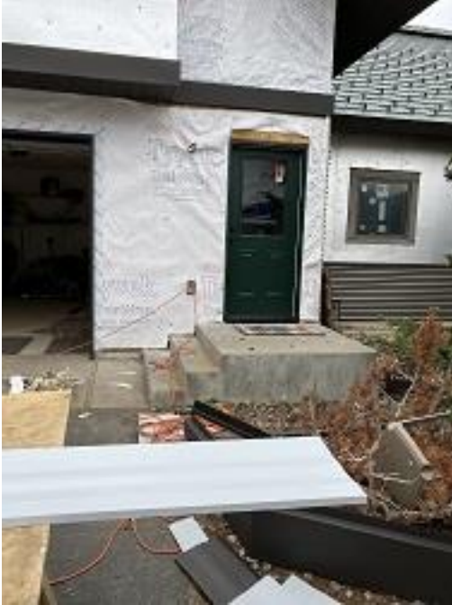
Building E8 Unit 57 Front Door Installed
