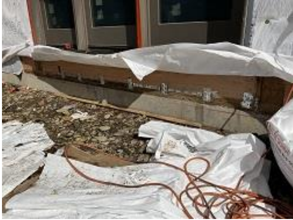
Building E8 Unit 55 Deck Blocking Clips Installed
