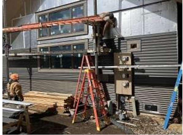
Building E8 Unit 58 Side Lap Siding Installed
