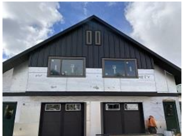
Building E8 Unit 58 Front Snap Batten Siding Installed
