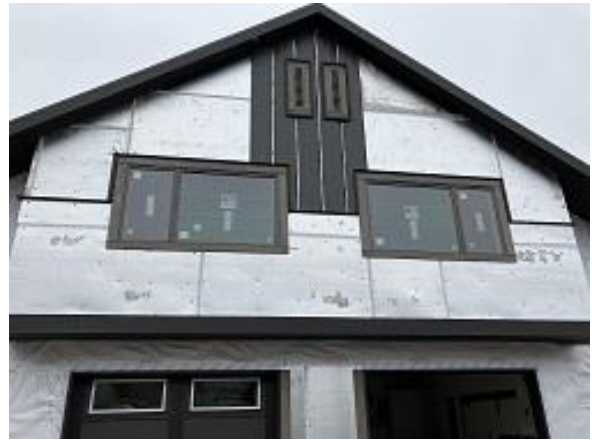
Building E8 Units 57 & 58 Front Snap Batten Siding Installation Began
