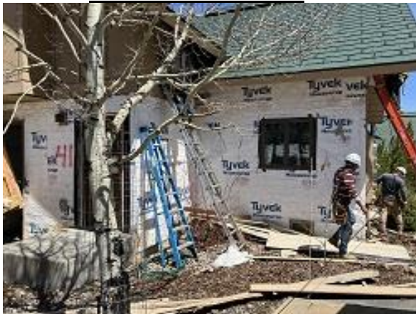
Building E5 Unit 41 Front & Side Demo Began
