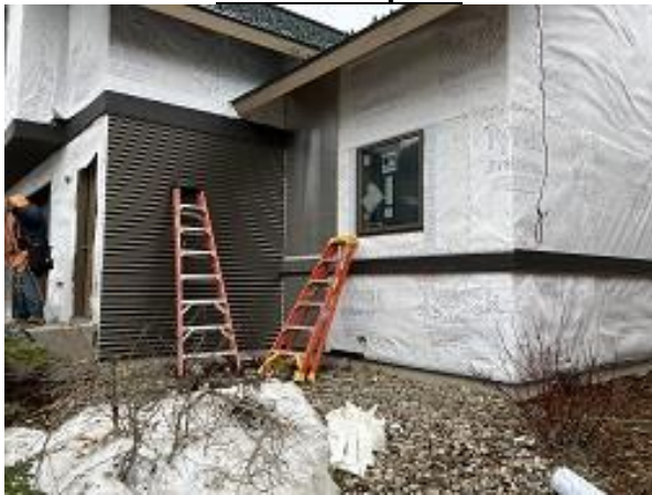
Building E8 Unit 55 Corrugated Siding Installed
