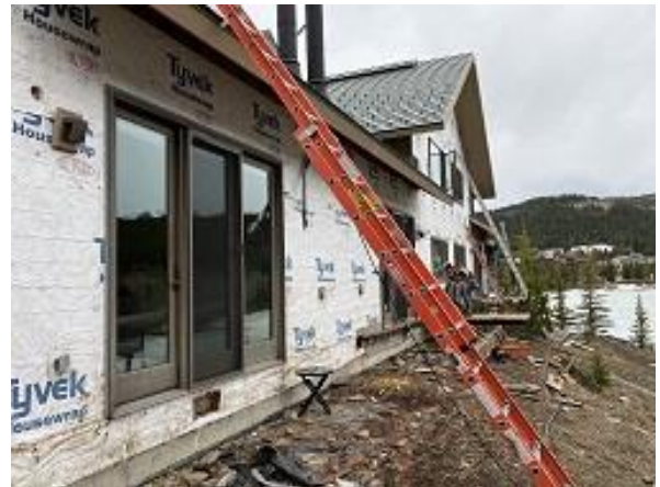
Building E5 Units 43 & 44 Back Demo Continued
