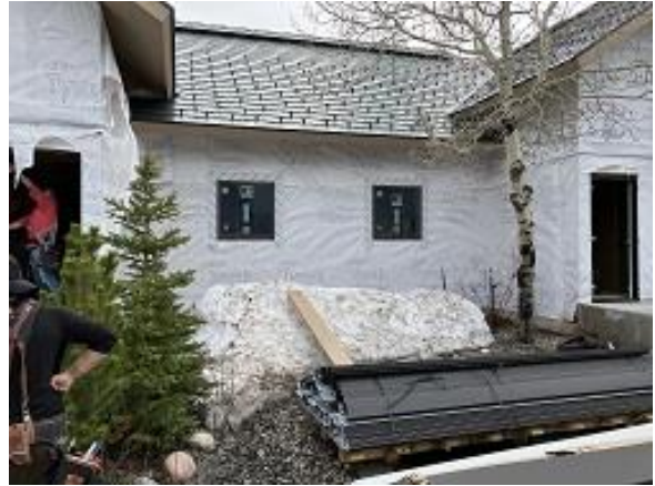
Building E6 Units 46 & 47 Front Doors & Windows Installed
