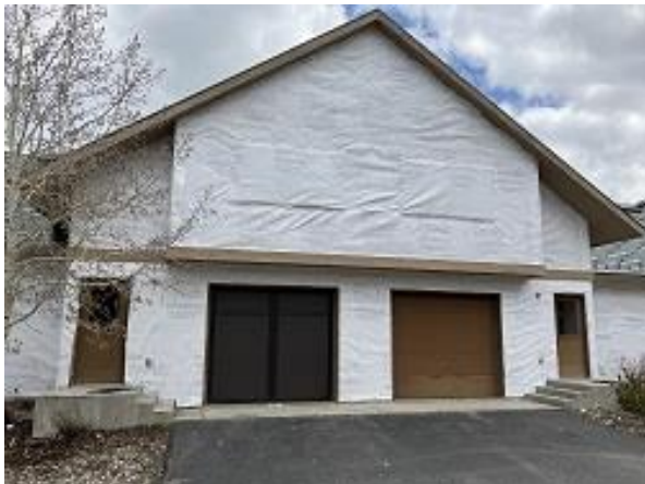
Building E9 Unit 61 & 62 Front Tyvek Installed
