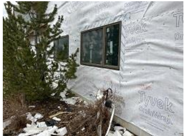
Building E8 Units 57 & 58 Back Lower Windows Installed
