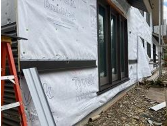
Building E8 Unit 55 & 56 Back Wainscot Flashing Installed
