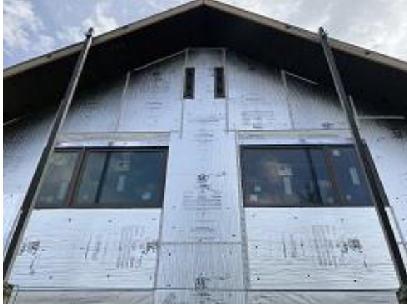
Building E8 Units 55 & 56 Back Soffit and Insulation Installed
