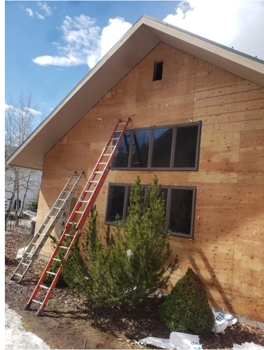
Building E5 Units 41 Side Sheathing Exposed
