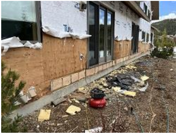
Building E5 Units 42 & 43 Deck Blocking Installed
