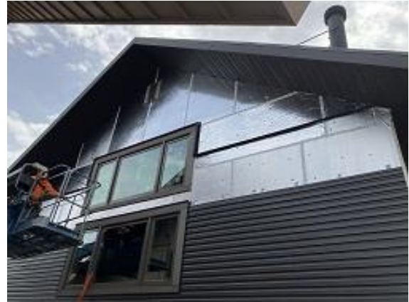
Building E8 Unit 55 Side Snap Batten Flashing Installed
