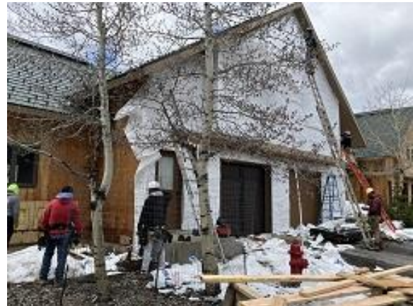
Building E6 Unit 45 & 46 Front Tyvek Installed
