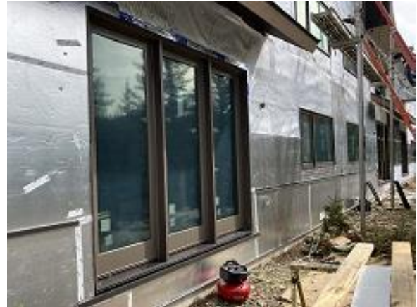
Building E8 Unit 55 & 56 Back Insulation Installed
