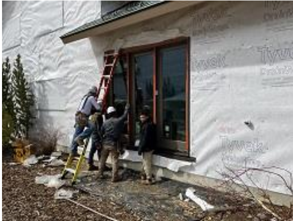
Building E6 Unit 47 Deck Door Installed
