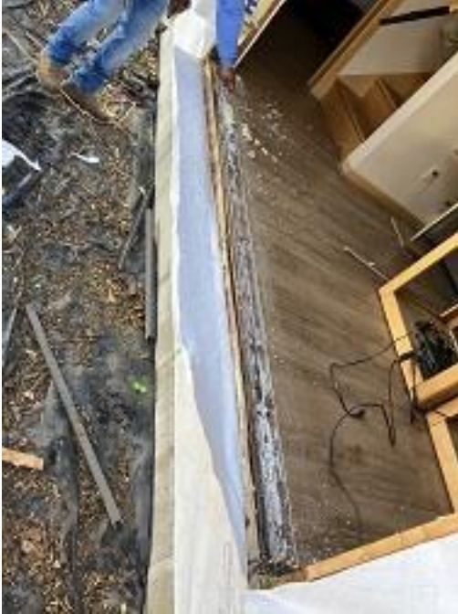
Building E6 Unit 45 Deck Door Removed
