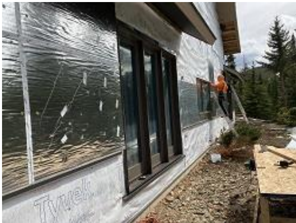
Building E8 Unit 57 & 58 Back Insulation Installed
