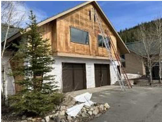
Building E5 Unit 41 & 42 Front Sheathing Exposed
