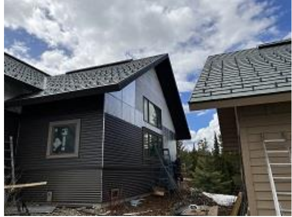
Building E9 Unit 55 Side Insulation & Lap Siding Installed
