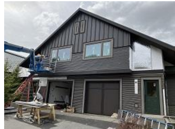
Building E8 Units 55 & 56 Front Lap Siding Installed
