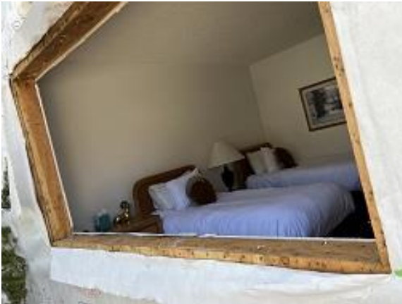
Building E6 Unit 45 Back Lower Window Removed
