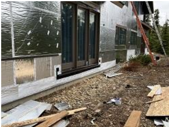
Building E8 Unit 57 Deck Ledger Flashing Installed
