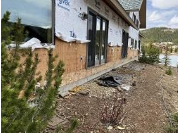
Building E5 Units 42 & 43 Deck Blocking Sheathing Installed
