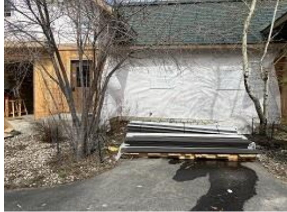
Building E5 Units 42 & 43 Front Tyvek Installed
