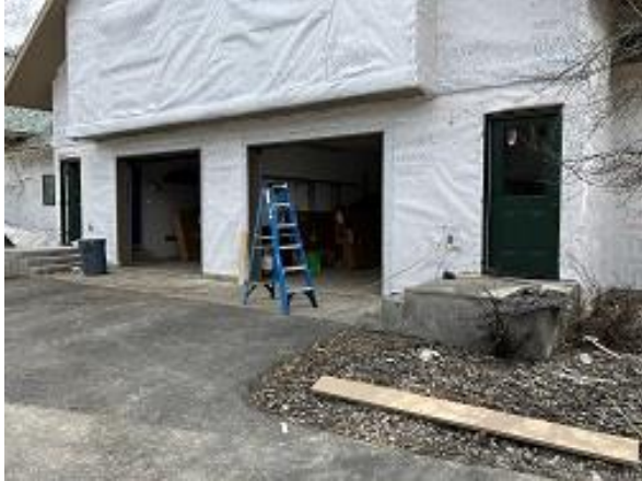
Building E6 Units 47 & 48 Front Doors Installed
