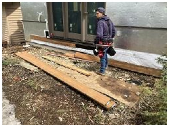
Building E8 Unit 55 Deck Ledger Board Installed
