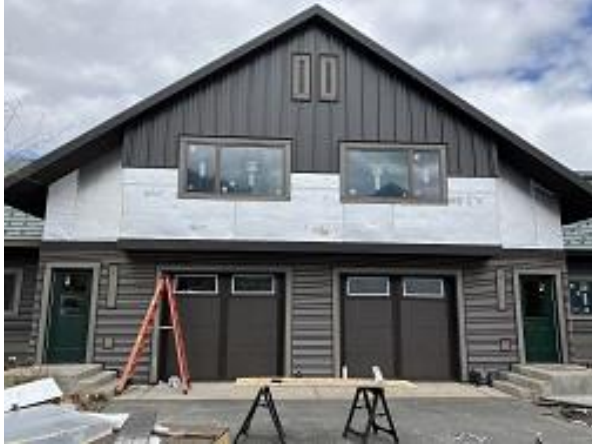
Building E8 Units 57 & 58 Front Corrugated Installed
