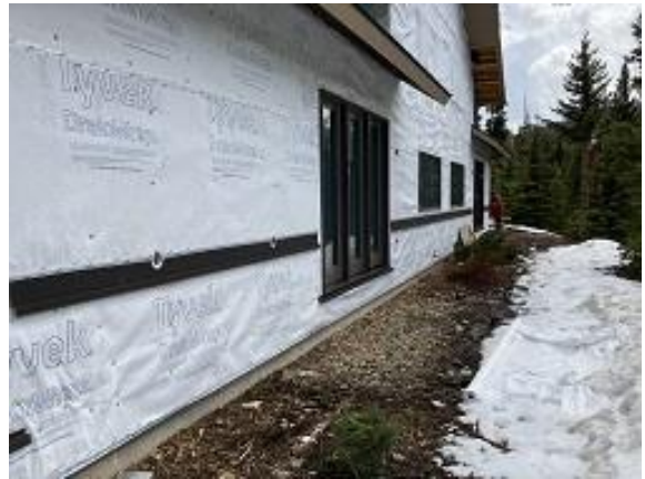
Building E8 Unit 57 & 58 Back Wainscot Flashing Installed
