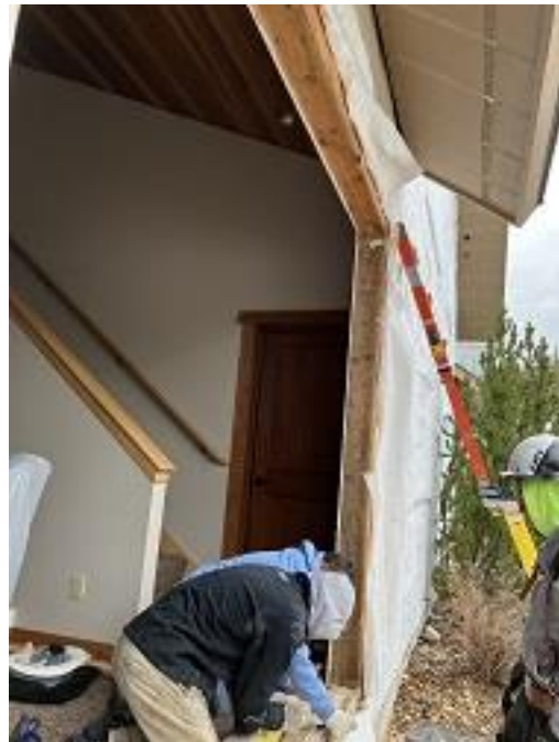
Building E6 Unit 48 Deck Door Removed
