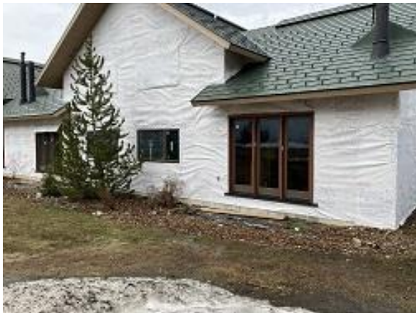
Building E6 Units 45 & 46 Deck Doors & Lower Back Windows Installed
