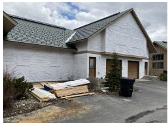
Building E9 Unit 63 & 64 Front Tyvek Installed
