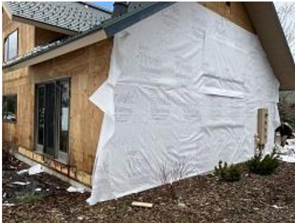
Building E6 Unit 45 Back Sheathing Exposed Side Tyvek Installed
