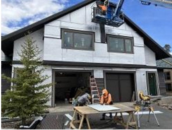
Building E8 Units 55 & 56 Front Snap Batten & Corrugated Installed
