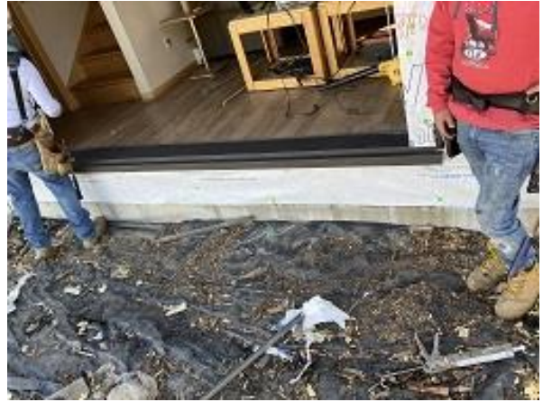
Building E6 Unit 45 Deck Door Pan Installed
