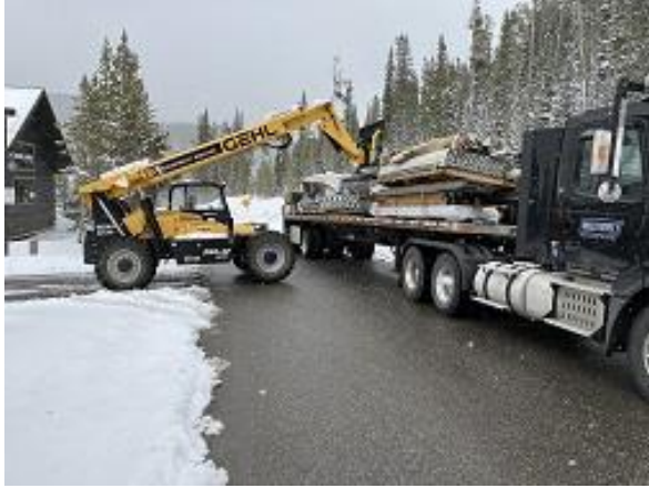
Delivery of Materials to Site from Storage Yard
