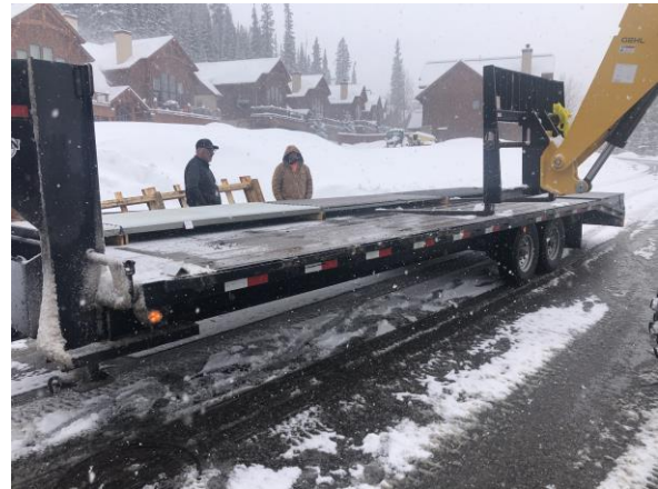
Delivery of E8 Siding Materials
