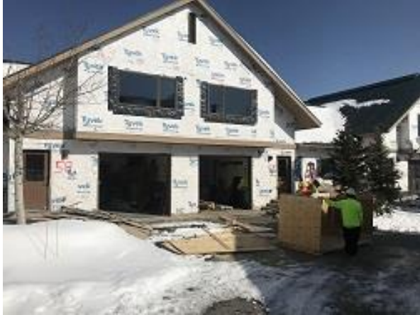
Building E8 Units 57 & 58 Front Demo Complete
