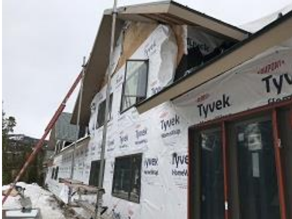
Building E8 Unit 57 & 58 Back Tyvek, Windows & Doors Installation Began
