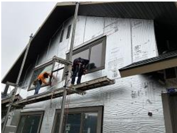
Building E8 Units 55 & 56 Back Snap Batten Flashing Installed
