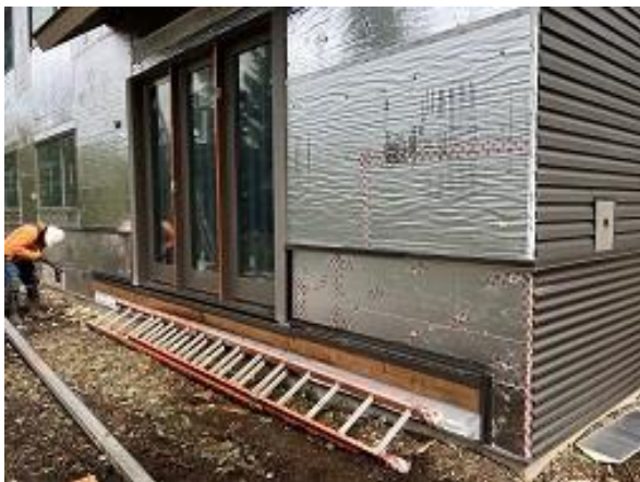
Building E8 Unit 58 Deck Ledger, Flashing and J Channel Installed
