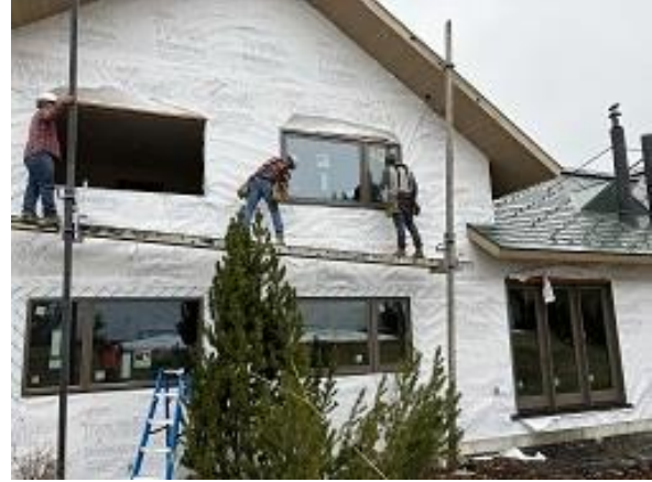
Building E6 Units 47 & 48 Back Upper Windows Installed
