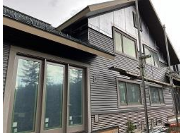
Building E8 Units 55 & 56 Back
