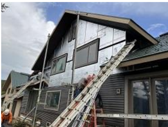
Building E8 Units 55 & 56 Back Lap Siding Installed
