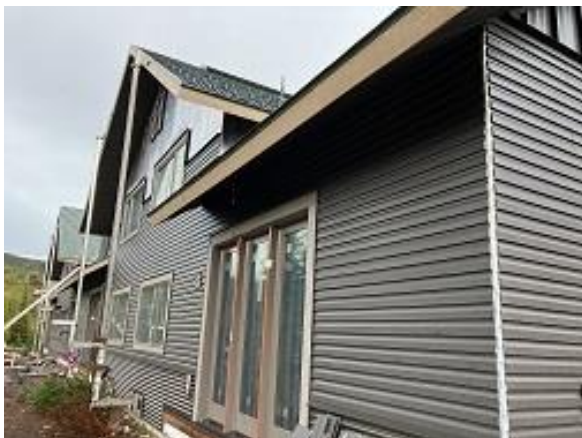
Building E8 Units 58 & 57 Back
