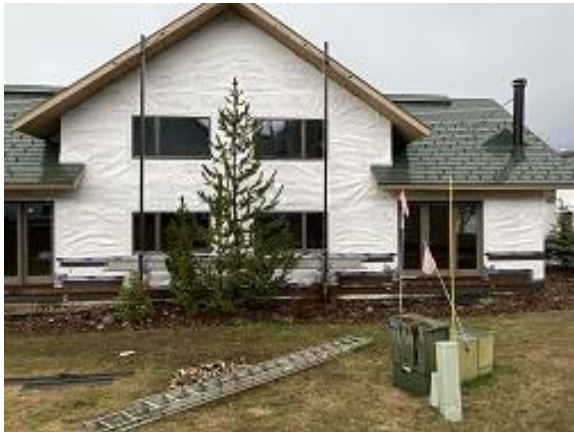
Building E6 Units 45 & 46 Back
