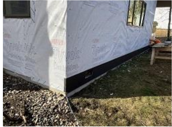
Building E6 Unit 48 Side Base Flashing Installed
