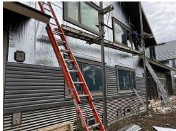
Building E8 Units 55 & 56 Back Lap Siding and Snap Batten Flashing Installed
