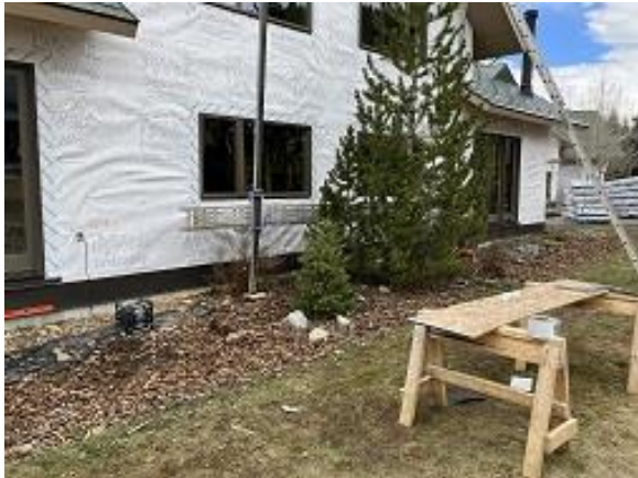
Building E6 Units 45 & 46 Back Base Flashing Installed
