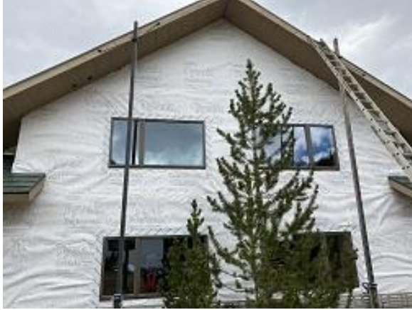
Building E6 Units 46 & 47 Back Upper Windows Installed
