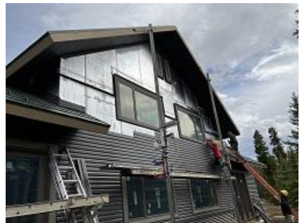
Building E8 Units 57 & 58 Back Lap Siding Installed
