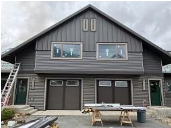
Building E8 Units 57 & 58 Front Lap Siding Installed
