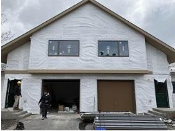
Building E6 Units 45 & 46 Front Upper Windows Installed
