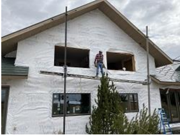
Building E6 Units 47 & 48 Back Upper Windows Removed
