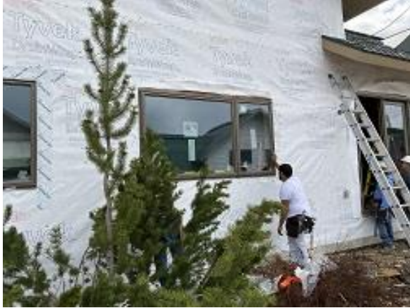
Building E9 Unit 63 Back Lower Window Installed
