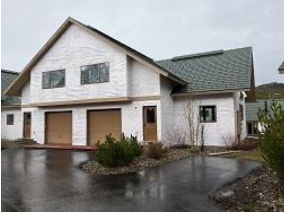
Building E9 Units 63 & 64 Front
