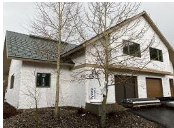
Building E9 Units 61 & 62 Front
