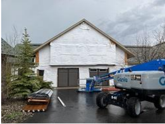
Building E5 Units 44 & 41 Front Tyvek Installed
