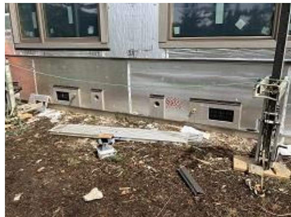
Building E8 Units 57 & 58 Back Block Outs Installed
