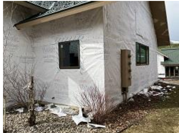
Building E9 Unit 64 Kitchen & Side Lower Window Installed
