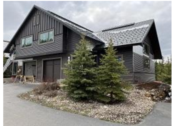
Building E8 Units 55 & 56 Front Lap Siding Installation Continued
