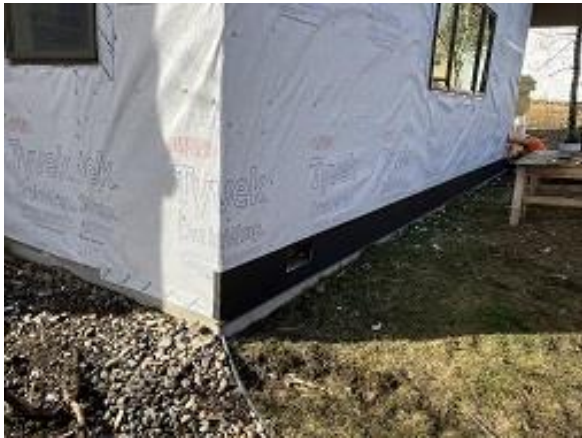
Building E6 Unit 48 Side Base Flashing Installed
