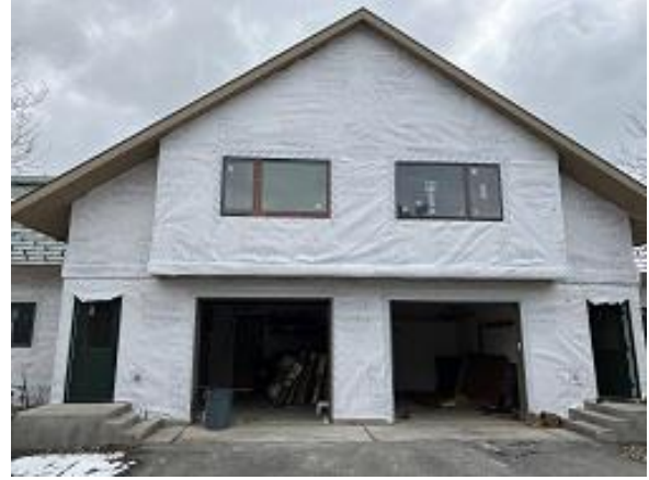
Building E6 Units 47 & 48 Front Upper Windows Installed
