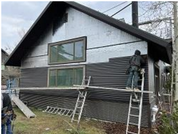
Building E6 Unit 48 Side Lap Siding Installed
