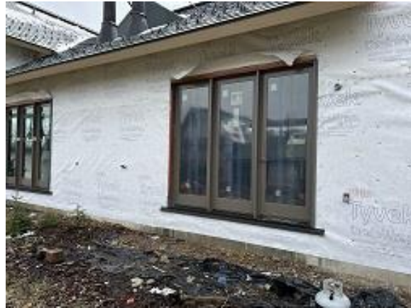
Building E9 Units 62 & 63 Deck Door Installed
