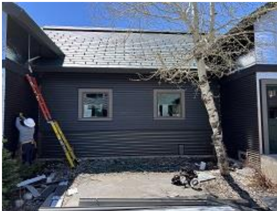
Building E6 Units 46 & 47 Front Corrugated and Lap Siding Installed
