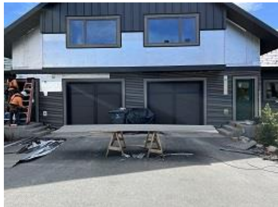
Building E6 Units 45 & 46 Front Corrugated Siding and Garage Door Installed
