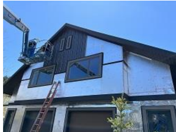
Building E6 Units 45 & 46 Front Snap Batten Siding Installed
