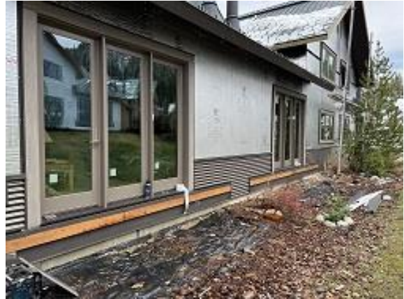
Building E6 Units 46 & 47 Back Corrugated Siding Installed
