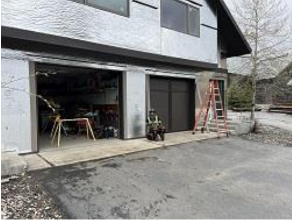
Building E6 Units 45 - 48 Garage Door Trim Installed
