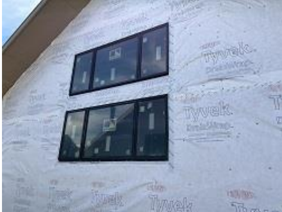
Building D Unit 38 Side Windows Installed
