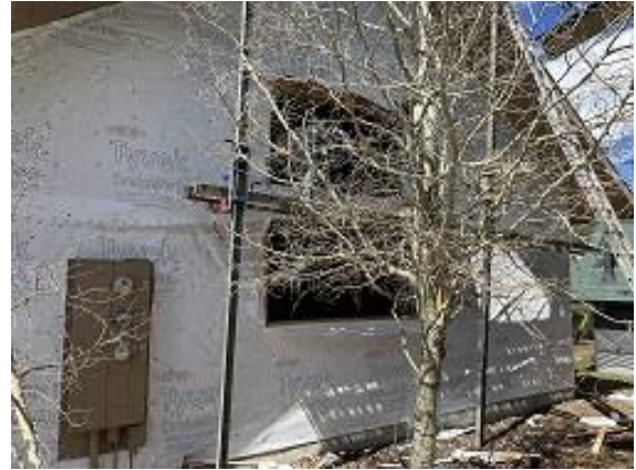
Building D Unit 36 Side Windows Installed
