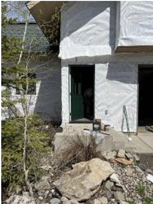
Building E5 Unit 42 Front Door Installed
