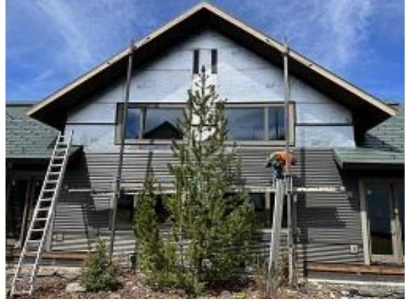
Building E6 Units 45 & 46 Back Lap Siding Installed
