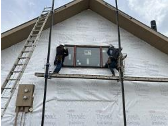
Building C5 Unit 40 Side Upper Window Installed
