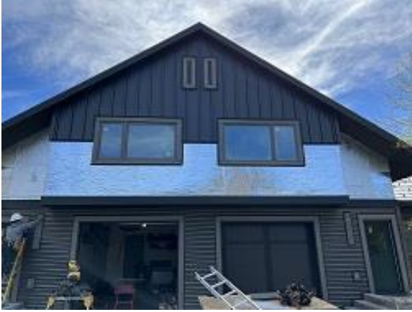
Building E6 Units 47 & 48 Front Snap Batten Siding Installed
