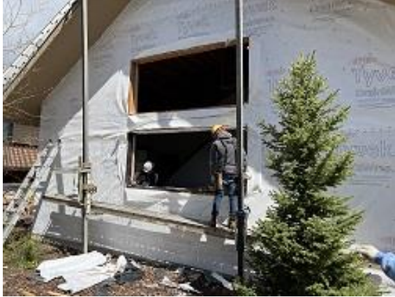
Building C5 Unit 39 Side Windows Removed
