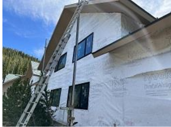
Building D Units 37 & 38 Back Windows Installed
