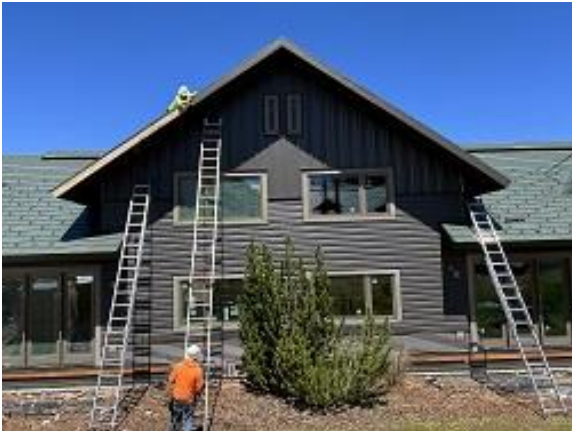
Building E6 Units 47 & 48 Back Fascia Installed
