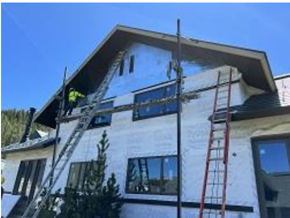
Building E9 Units 63 & 64 Back Insulation Installed
