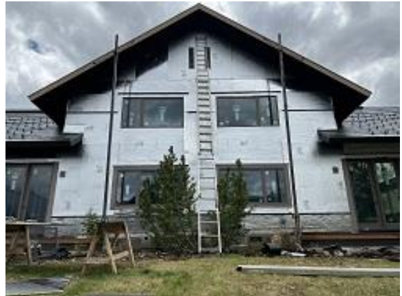
Building E9 Units 61 & 62 Back Door & Window Trim Installed
