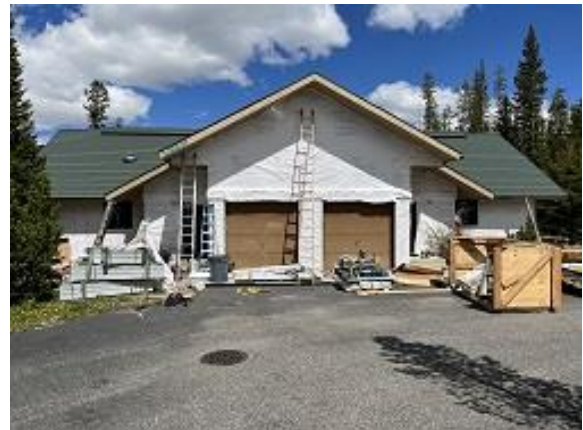
Building A Unit 2 Front Tyvek & Windows Installed
