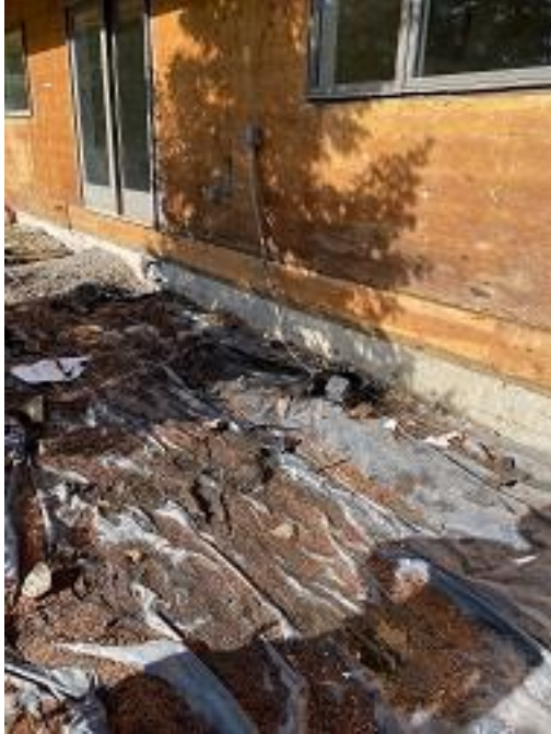
Building A Unit 1 Deck Sheathing Removed
