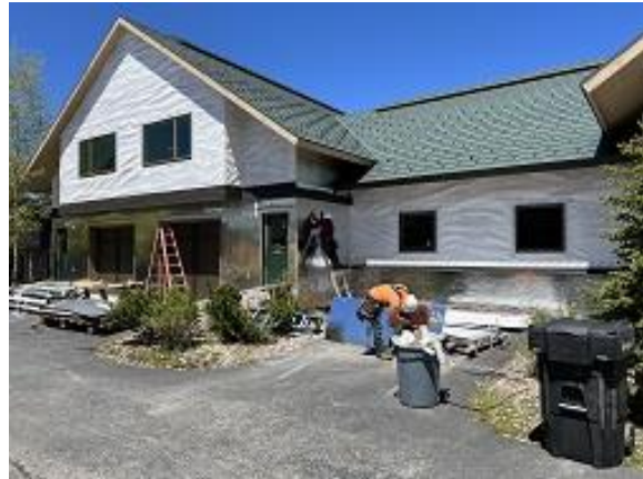
Building E9 Units 61 & 62 Front Insulation Installed
