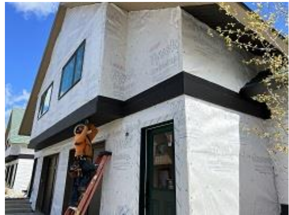
Building E9 Unit 64 Front Soffit and Belly Band Flashing Installed
