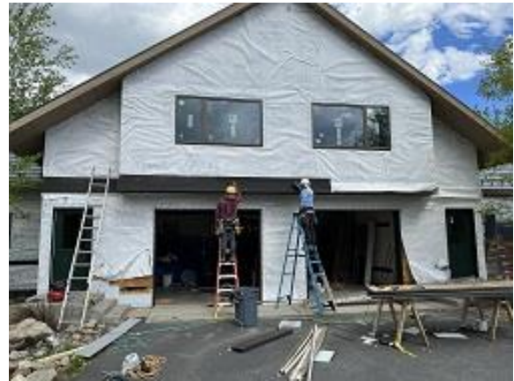
Building E6 Units 41 & 42 Front Belly Band Flashing and Soffit Installed
