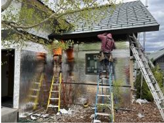
Building E5 Unit 41 Fascia Installed
