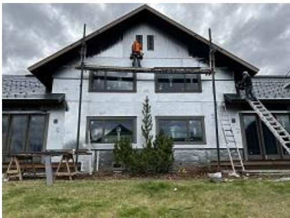
Building E9 Units 63 & 64 Back Door & Window Trim Installed
