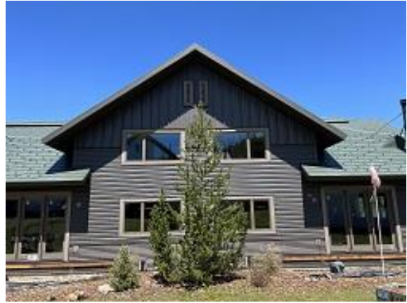
Building E6 Units 45 & 46 Back Fascia Installed
