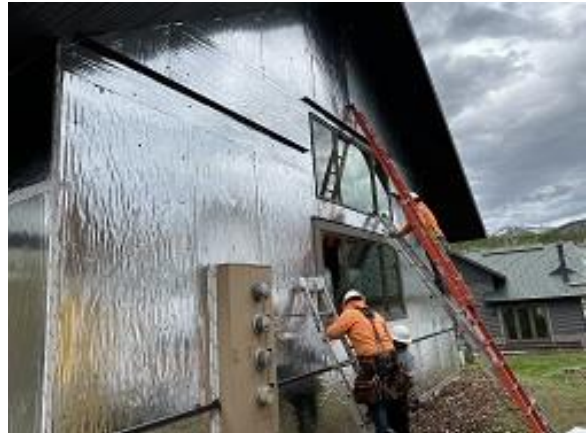
Building E9 Unit 64 Side Window Trim Installed
