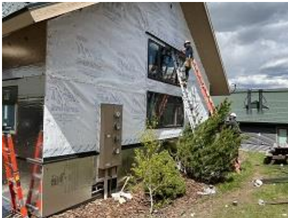
Building E6 Unit 41 Side Head Flashing and Insulation Installed
