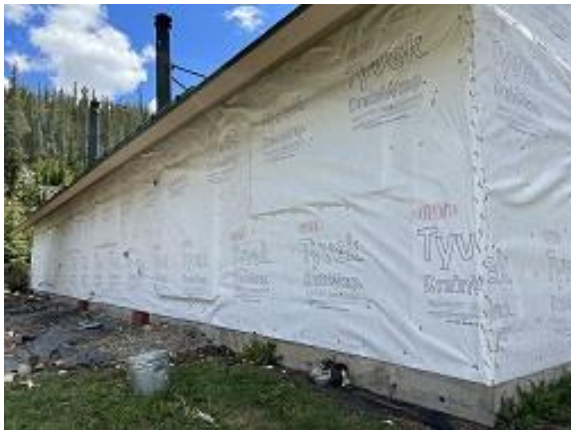
Building A Unit 2 Back Tyvek Installed
