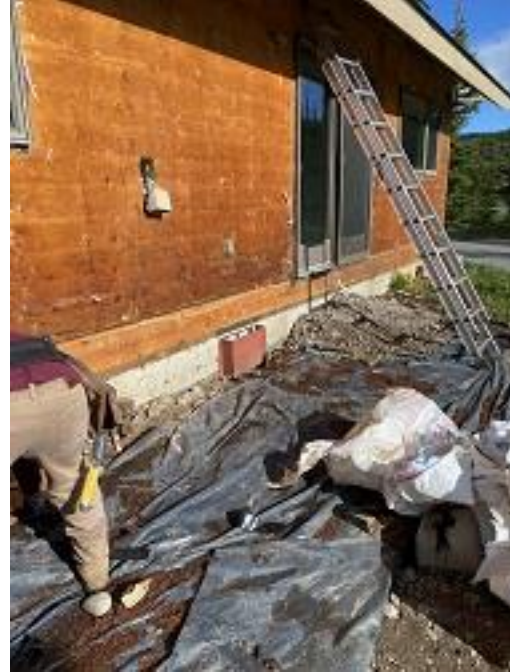
Building A Unit 2 Deck Sheathing Removed
