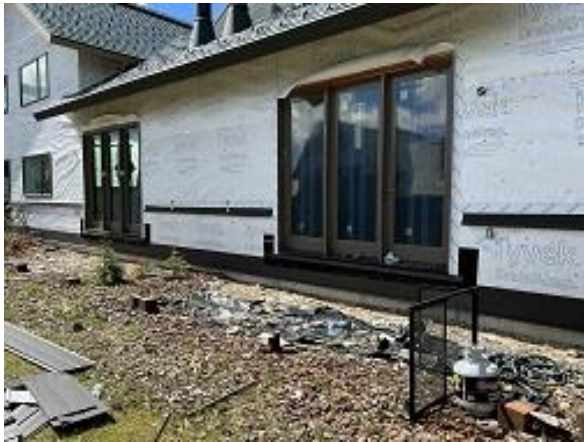
Building E9 Units 62 & 63 Back Base and Wainscot Flashing Installed
