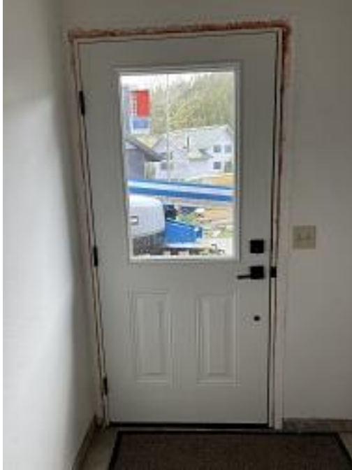
Building E8 Unit 55 Front Door Insulation Installed
