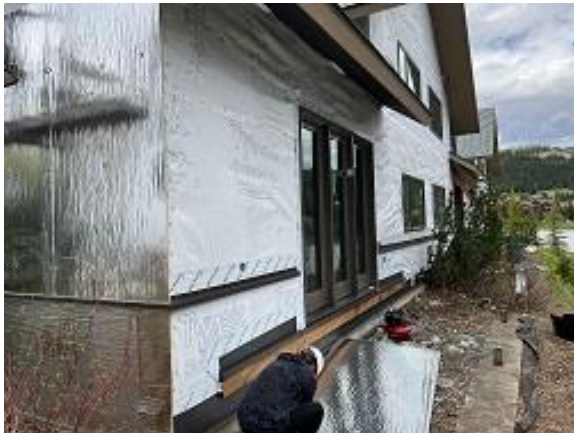
Building E5 Units 41 - 44 Soffit & Insulation Installed
