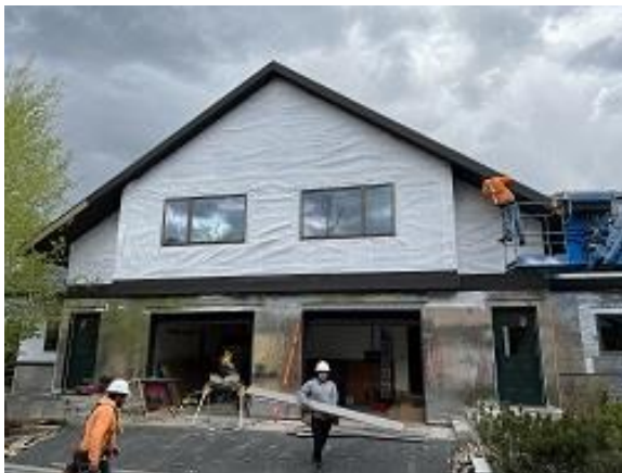
Building E9 Units 61 & 62 Front Soffit, Fascia and Insulation Installed
