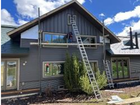
Building E6 Units 45 & 46 Back Snap Batten Siding Installed
