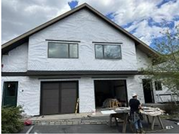
Building E6 Units 43 & 44 Front Base and Head Flashing Installed
