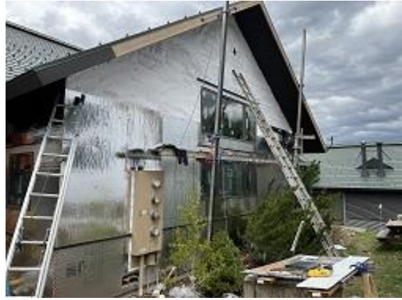
Building E5 Unit 41 Insulation, Soffit & Fascia Installed
