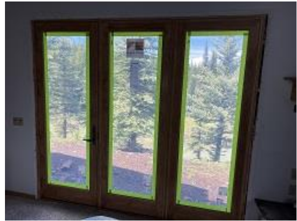
Building E8 Unit 55 Deck Door Insulation Installed
