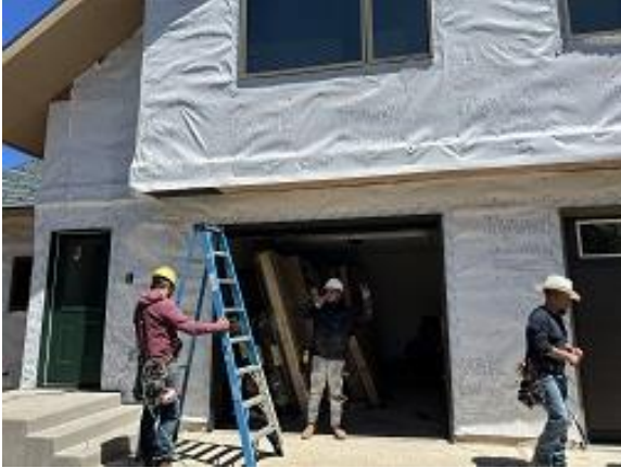
Building E5 Units 43 & 44 Front Garage Door Trim & Soffit Installed
