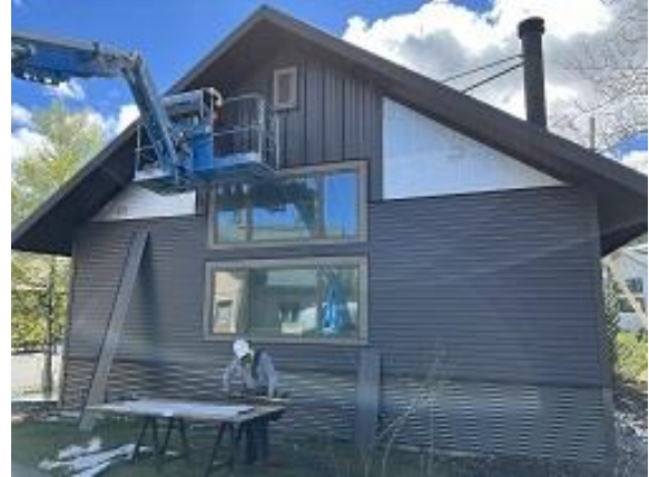
Building E6 Unit 48 Side Snap Batten Siding Installed
