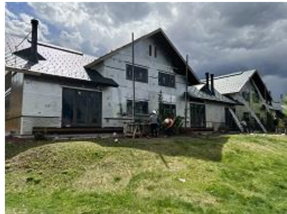
Building E9 Units 61 - 64 Back Insulation Installed
