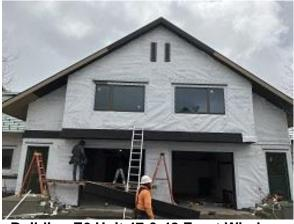
Building E6 Unit 47 & 48 Front Window Head Belly Band Flashing Installed
