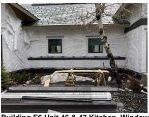
Building E6 Unit 46 & 47 Kitchen Window Head & Wainscot Flashing Installed
