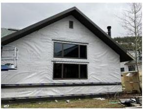
Building E6 Unit 48 Side Soffit, Window Head & Wainscot Flashing Installed
