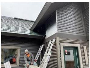
Building E8 Units 58 Front Roof Flashing, Insulation & J Channel Installed
