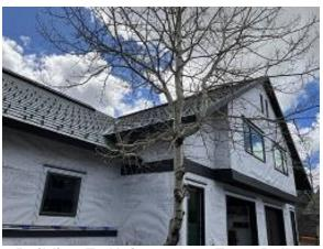
Building E6 Units 47 & 48 Front Belly Band, Soffit & Fascia Installed
