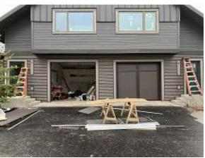
Building E8 Units 55 & 56 Front Corrugated Siding Installed
