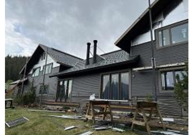
Building E95 Units 62 & 63 Back Lap Siding Installed
