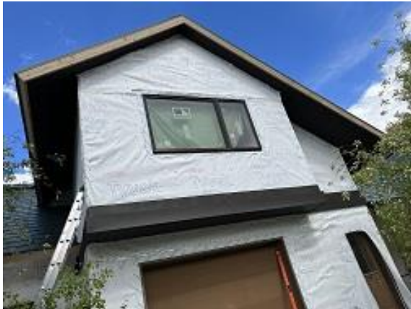
Building D Unit 36 Front Soffit Installed
