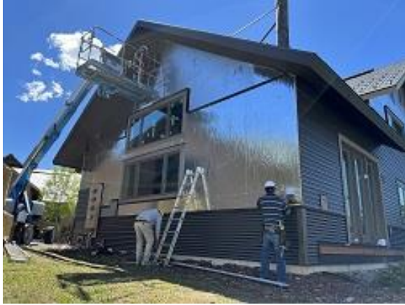
Building E9 Unit 64 Side Corrugated & Lap Siding Installed
