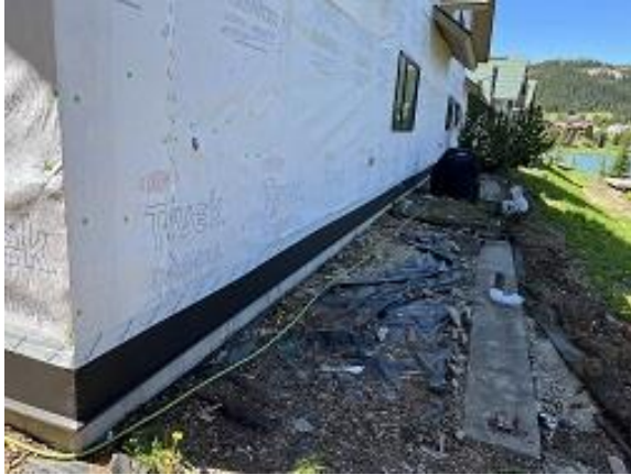
Building D Unit 36 Back Base Flashing Installed
