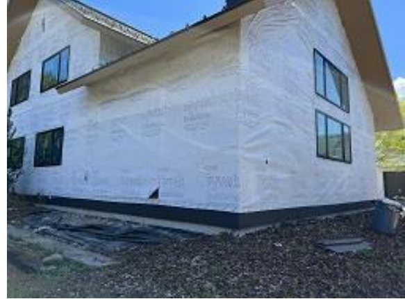
Building D Units 37 Back & 38 Back and Side Base Flashing Installed
