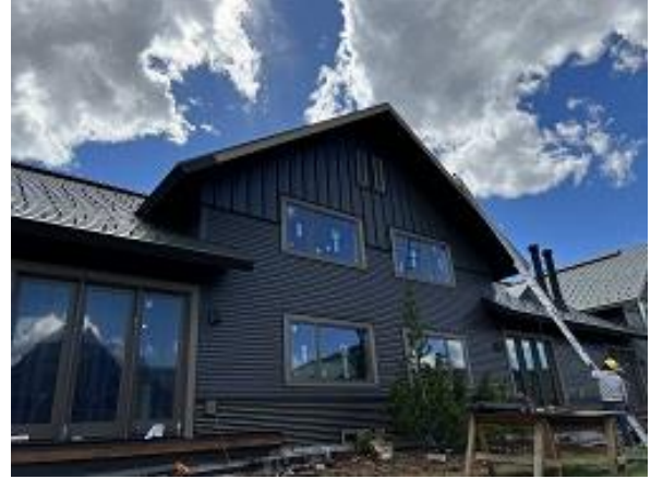
Building E9 Units 63 & 64 Back Snap Batten Siding Installed
