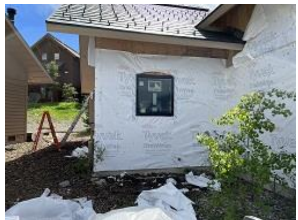
Building C8 Unit 66 Front Kitchen Window Installed
