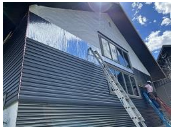
Building E5 Unit 44 Side Lap Siding Installed
