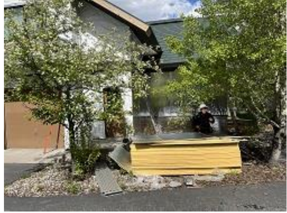
Building D Unit 36 Front Fascia, Soffit and Insulation Installed
