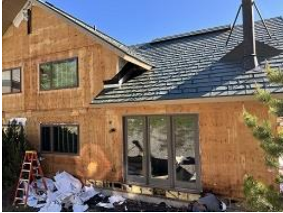
Building C8 Unit 66 Back Tyvek & Deck Sheathing Removed
