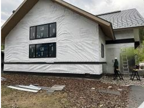
Building D Unit 38 Side Wainscot Flashing and Front Insulation Installed
