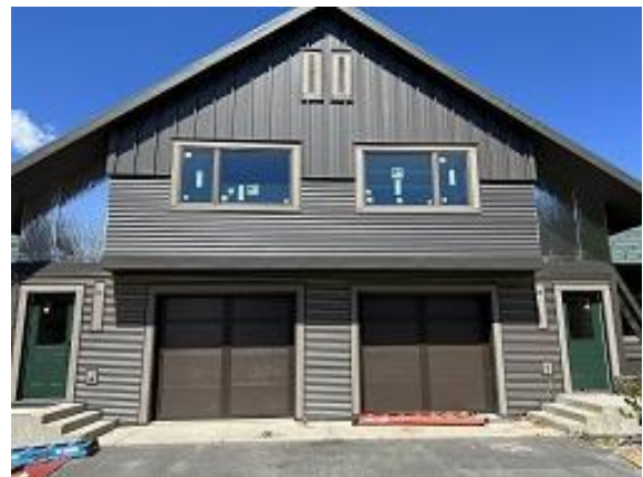
Building E9 Units 63 & 64 Front Lap & Snap Batten Siding Installed
