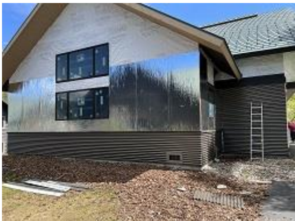
Building D Unit 38 Side & Front Corrugated Siding and Insulation Installed
