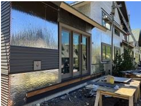
Building E5 Unit 41 Back Lap Siding Installed
