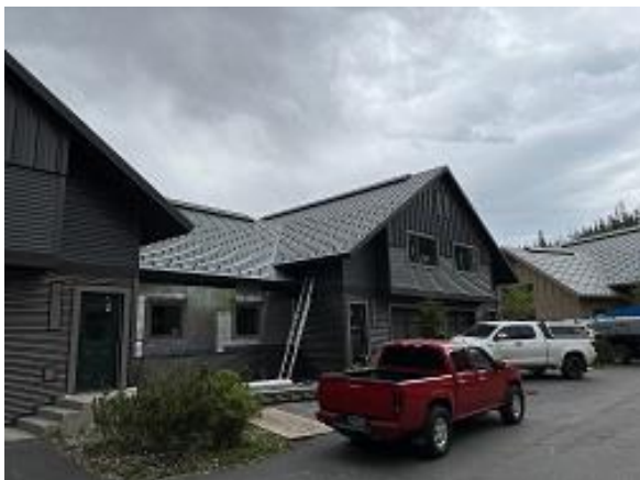
Building E95 Units 62 & 63 Front Lap Siding Installed
