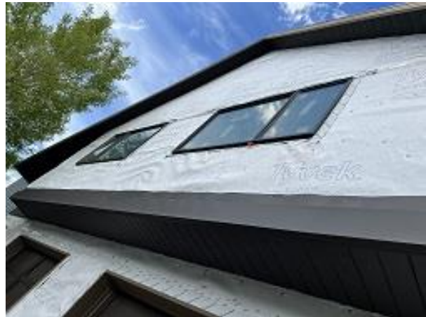
Building D Units 37 & 38 Front Soffit Installed
