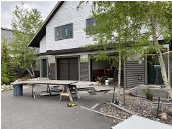
Building E5 Units 43 & 44 Front Corrugated Siding Installed
