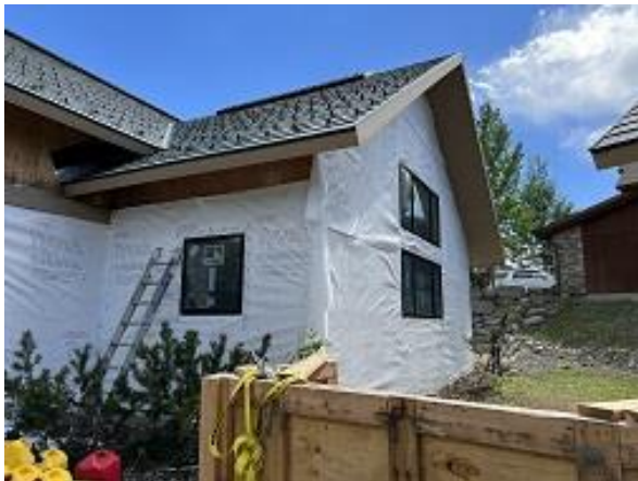
Building C8 Unit 65 Front Kitchen and Side Windows Installed
