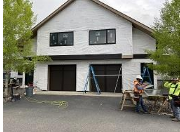
Building D Units 37 & 38 Front Belly Band Flashing Installed
