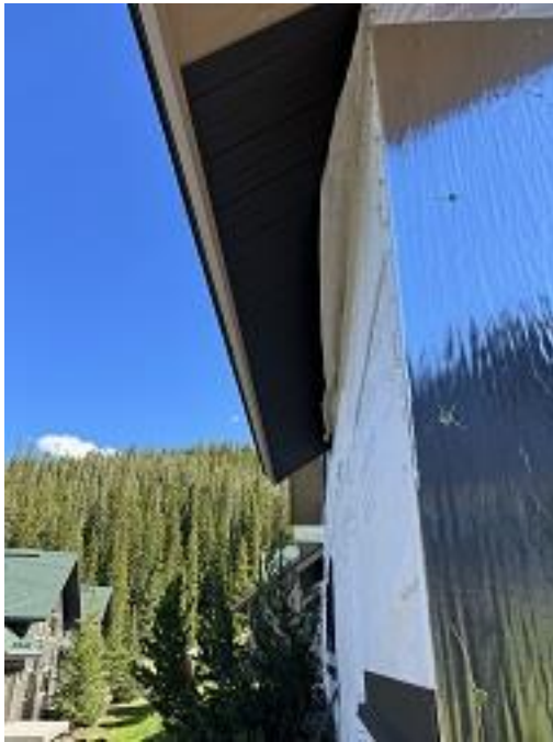
Building D Unit 38 Back Soffit Installed
