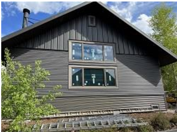
Building E9 Unit 61 Side Lap Siding Installed
