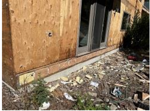
Building C8 Unit 65 Back Deck Blocking Installed
