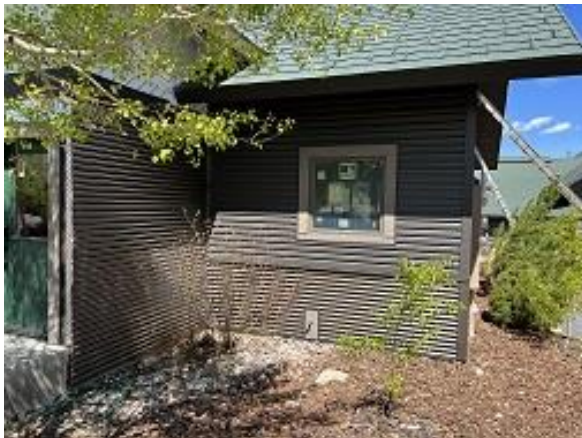
Building E5 Unit 41 Front Corrugated & Lap Siding Installed
