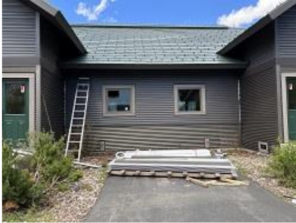
Building E9 Units 62 & 63 Front Lap Siding Installed
