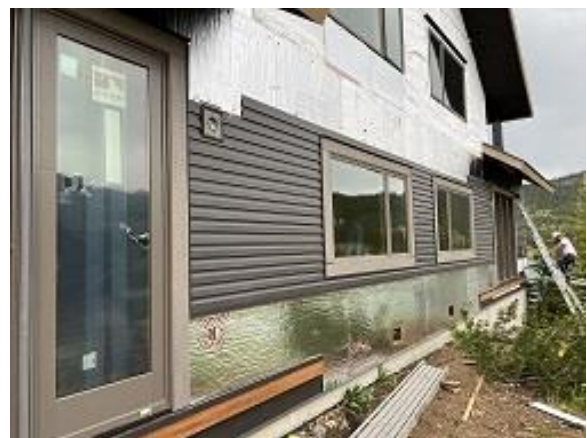
Building E5 Units 43 & 44 Back Lap Siding Installed
