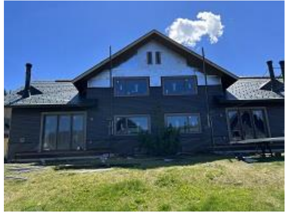
Building E9 Units 63 & 64 Back Lap Siding Installed
