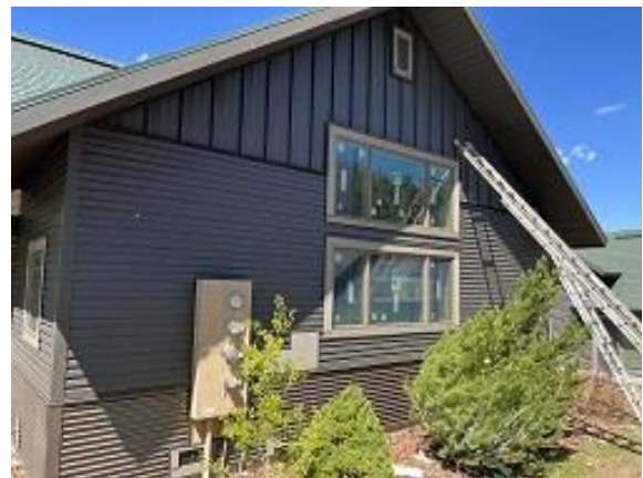
Building E5 Unit 41 Side Fascia Installed
