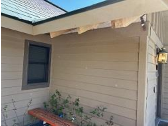
Building B Unit 4 Front Roof Framing Repairs Began
