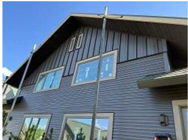
Building E9 Units 61 & 62 Back Snap Batten Siding Installed
