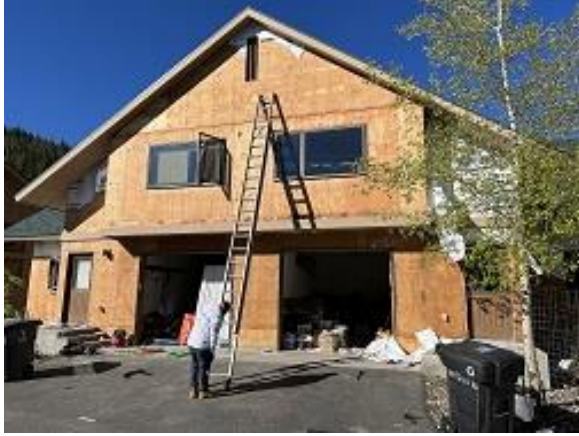
Building C8 Units 65 & 66 Front Demolition Complete
