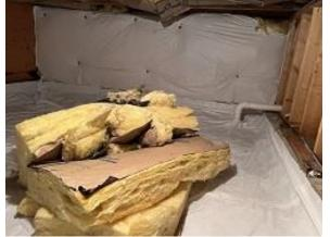
Building E3 Unit 25 Crawl Space Radon Plastic & Footing Crossover Vent Installed
