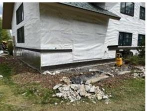
Building C5 Unit 40 Side & Back Base & Wainscot Flashing & Insulation Installed and Deck Footing Demolition Complete
