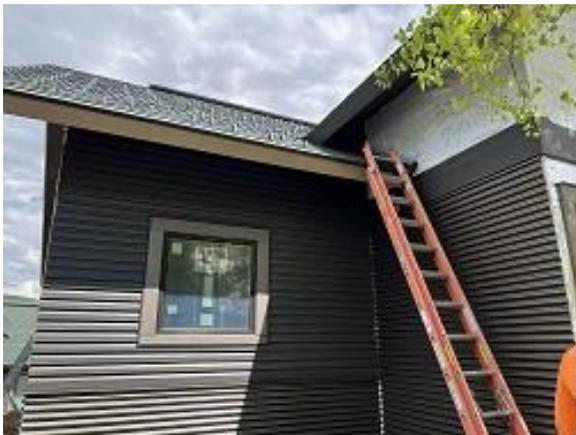
**Building D Unit 38 Front Lap Siding and Diverter Installed**
