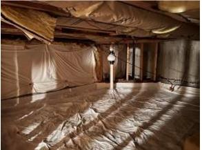
Building E3 Unit 25 Crawl Space Radon Plastic & Exhaust Fan Installed
