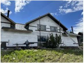
Building D Units 37 & 38 Back Snap Batten & Head Flashing Installed
