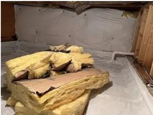
**Building E3 Unit 25 Crawl Space Radon Plastic & Footing Crossover Vent Installed**
