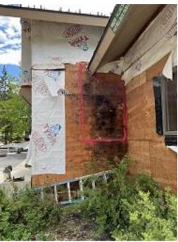
Building C1 Unit 12 Front Tyvek Removed and Damaged Area Marked
