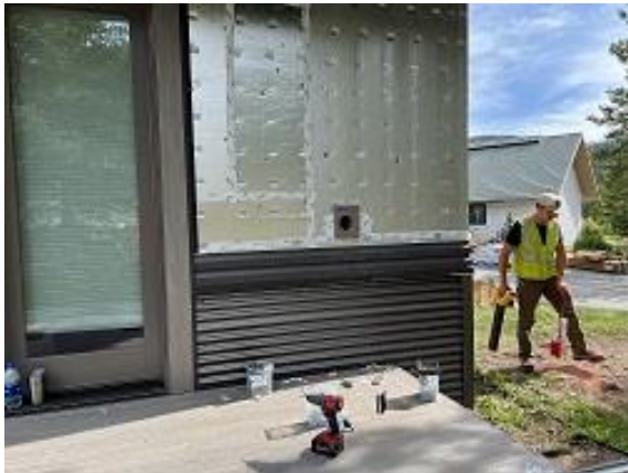
Building E1 Unit 8 Back Lap Siding Removed to Locate Fireplace Vent
