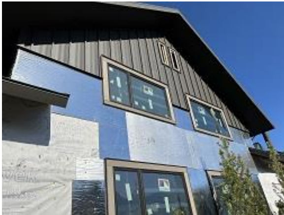
Building D Units 37 & 38 Back Snap Batten Siding Installed
