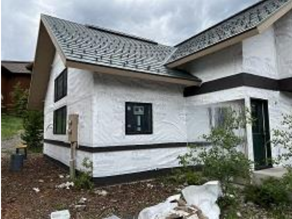
Building C8 Unit 66 Front & Side Base & Wainscot Flashing Installed
