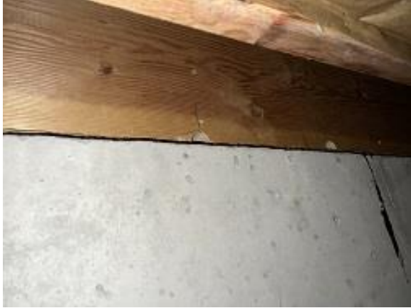
Building C1 Unit 12 Deck Ledger Blocking Installed in Crawl Space
