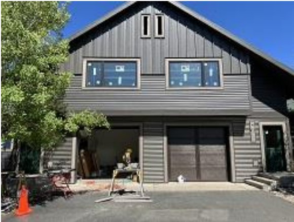
Building D Units 37 & 38 Front Corners Installed
