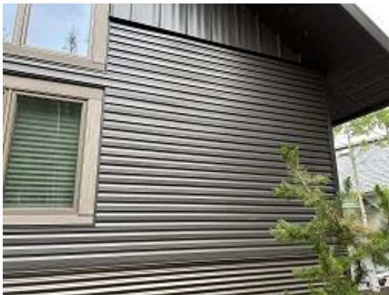
Building E3 Units 27 Side Wire Penetration Repaired
