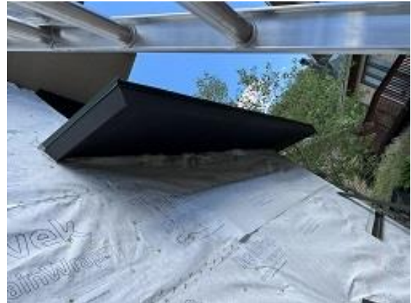
Building C5 Unit 39 Back Soffit & Fascia Installed
