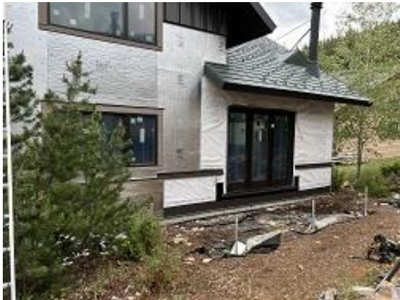
Building C5 Unit 39 Deck Door & Helical Piers Installed
