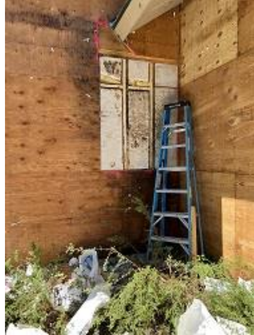
Building C1 Unit 12 Front Sheathing Exposed Substrate Repaired
