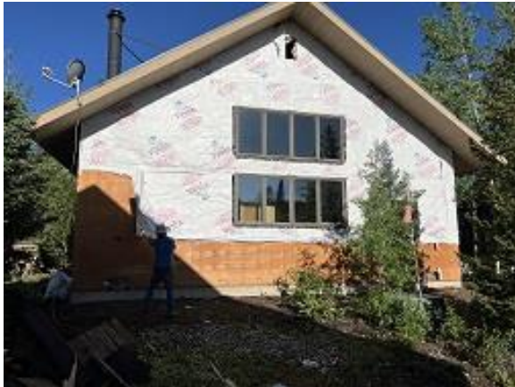
Building C2 Unit 14 Side Sheathing Exposed
