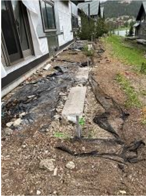
Building D Units 36 & 37 Deck Helical Piers Installed
