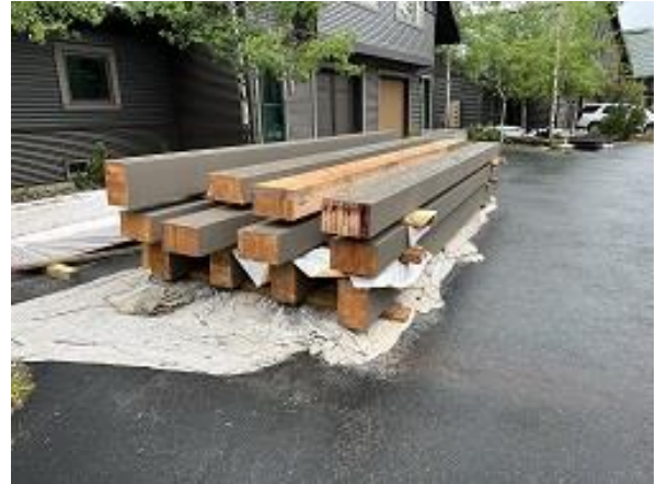
Deck GLULAM Painting Continued
