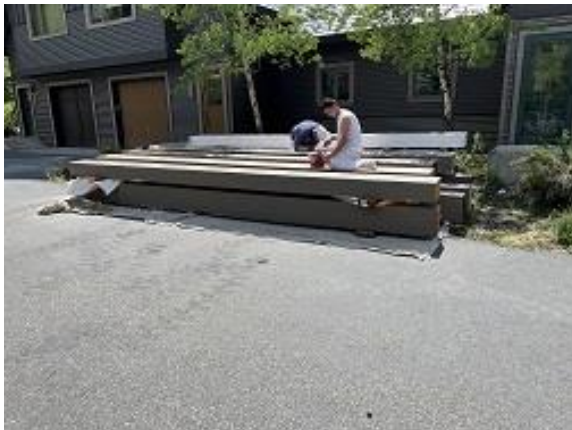
Deck GLULAMs Painting Continued
