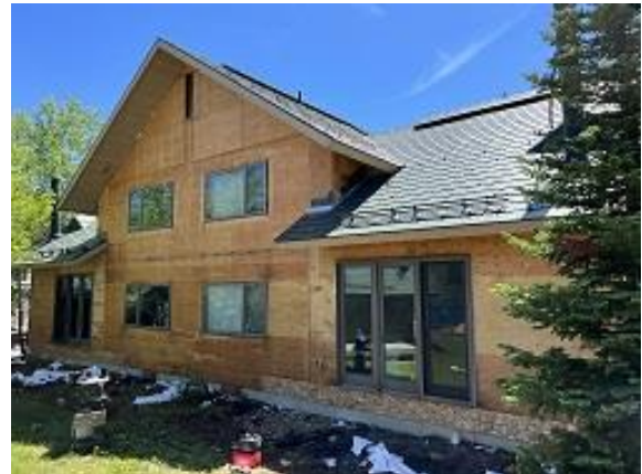
Building C1 Units 12 & 13 Back Sheathing Exposed & Deck Sheathing Installed
