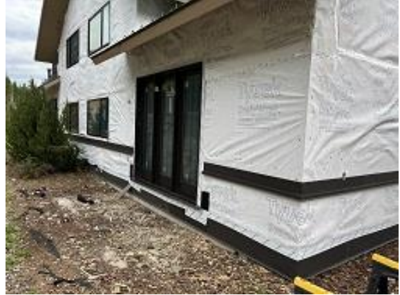
Building C8 Units 65 & 66 Back Base & Wainscot Flashing and Deck Door Installed
