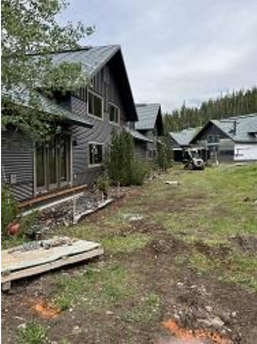
Building E6 Units 45 - 48 Deck Helical Piers Installed
