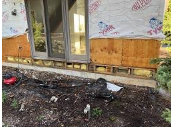
Building C2 Unit 14 Deck Ledger Sheathing Removed
