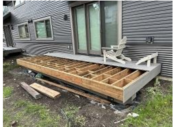
Building E2 Unit 23 Decking Removed for Railing Installation
