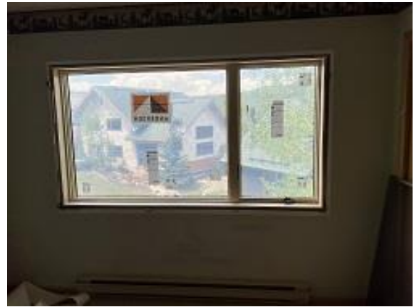
Building C1 Unit 12 Back Upper Window Installed
