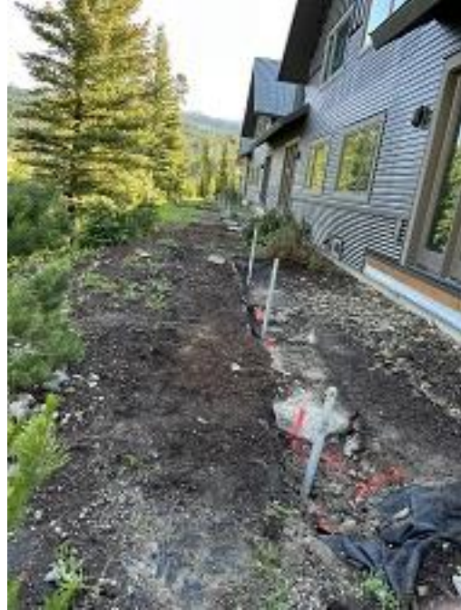
Building E8 Units 55 - 58 Deck Helical Piers Installed
