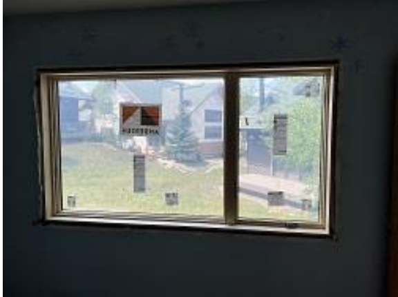
Building C1 Unit 12 Back Lower Window Installed
