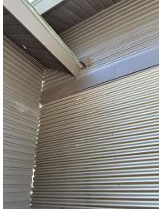
Building E5 Unit 44 Front Diverter & Lap Siding Installed
