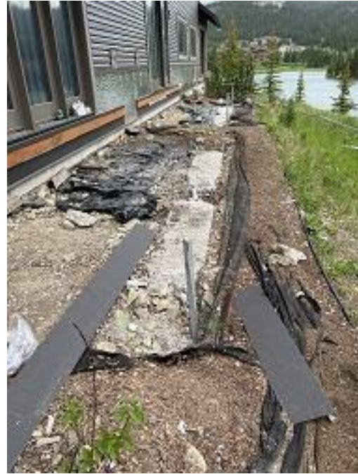
Building E5 Units 42 & 43 Deck Helical Piers Installed
