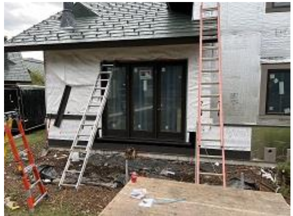
Building C5 Unit 40 Deck Door & Helical Piers Installed
