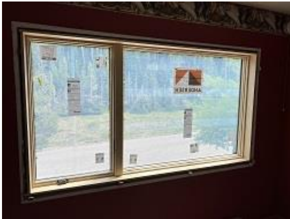
Building C1 Unit 12 Front Upper Window Installed
