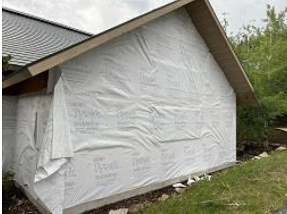
Building C2 Unit 15 Side Tyvek Installed
