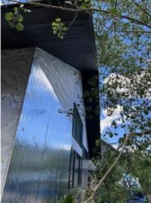
Building C5 Unit 39 Side Soffit & Fascia Installed
