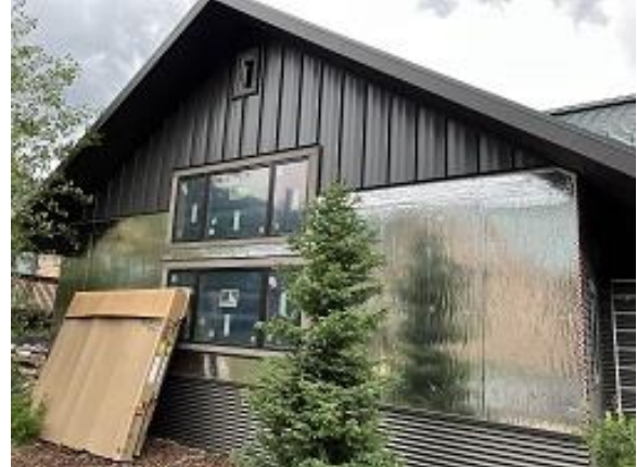
Building C5 Unit 39 Side Snap Batten Siding Installed
