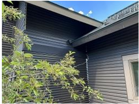
Building E5 Unit 41 Front Diverter and Lap Siding Installed
