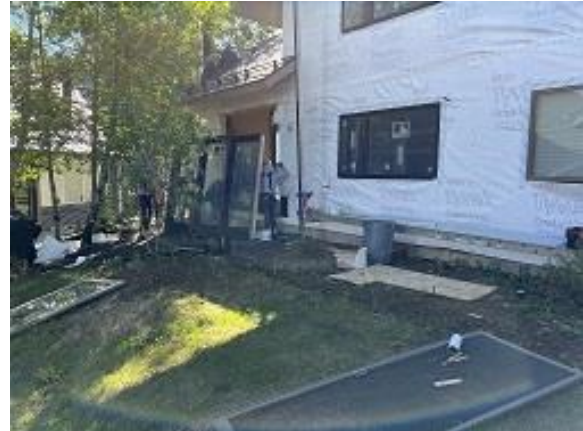
Building C1 Unit 12 Deck Door Installation
