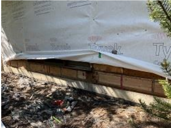
Building C2 Unit 15 Deck Ledger Blocking Completed
