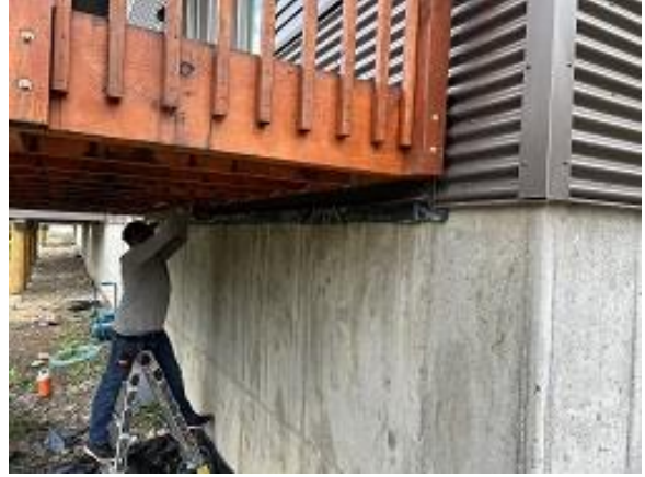
Building E7 Unit 52 Deck Ledger Flashing Installation
