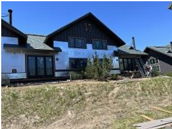
Building D Units 37 & 38 Back Lap Siding Installation Continued
