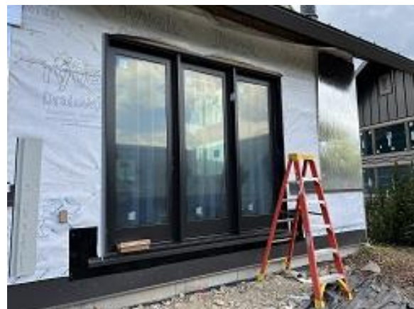
Building D Unit 38 Deck Door Installation Began
