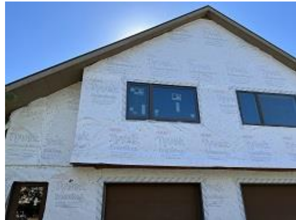
Building C3 Unit 33 Front Upper Window Installed
