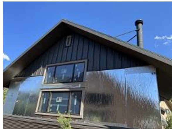
Building C8 Unit 65 Side Snap Batten Siding Installed
