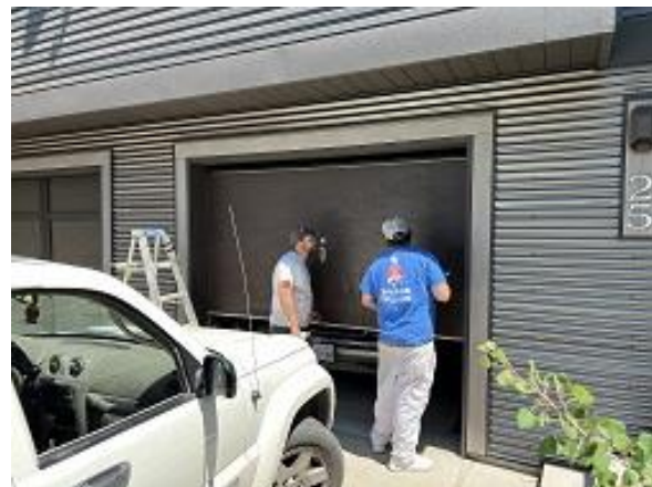
Building E3 Unit 25 Garage Door Painted
