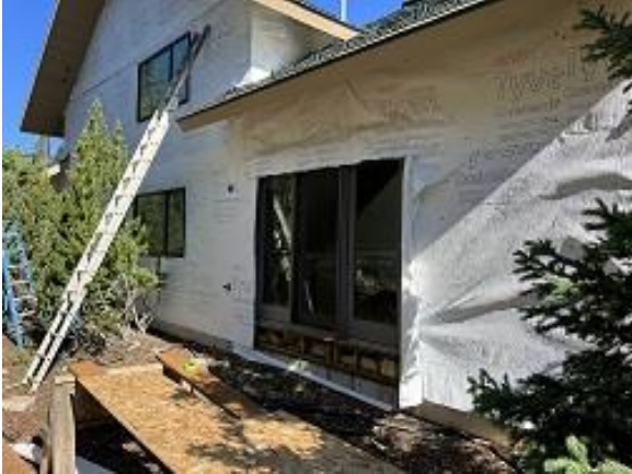
Building C2 Unit 14 Back Windows Installation Began
