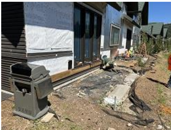
Building D Units 36 & 37 Deck Ledger Installed
