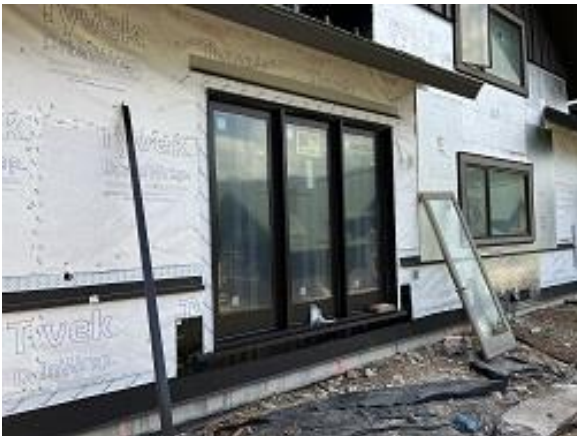
Building D Unit 36 Deck Door Installation Began
