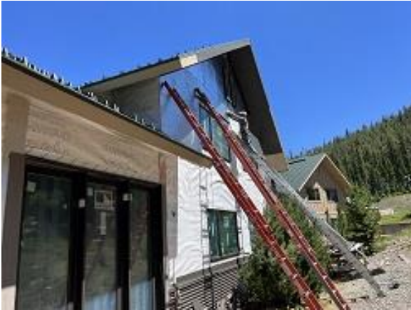
Building C8 Units 65 & 66 Back Head Flashing and Insulation Installed
