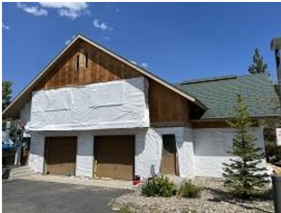
Building C3 Units 32 & 33 Front Tyvek Installed
