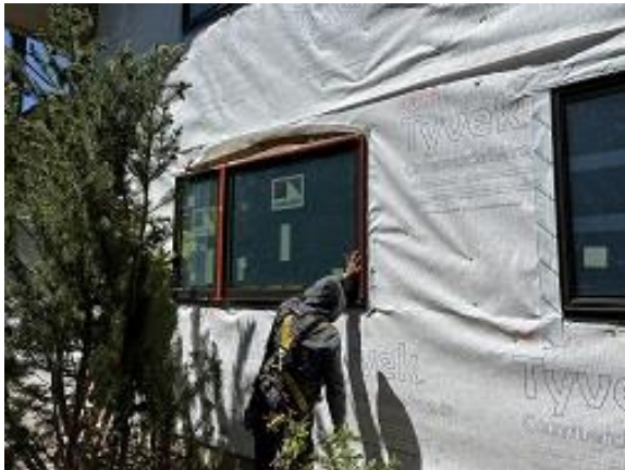
Building C2 Unit 15 Back Lower Window Installed
