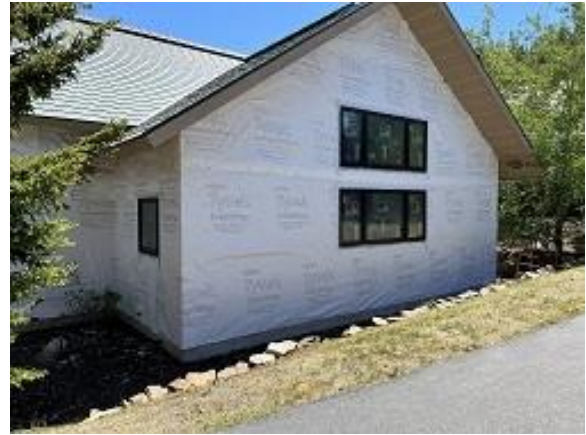
Building C2 Unit 15 Front & Side Windows Installed
