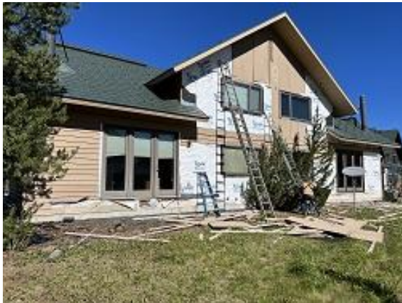
Building C3 Units 32 & 33 Back Siding Demolition
