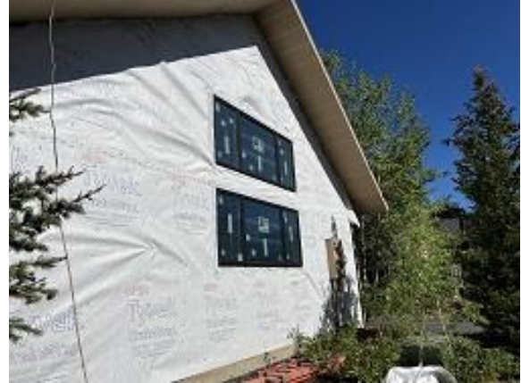
Building C2 Unit 14 Side Windows Installation Began
