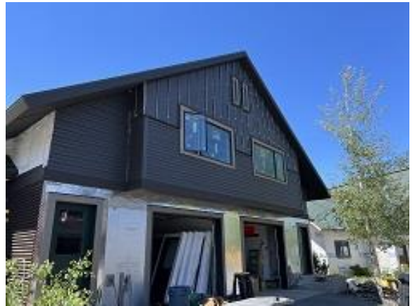
Building C8 Units 65 & 66 Front Snap Batten Siding Installation
