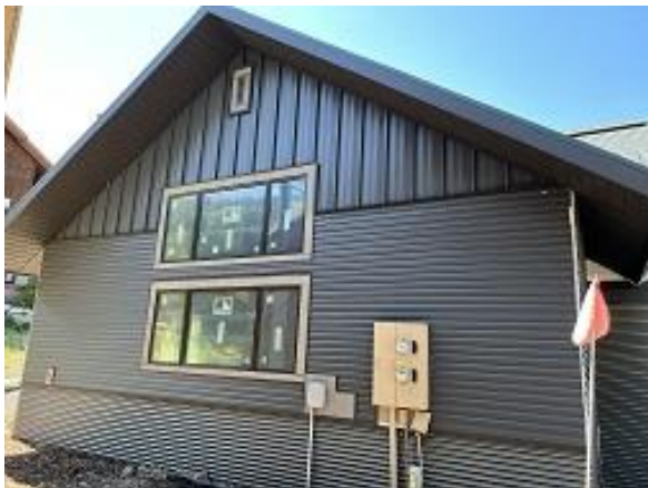
Building C8 Unit 66 Side Snap Batten Siding Installed
