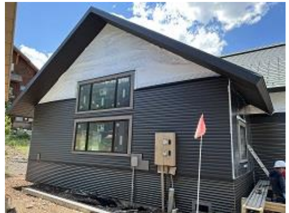
Building C8 Unit 66 Side Lap Siding Installed
