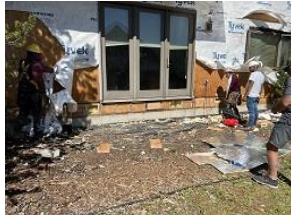
Building C3 Unit 32 Deck Ledger Sheathing Removed & Blocking Installed
