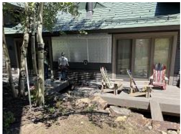
Building E1 Units 10 & 11 Lap Siding Replacement Around Fireplace Vents Uncovered
