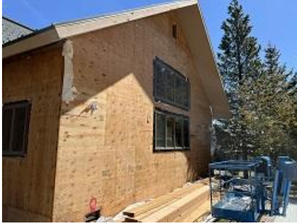
Building C3 Unit 32 Side Sheathing Exposed
