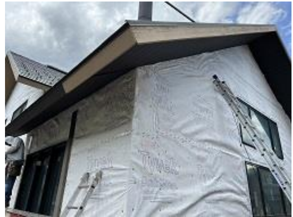
Building C8 Unit 66 Side & Back Soffit & Fascia Installed
