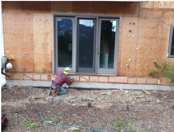
Building C7 Unit 59 Deck Ledger Blocking Installed
