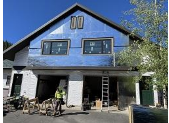
Building C8 Units 65 & 66 Front Insulation and Window Trim Installed
