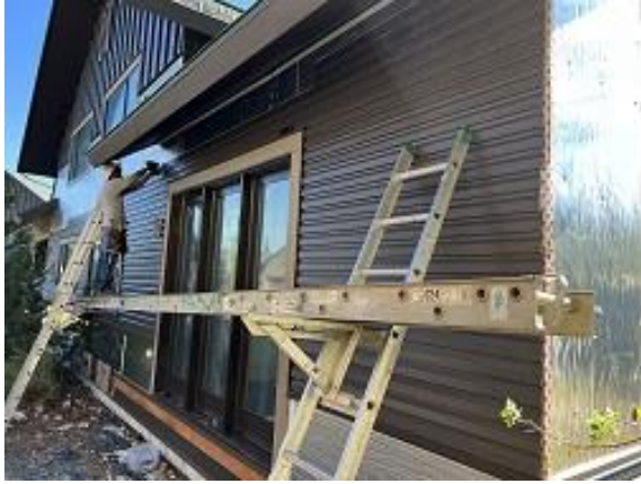
Building C5 Units 39 - 40 Lap Siding Installation Continued
