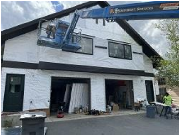
Building C8 Units 65 & 66 Front Snap Batten Flashing Installation Began
