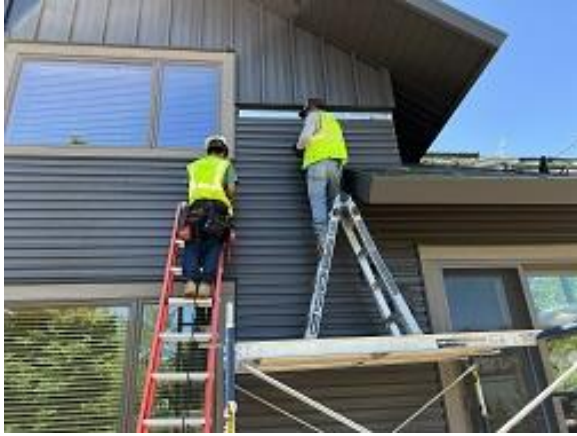
Building E3 Unit 24 Lap Siding Wire Penetration Repair
