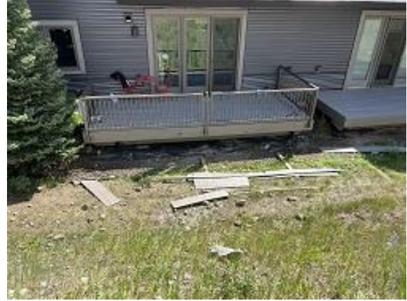
Building E4 Unit 29 Decking Reinstalled
