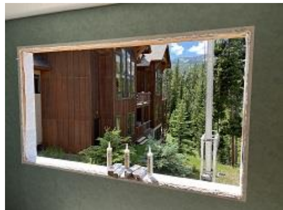
Building C7 Unit 59 Back Upper Window Removed
