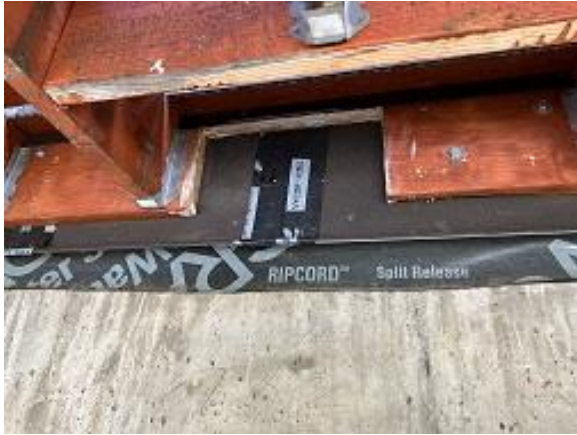
Building E7 Unit 52 Deck Ledger Flashing & Additional Flashing Tape Installed
