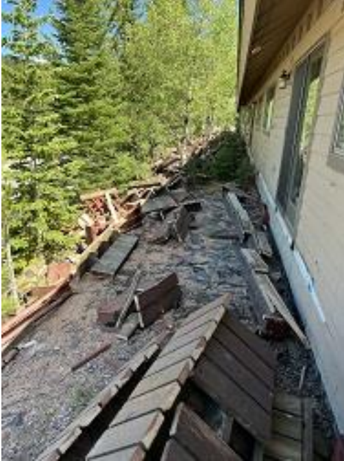
Building B Units 3 - 7 Deck Demolition
