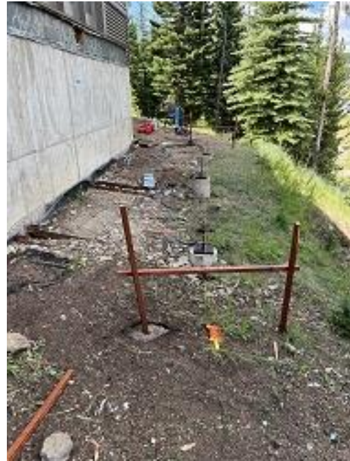
Building E7 Unit 52 Deck Post Knife Plates Installed
