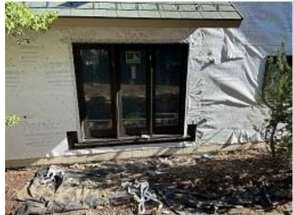
Building C2 Unit 15 Deck Door Installed
