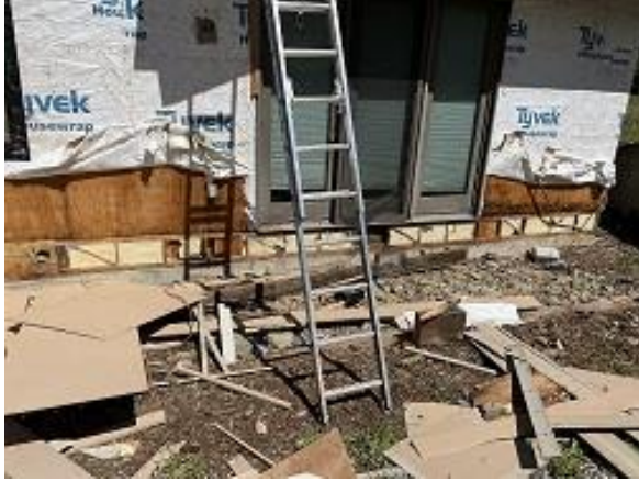
Building C9 Unit 68 Deck Ledger Sheathing Removed & Blocking Installed
