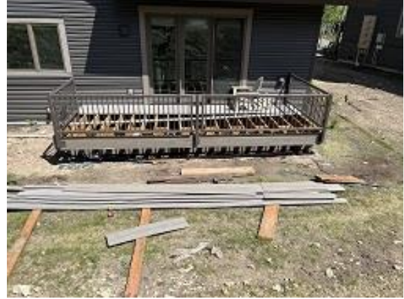
Building E2 Unit 23 Deck Railing Installed
