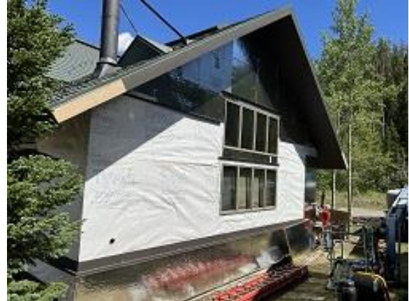
Building C1 Unit 13 Side Snap Batten Flashing and Insulation Installed
