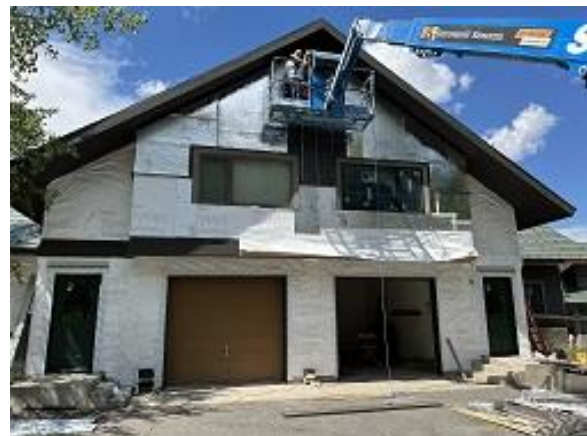
Building C1 Units 12 & 13 Front Snap Batten Siding Installed
