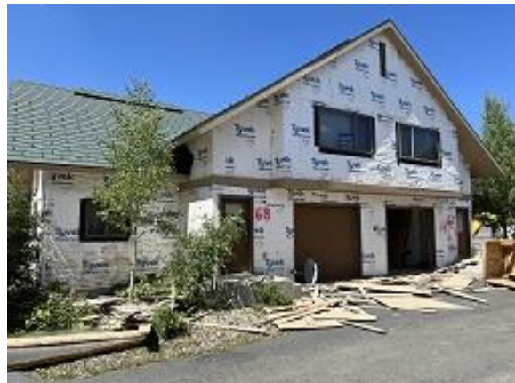
Building C9 Units 67 & 68 Front Siding Demolition
