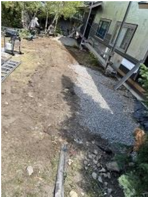
Building C1 Units 12 & 13 Deck Footings Infilled
