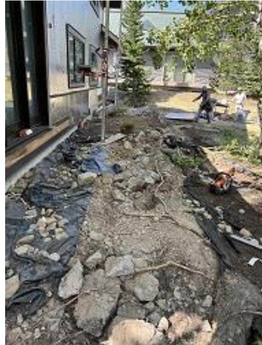
Building C1 Units 12 & 13 Deck Footing Demolition
