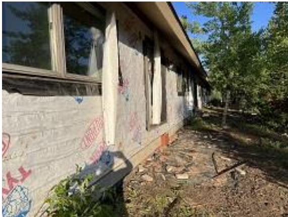
Building B Units 3-7 Back Siding Demolition
