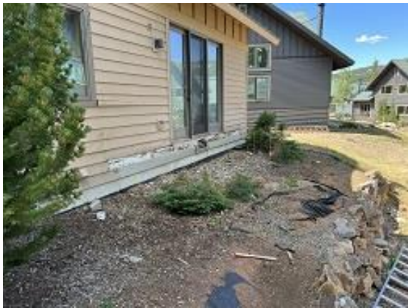
Building C10 Unit 69 Deck Demolition
