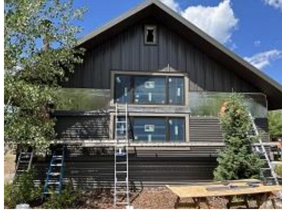
Building C5 Unit 39 Side Lap Siding Installed
