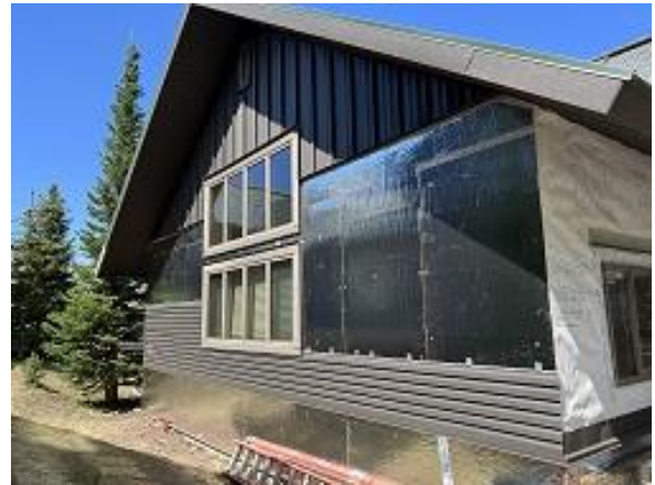
Building C1 Unit 13 Side Lap Siding Installed
