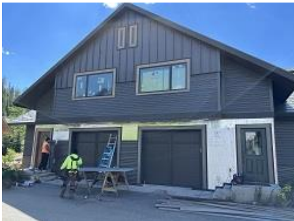
Building C5 Units 39 & 40 Front Corrugated Siding Installation Continued
