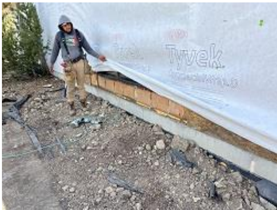
Building C3 Unit 33 Deck Ledger Blocking Installed
