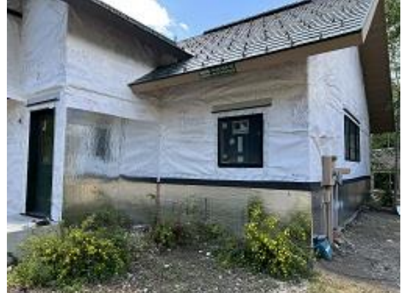
Building C1 Unit 12 Front & Side Insulation Installed
