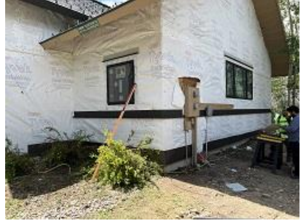
Building C1 Unit 12 Front & Side Base, Wainscot & Head Flashing Installed
