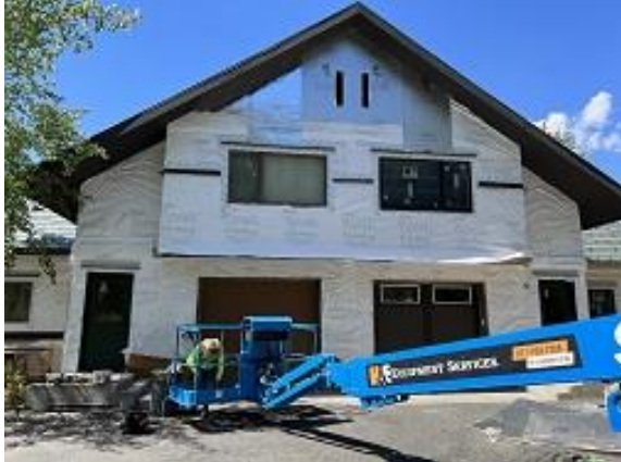
Building C1 Units 12 & 13 Front Snap Batten & Head Flashing and Insulation Installed
