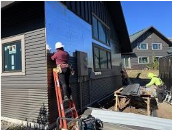
Building C5 Unit 40 Side Lap Siding Installed
