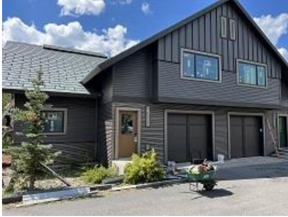
Building C5 Units 39 & 40 Front Corrugated Siding & Corners Installed
