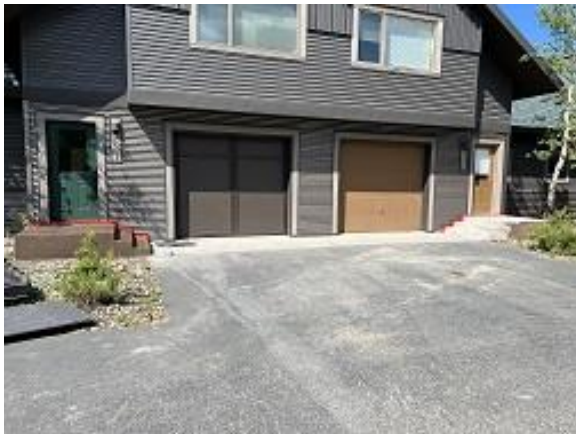
Building E4 Units 31 & 32 Stoop Refinishing
