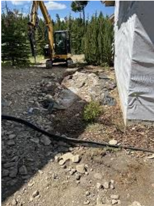
Building C7 Units 59 & 60 Deck Footing Demolition
