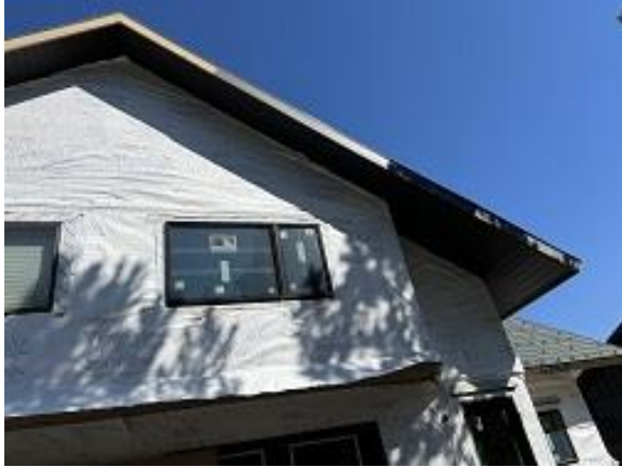
Building C1 Unit 12 Front Soffit & Fascia Installed
