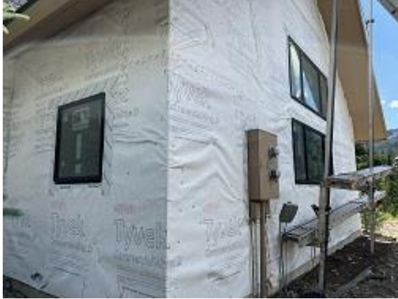
Building C7 Unit 59 Kitchen & Side Windows Installed
