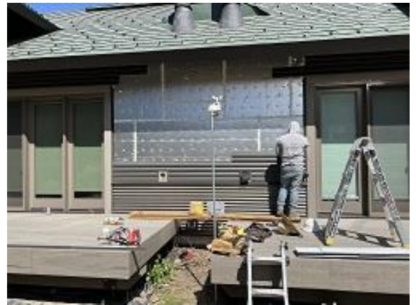
Building E2 Units 21 & 22 Back Fireplace Vent Located and Lap Siding Replaced
