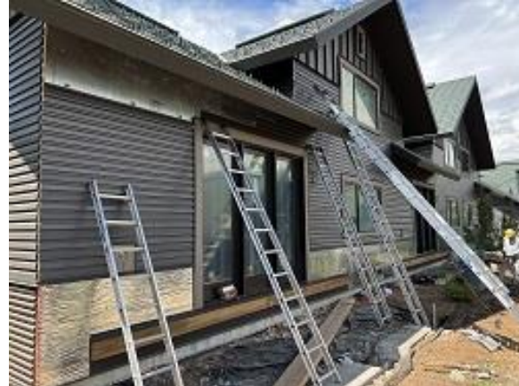
Building D Units 36 & 37 Lap Siding Installed
