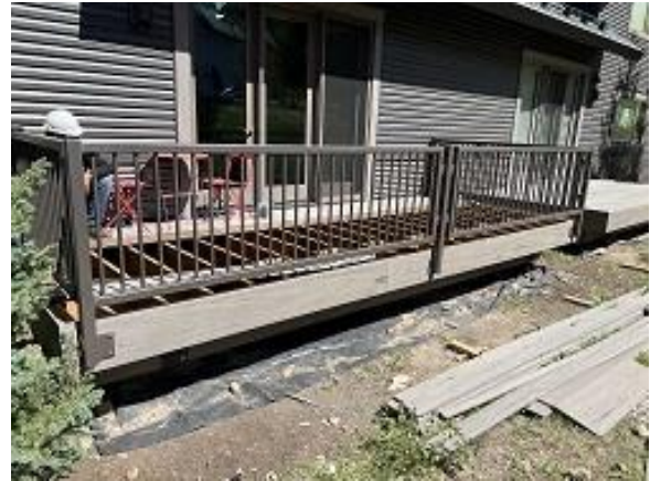
Building E4 Units 29 Deck Railing Installed
