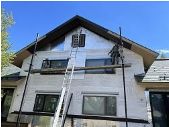
Building C1 Units 12 & 13 Back Soffit, Fascia and Insulation Installed
