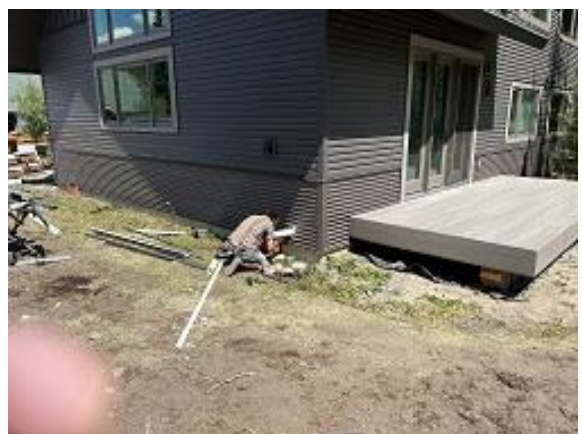
Building E1 Unit 11 Side Radon Exhaust Siding Penetration
