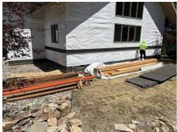
Building C3 Unit 32 Front & Side Wainscot & Base Flashing Installed
