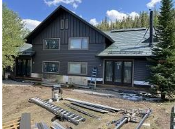
Building C1 Units 12 & 13 Back Lap Siding Installed
