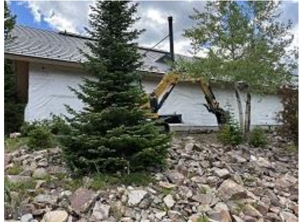
Building B Unit 3 Deck Footing Removal
