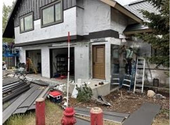
Building C2 Units 14 & 15 Front Insulation Board Installed
