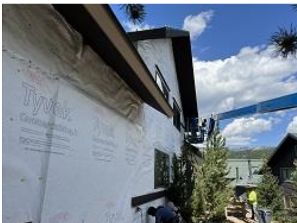
Building C3 Units 32 & 33 Back Soffit, Fascia, Wainscot & Head Flashing Installed
