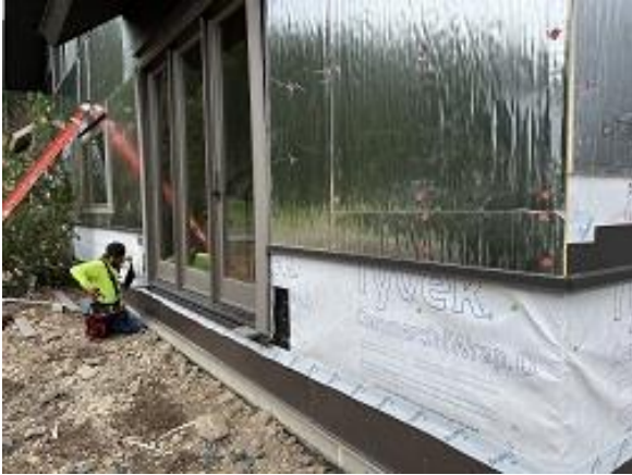
Building C3 Unit 33 Deck Door Trim Installed
