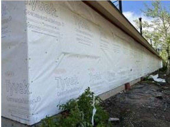
Building B Units 3 -7 Back Tyvek Installed
