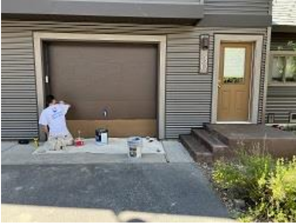
Building E4 Unit 30 Garage Door Painted
