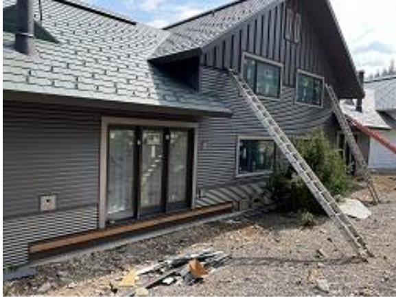
Building C8 Unit 65 Back Lap Siding Installed
