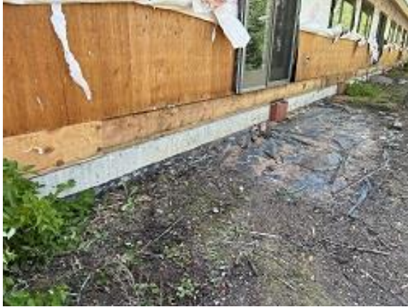
Building B Unit 3 Deck Ledger Sheathing Removed
