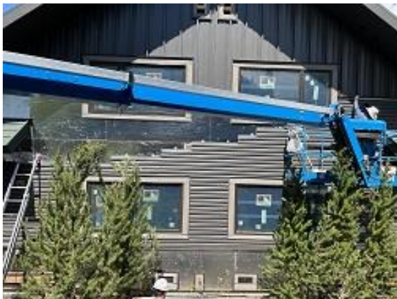
Building C2 Units 14 & 15 Back Lap Siding Installed
