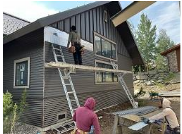
Building C8 Unit 65 Side Lap Siding Installed
