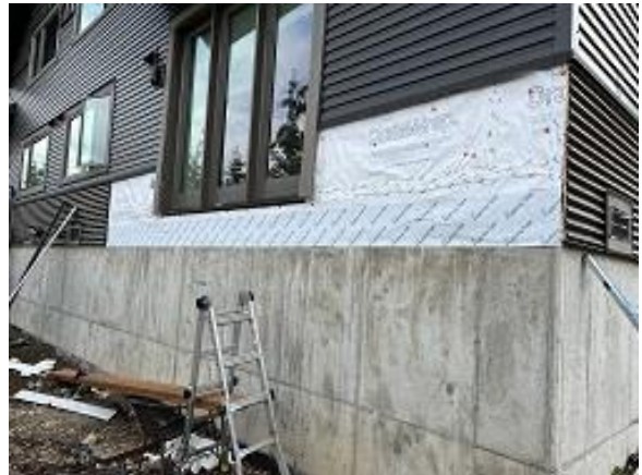
Building E7 Unit 52 Deck Ledger Tyvek and Flashing Tape Installed
