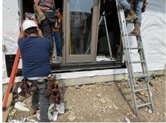
Building C3 Unit 33 Deck Door Removed & Reinstalled
