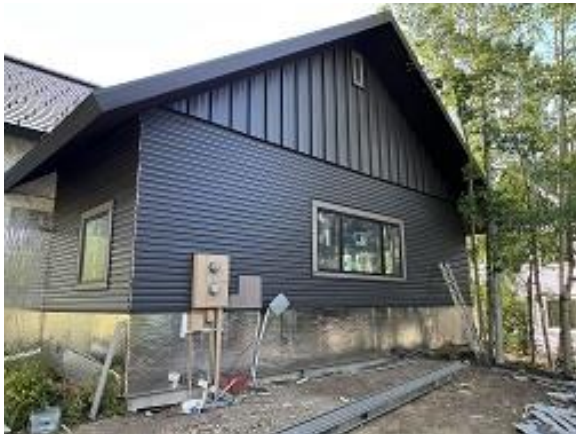
Building C1 Unit 12 Front & Side Lap Siding Installed
