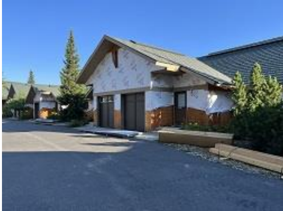
Building B Units 3 - 7 Siding Demolished
