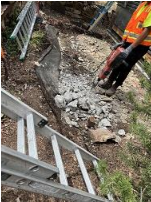
Building C2 Unit 15 Back Deck Footing Removed
