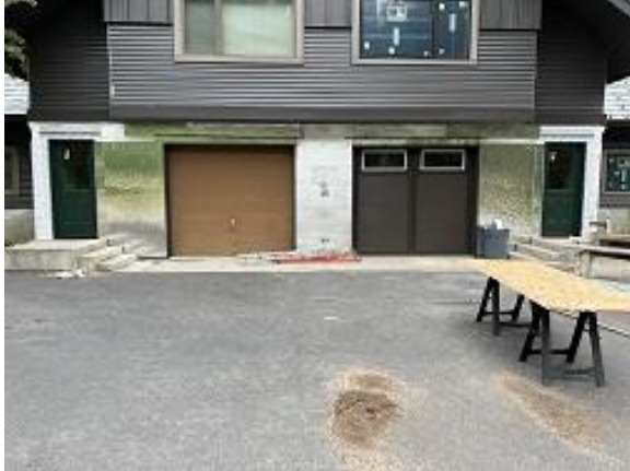
Building C1 Units 12 & 13 Front Base Flashing & Insulation Board Installed
