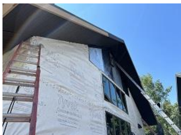
Building C3 Unit 33 Side Soffit & Fascia Installed
