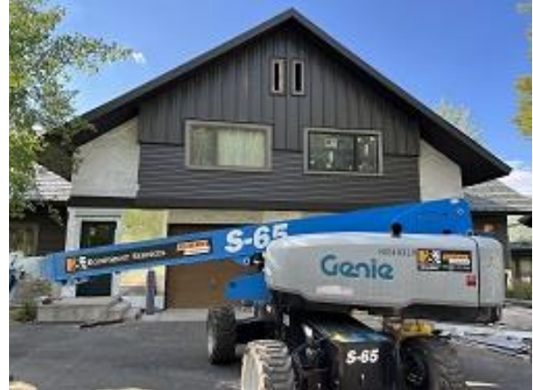
Building C1 Units 12 & 13 Front Lap Siding Installed
