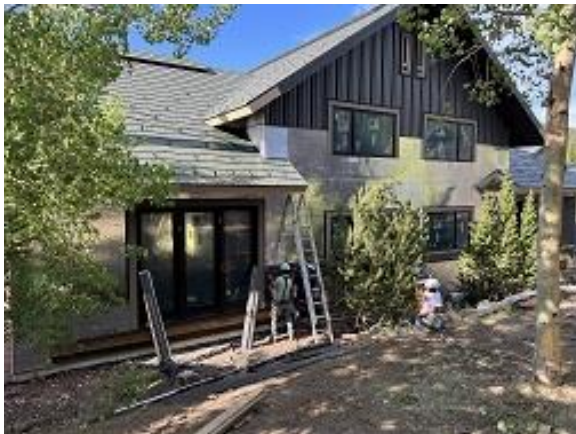
Building C2 Units 14 & 15 Back Lap Siding Installed
