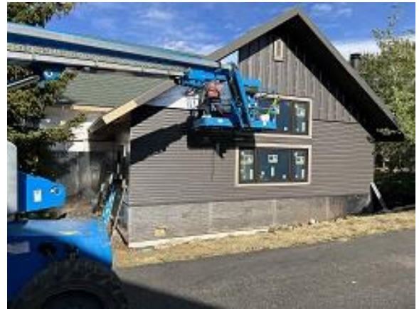
Building C2 Unit 15 Side Snap Batten Siding Installed
