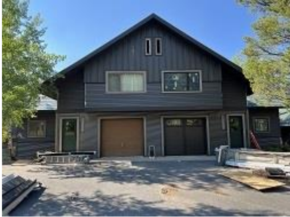
Building C1 Units 12 & 13 Front Corrugated Siding Installed
