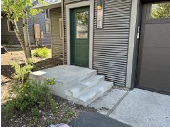
Building E2 Unit 23 Stoop Patched
