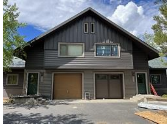
Building C1 Units 12 & 13 Front Corners Installed
