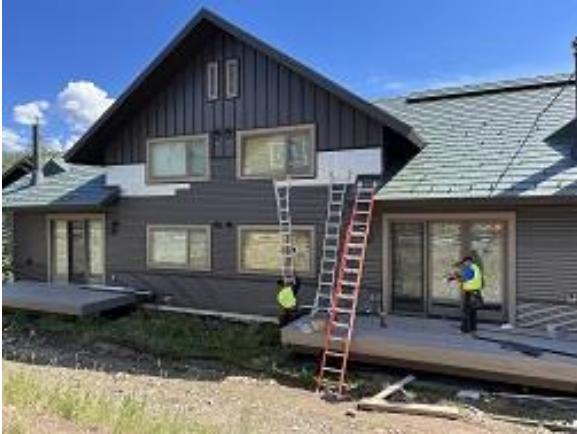
Building E2 Units 21 & 23 Back Lap Siding Repair
