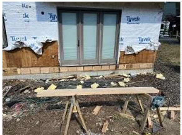
Building C4 Unit 34 Deck Ledger Blocking Installed
