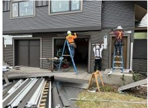
Building C2 Units 14 & 15 Front Corrugated Siding Installed
