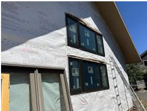
Building C7 Unit 60 Side Windows Installed
