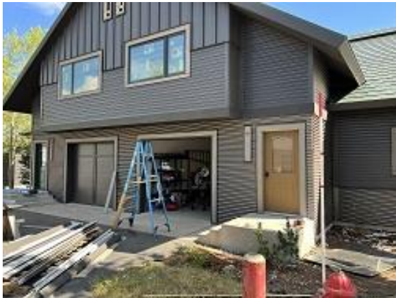
Building C2 Units 14 & 15 Front Corrugated Siding Installed
