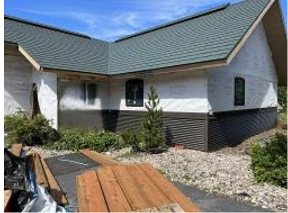
Building A Unit 1 Front & Side Corrugated Siding Installed
