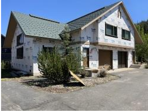
Building C10 Units 69 & 70 Front Siding Demolition Completed
