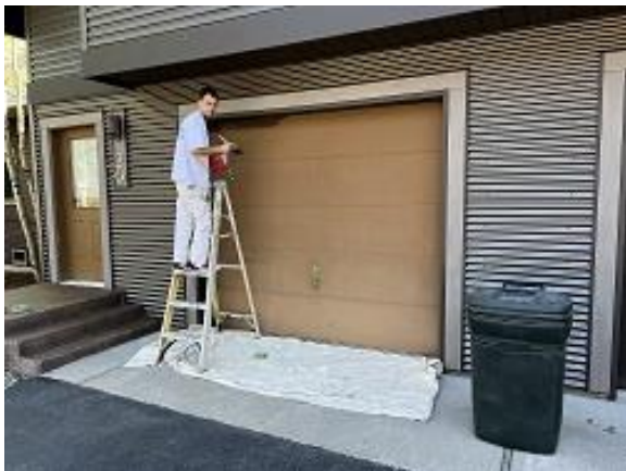
Building E3 Unit 26 Garage Door Painted
