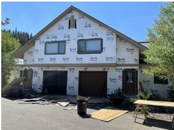
Building C4 Units 34 & 35 Front Siding Demolition Completed
