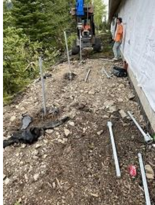
Building B Unit 7 Deck Helical Piers Installed
