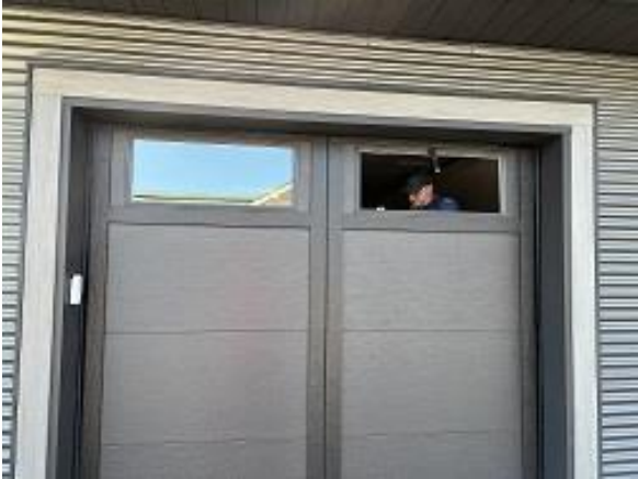
Building E1 Unit 8 Garage Door Window Sash Replacement
