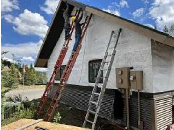
Building A Unit 2 Side Soffit & Fascia Installed
