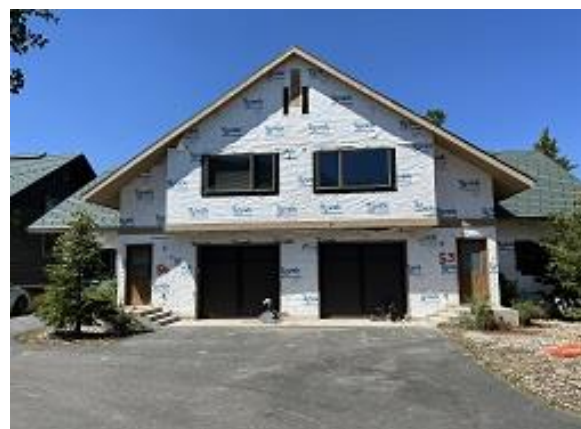
Building C6 Units 53 & 54 Front Siding Demolition Completed
