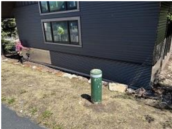
Building C2 Unit 15 Side Corrugated Siding Installed
