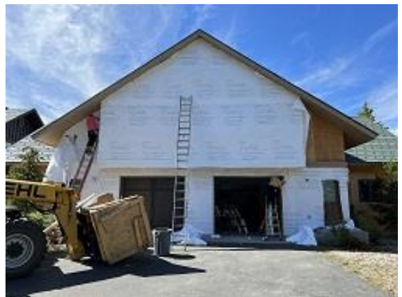
Building C6 Units 53 & 54 Front Tyvek Installed
