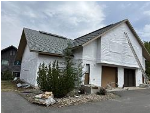
Building C10 Units 69 & 70 Front & Side Tyvek Installed
