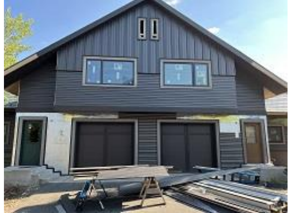
Building C2 Units 14 & 15 Front Corrugated Siding Installed
