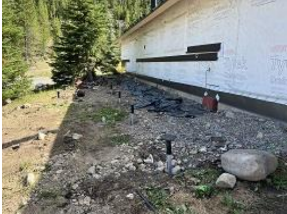
Building A Units 1 & 2 Deck Pier Beam Mounts Installed
