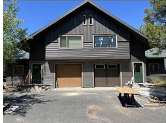
Building C1 Units 12 & 13 Front Corrugated Siding Installed
