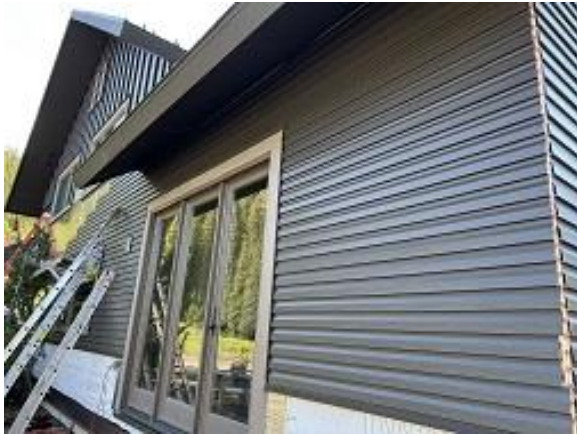
Building C3 Unit 33 Back Lap Siding Installed
