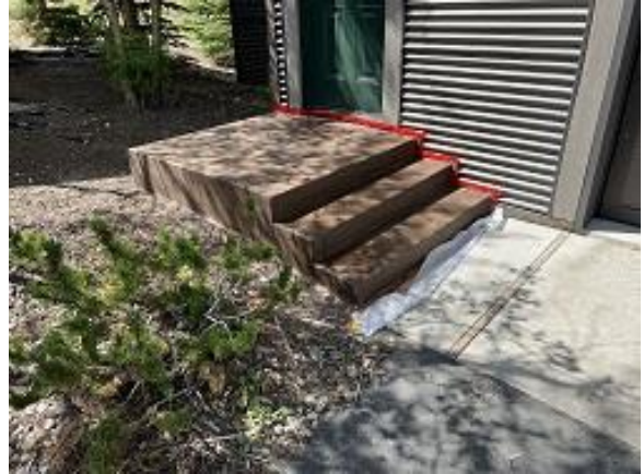
Building F2 Unit 19 Stoop Refinishing Began
