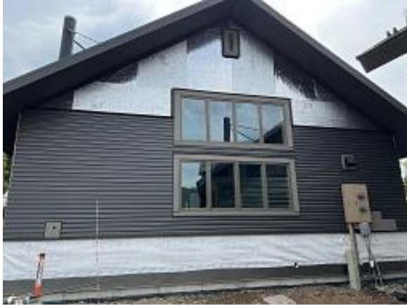
Building C3 Unit 33 Side Lap Siding Installed
