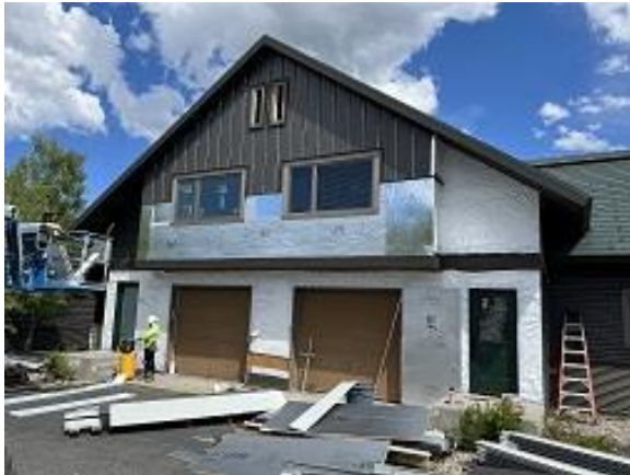
Building C3 Units 32 & 33 Front Snap Batten Siding Installed
