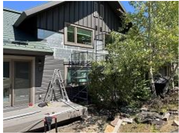
Building E1 Units 10 & 11 Back Lap Siding Repair
