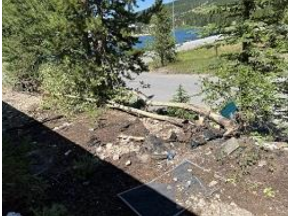
Building B Units 6 & 7 Deck Footing & Tree Removed
