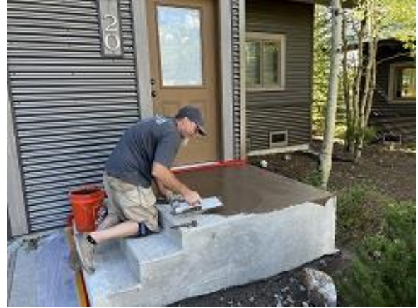
Building E2 Unit 20 Stoop Color Coat
