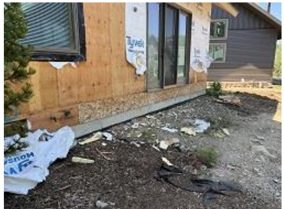
Building C10 Unit 69 Deck Ledger Sheathing Installed
