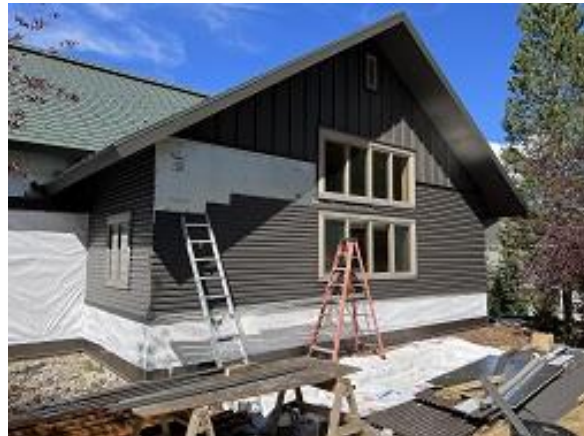
Building C3 Units 32 Side Lap Siding Installed
