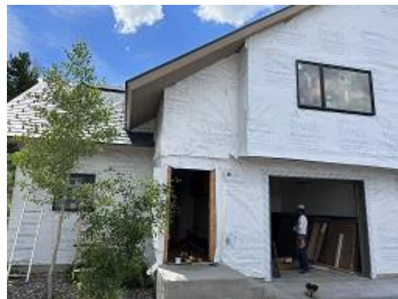
Building C9 Unit 68 Front Upper & Kitchen Windows Installed
