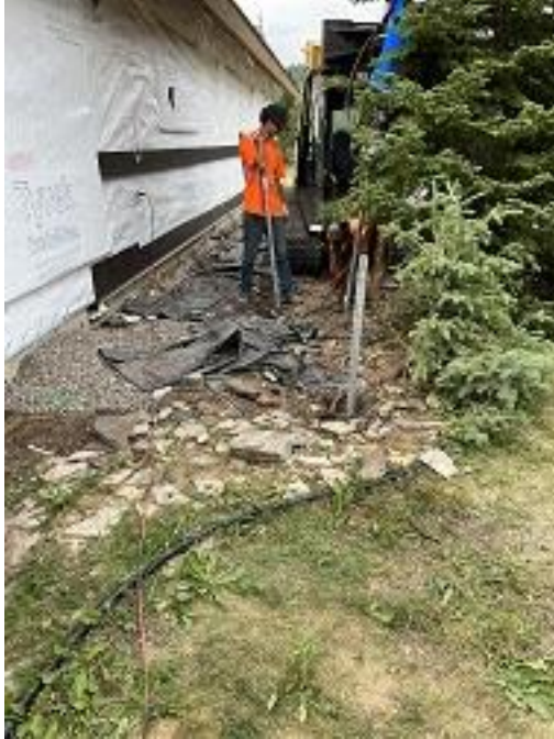
Building A Unit 1 Deck Helical Piers Installed
