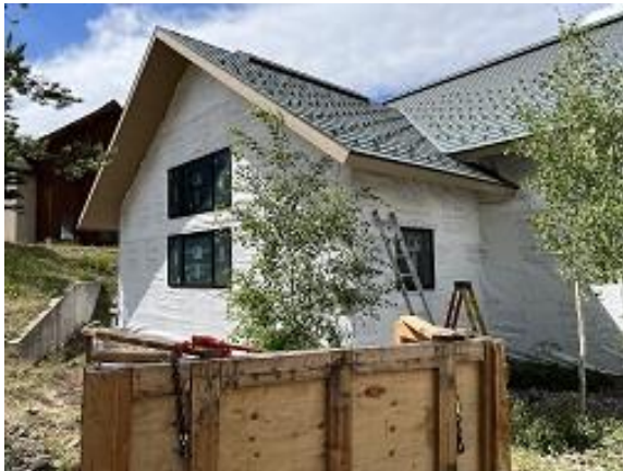
Building C9 Unit 68 Side & Kitchen Windows Installed
