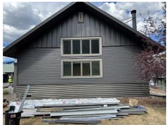
Building C3 Unit 32 Side Corrugated Siding Installed
