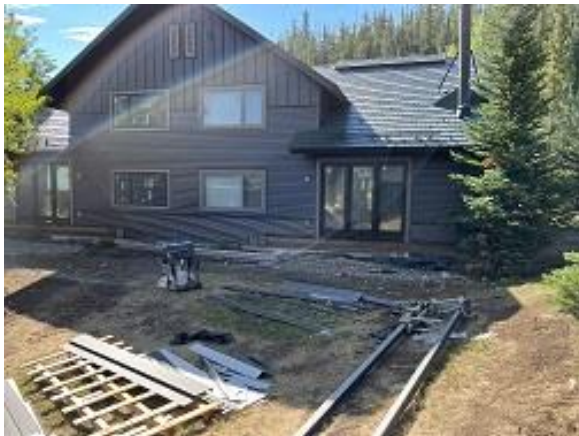
Building C1 Units 12 & 13 Back Corrugated Siding Installed
