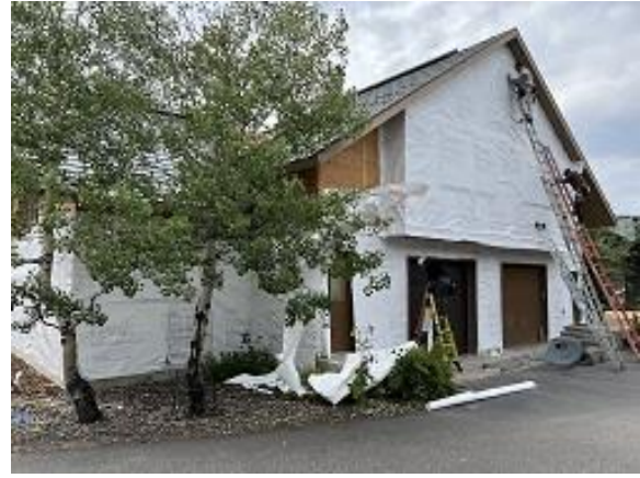
Building C4 Units 34 & 35 Front & Side Tyvek Installed
