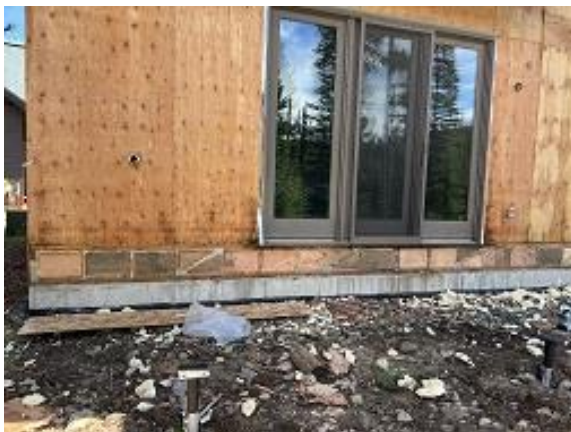
Building C6 Unit 53 Deck Ledger Sheathing Removed & Blocking Installed
