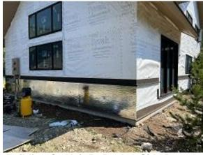
Building C7 Unit 59 Back & Side Base & Wainscot Flashing Installed
