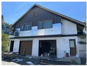
Building E9 Units 67 & 68 Front Foam Board Insulation and Snap Batten Siding Installed
