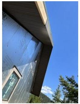
Building A Unit 1 Side Soffit, Fascia and Insulation Installed
