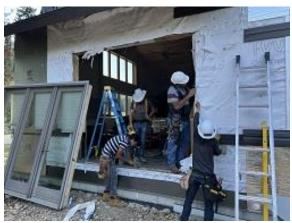
Building C3 Unit 32 Deck Door Remove, Flashed and Replaced
