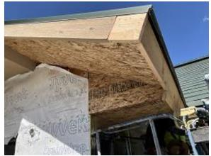
Building A Unit 1 Front Rafter Repair Fascia Installed
