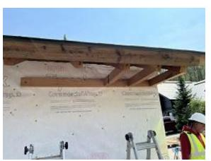
Building B Unit 5 Rafter Repair Soffit Cross Ties Installed
