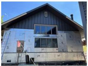
Building E9 Units 67 Side Foam Board Insulation and Snap Batten Siding Installed
