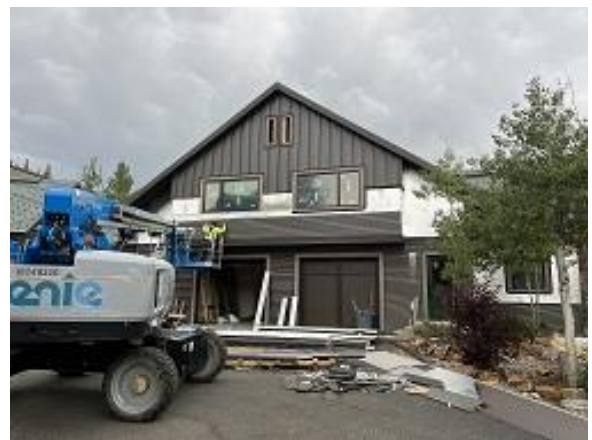
Building C7 Units 59 & 60 Front Lap Siding Installed
