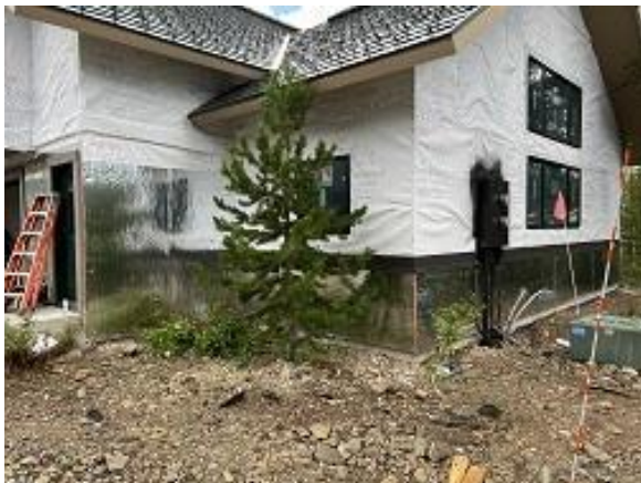
Building C6 Unit 53 Front & Side Insulation Board Installed
