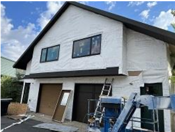
Building C10 Units 69 & 70 Belly Band Flashing Installed
