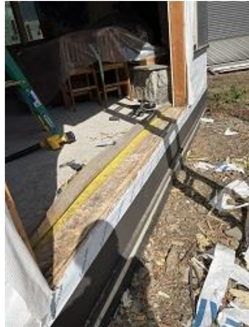
Building C10 Unit 69 Deck Door Removed
