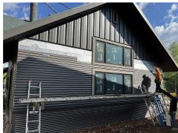
Building C7 Unit 60 Side Lap Siding Installed
