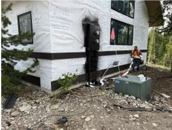
Building C6 Unit 53 Front & Side Base & Wainscot Flashing Installed
