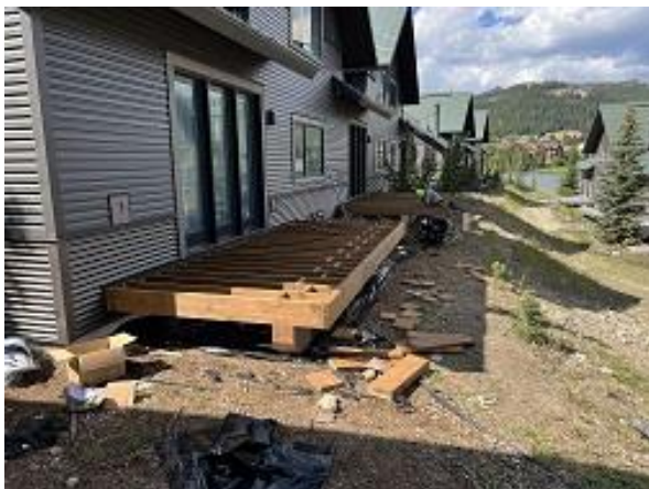
Building D Units 36 - 38 Deck Framing Began
