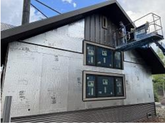
Building C7 Unit 60 Side Snap Batten Siding Installed
