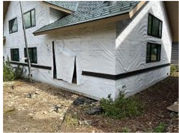
Building C6 Unit 54 Back & Side Base & Wainscot Flashing Installed
