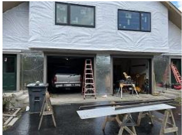
Building C6 Units 53 & 54 Front Insulation Board & Door Trim Installed
