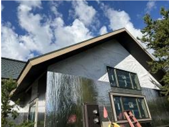
Building C6 Unit 53 Front & Back Soffit Installed
