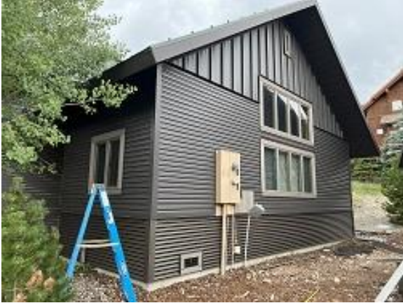
Building C9 Unit 67 Side Corrugated Siding Installed
