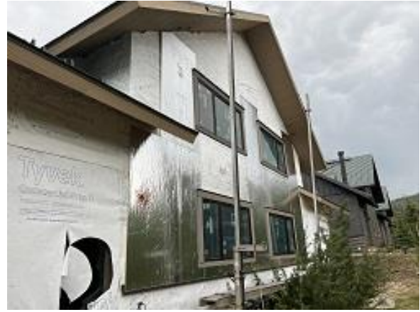
Building C6 Units 53 & 54 Back Insulation Board & Window Trim Installed
