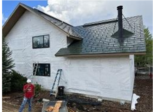
Building C4 Unit 34 Back Windows Installed
