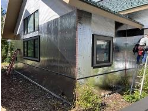
Building C6 Unit 54 Window Trim & J Channel Installed
