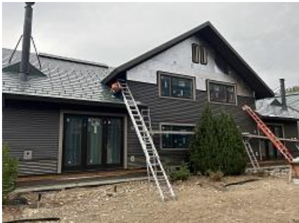
Building C7 Units 59 & 60 Back Lap Siding Installed
