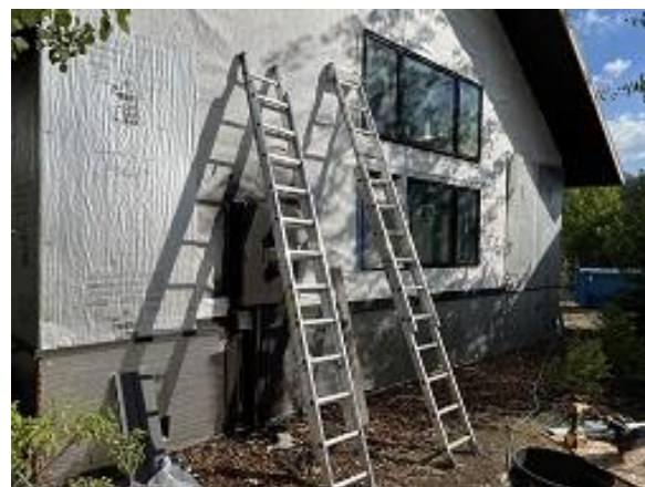
Building C10 Unit 70 Insulation Board Installed
