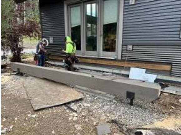
Building C3 Unit 32 Deck Beam Installed
