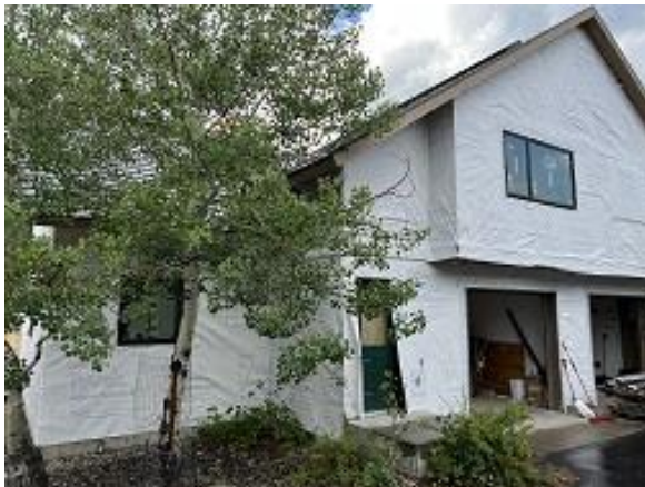
Building C4 Unit 34 Front Windows Installed
