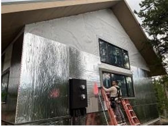
Building C6 Unit 53 Side Insulation Board & Window Trim Installed
