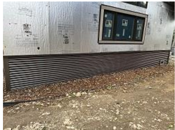
Building C7 Unit 60 Side Corrugated Siding Installed
