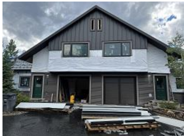
Building C7 Unit 59 & 60 Front Snap Batten Siding Installed
