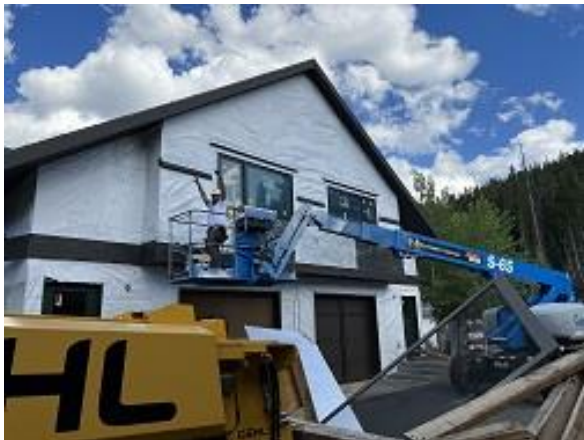
Building C10 Units 69 & 70 Snap Batten Flashing Installed
