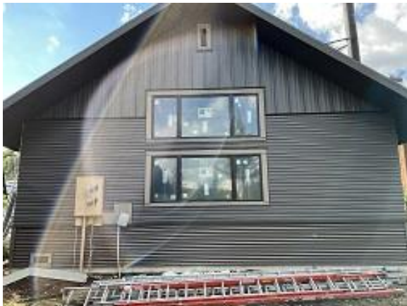
Building C7 Unit 59 Side Lap Siding Installed
