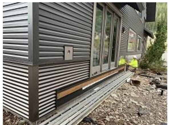
Building C9 Units 67 & 68 Back Corrugated Siding Installed
