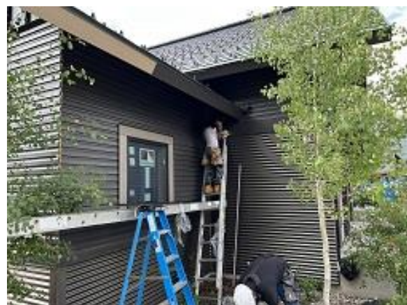
Building C9 Unit 68 Front Lap Siding Installed
