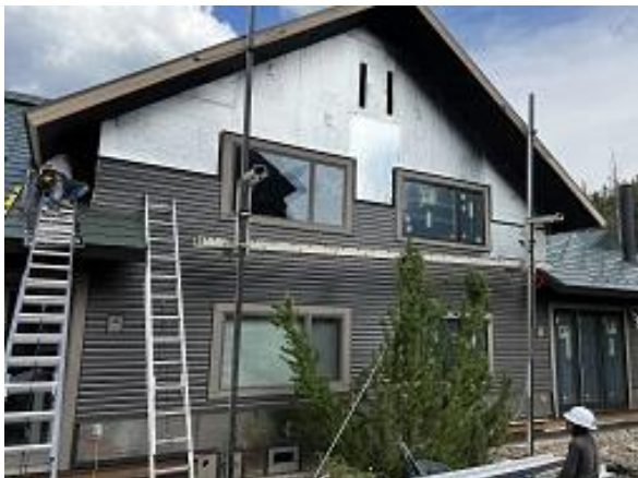
Building C9 Units 67 & 68 Back Lap Siding Installed
