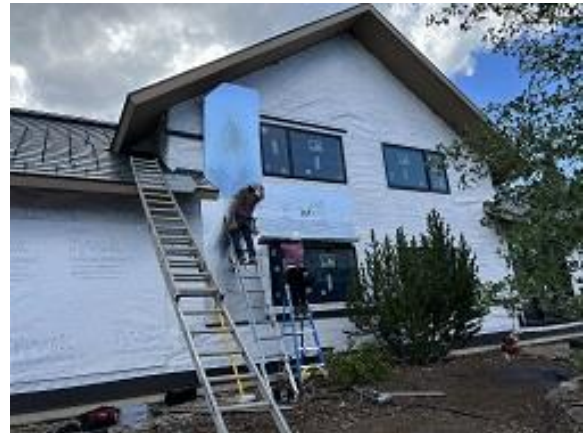
Building C10 Units 69 & 70 Insulation Board Installed
