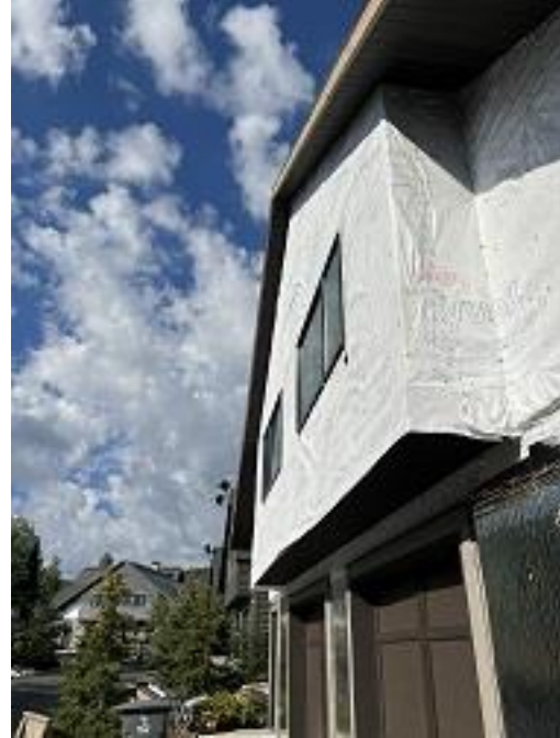
Building C6 Units 53 & 54 Front Soffit Installed
