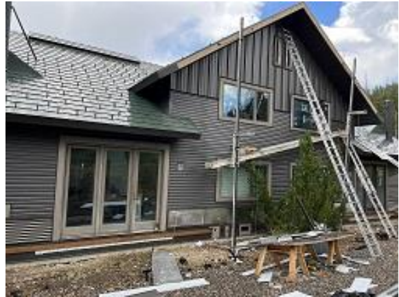
Building C9 Units 67 & 68 Back Lap Siding Installed
