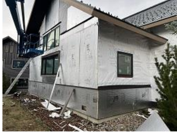
Building C10 Unit 69 Side Base & Wainscot Flashing and Insulation Board Installed
